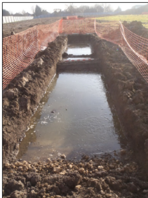
Plate 6: Trench 7, Looking South
