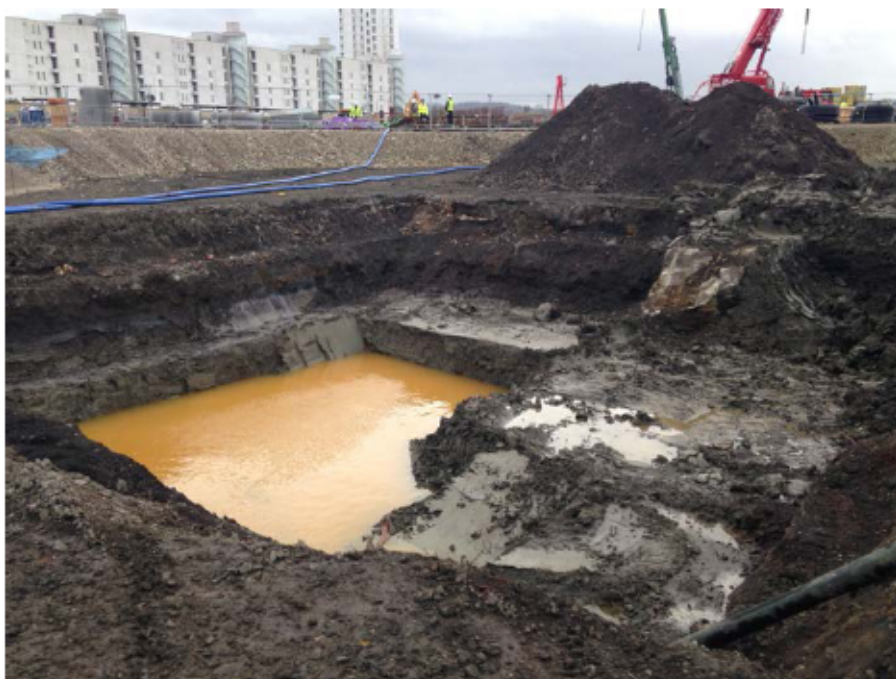
Plate 1: Tr1 under excavation, looking SE
