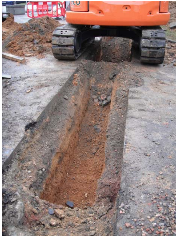
Plate 2: Excavation of DR1, Looking SSW
