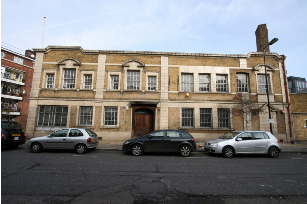
Plate 35: Webber Street (south) elevation of nos 17-19 Valentine Place/no. 21 Webber Street, looking north (VAL14 D100 (12))
