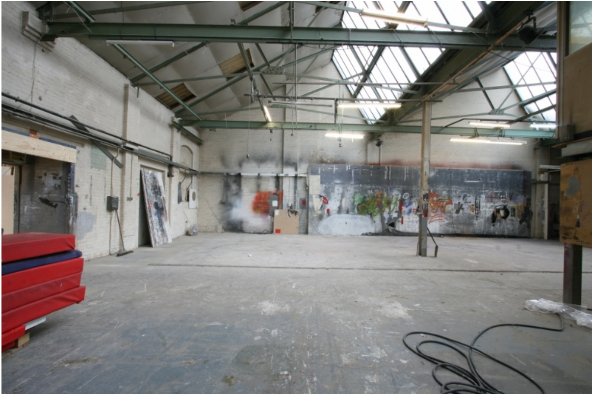
Plate 16: South walls of room B1G1 in nos 3-5 Valentine Place with saw-tooth roof, looking south (VAL14 D100 (130))
