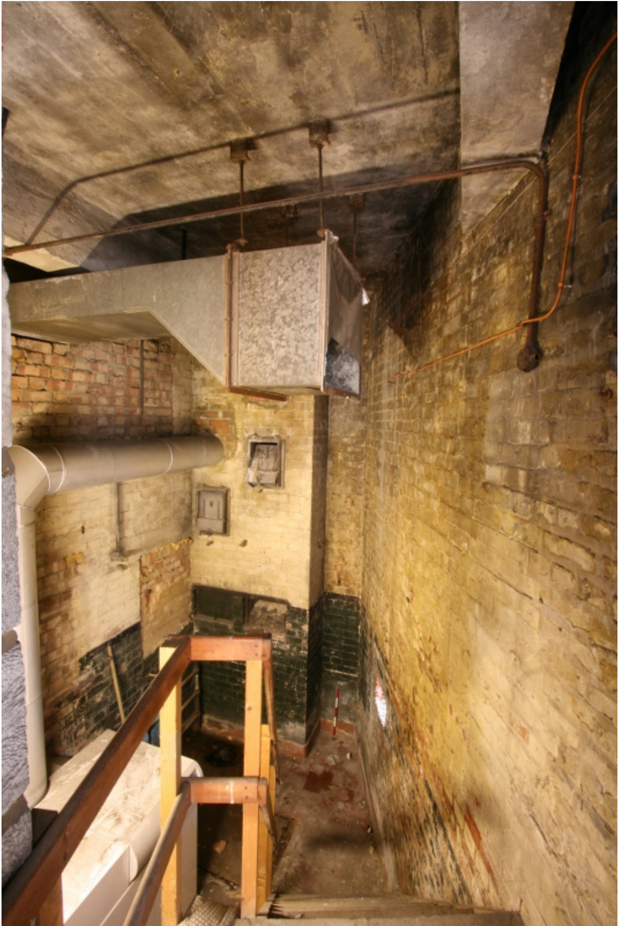
Plate 66: Basement/ground floor room B2B6/B2G20, looking east (VAL14 D100 (50))
