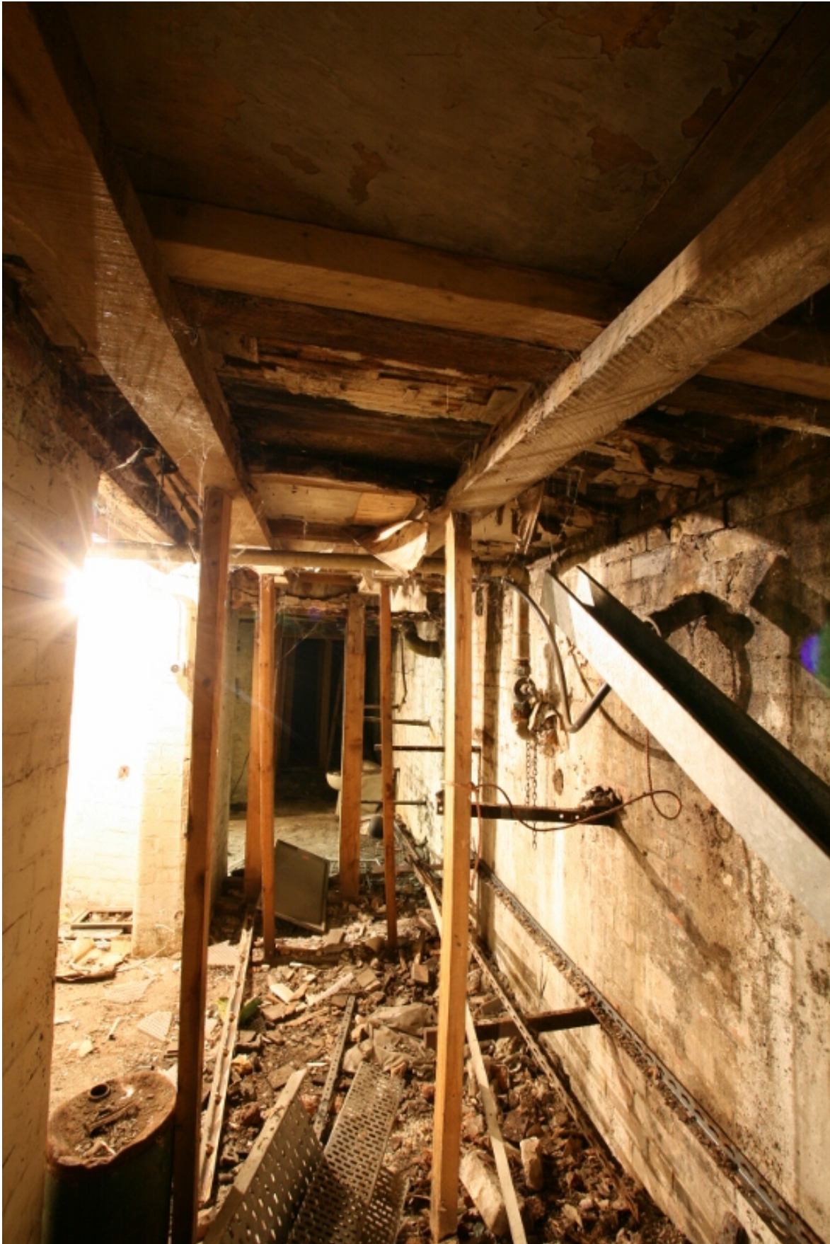
Plate 51: Pavement vault area of basement, looking west (VAL14 D100 (61))
