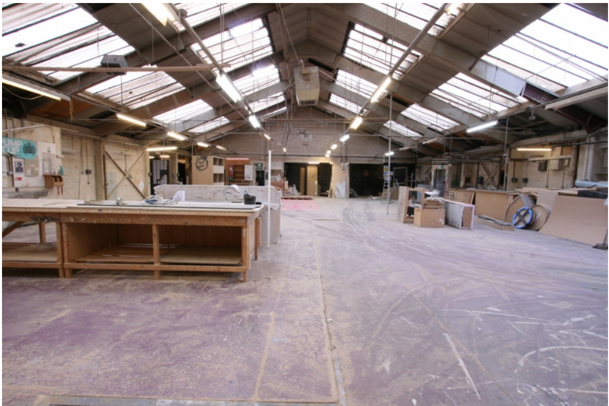
Plate 22: Main work area in room B1G3, looking south (VAL14 D100 (63))
