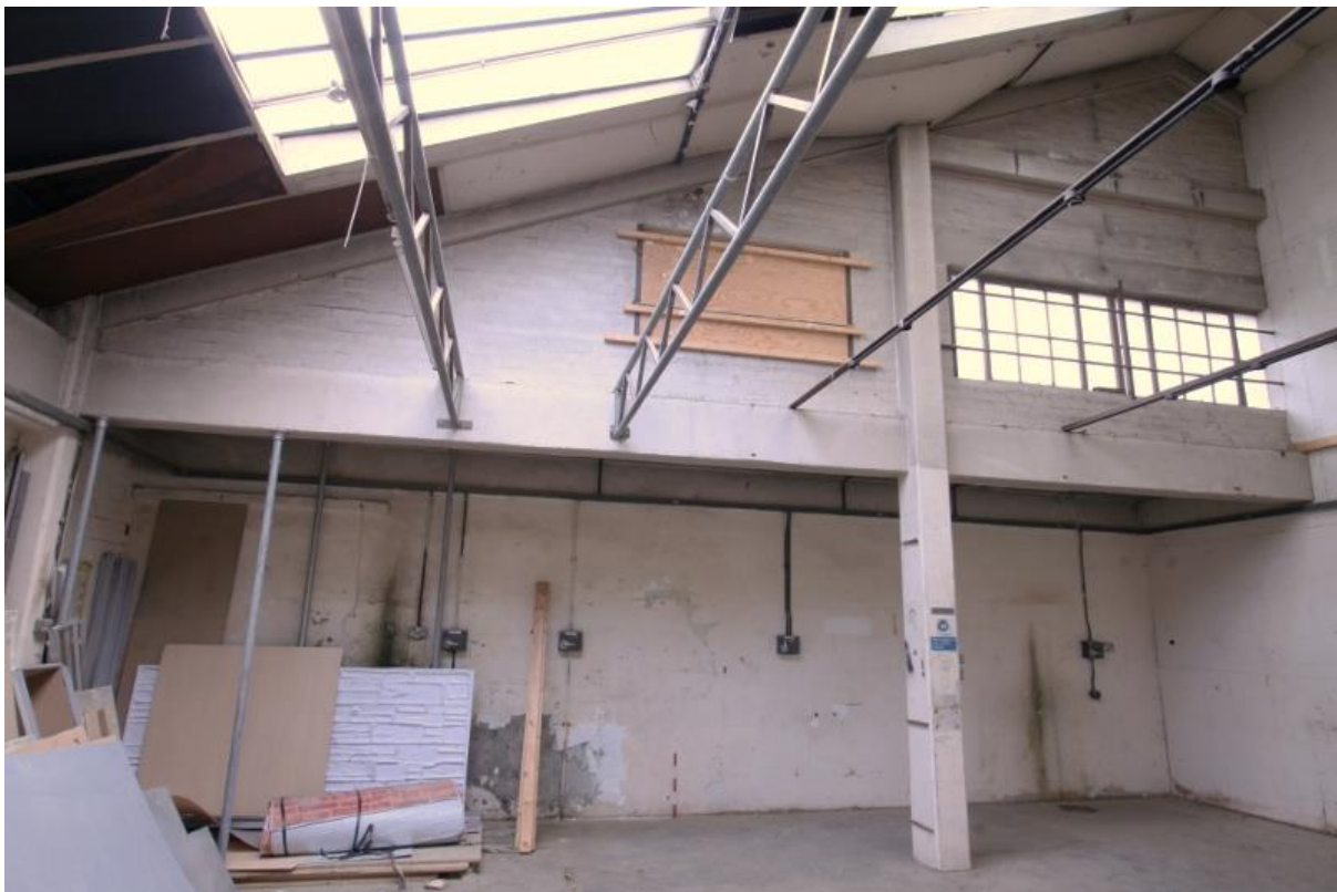
Plate 28: Room B1G4, looking north (VAL14 D100 (72))
