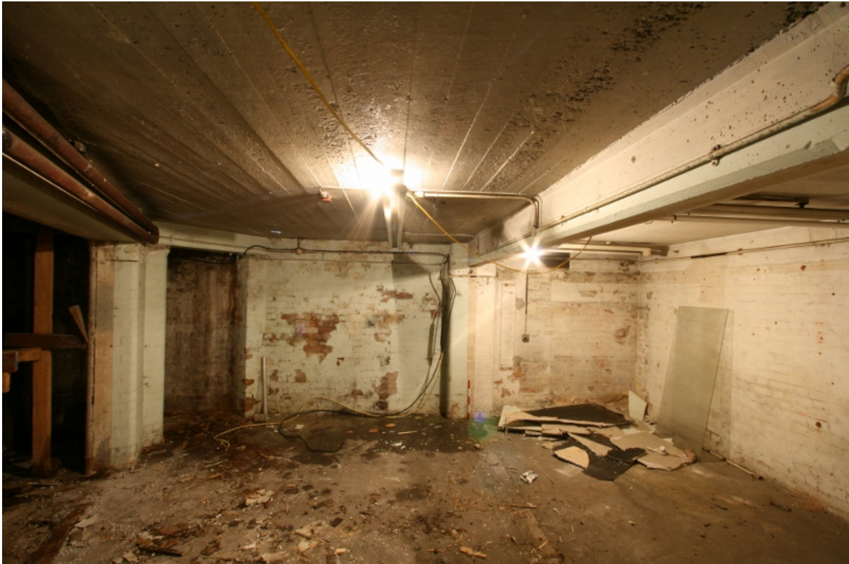
Plate 49: Basement room B2B3, looking west (VAL14 D100 (59))
