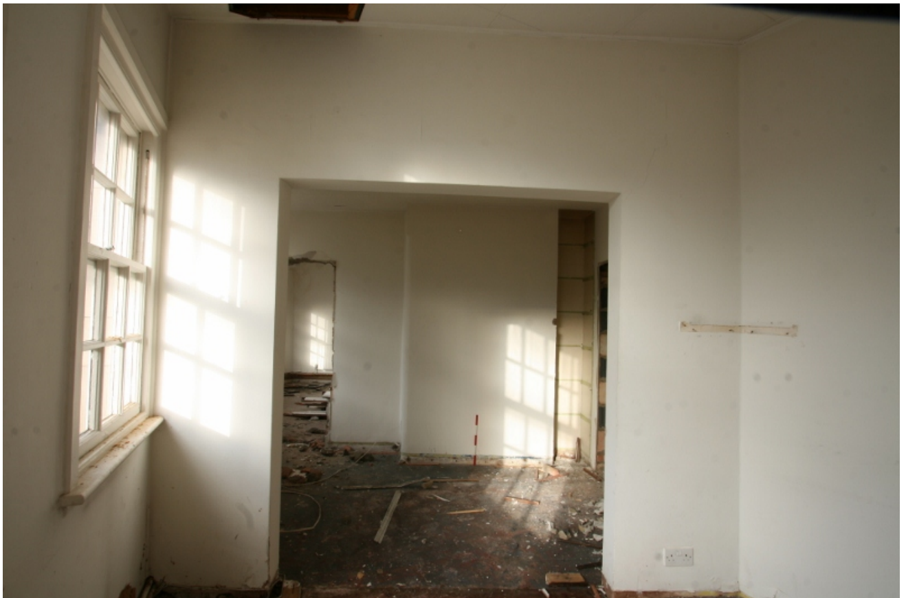
Plate 71: Chimney-breast in first floor room B2F5, looking west (VAL14 D100 (81))
