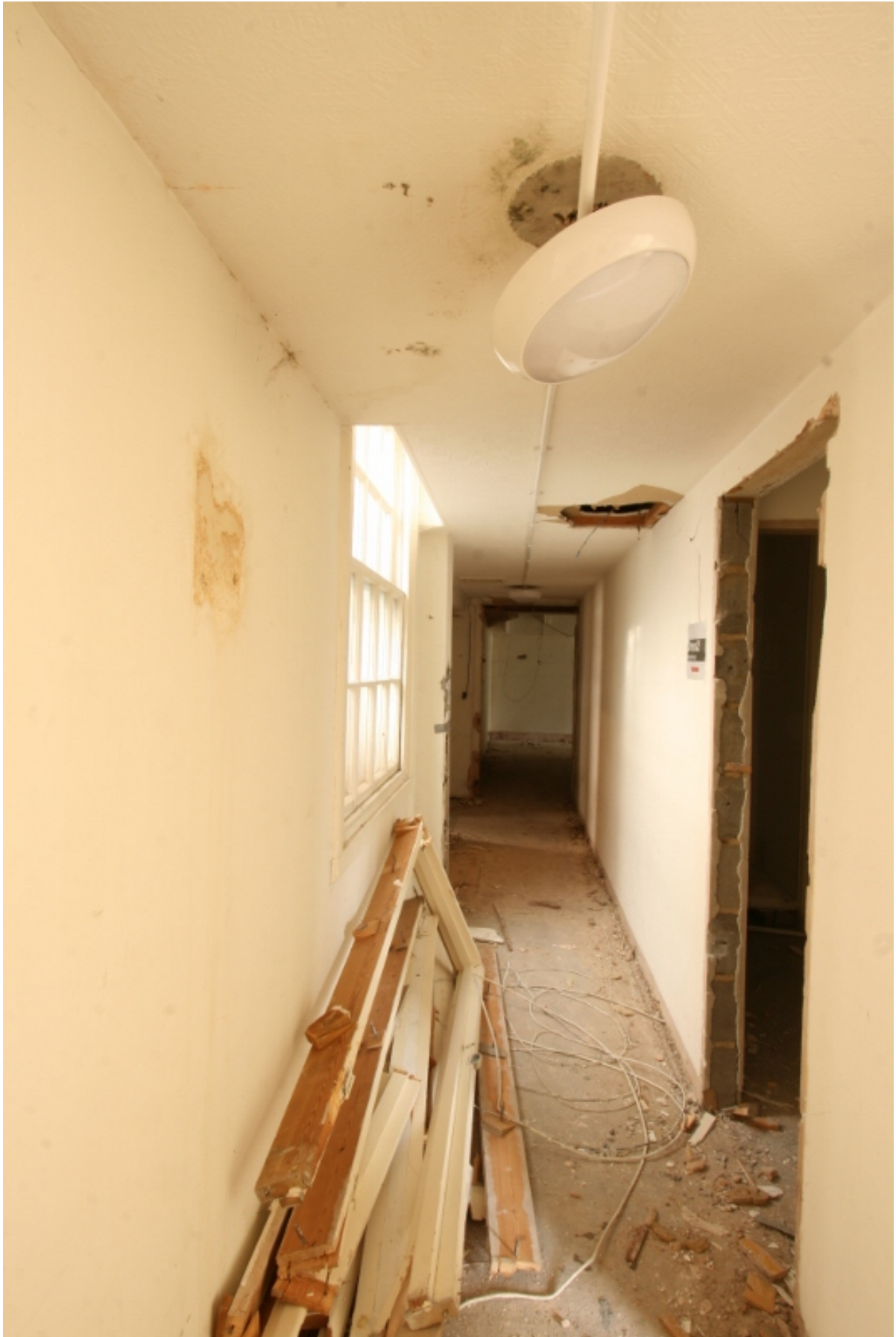
Plate 74: First floor corridor created by inserting modern partition breeze block wall, looking north (VAL14 D100 (91))
