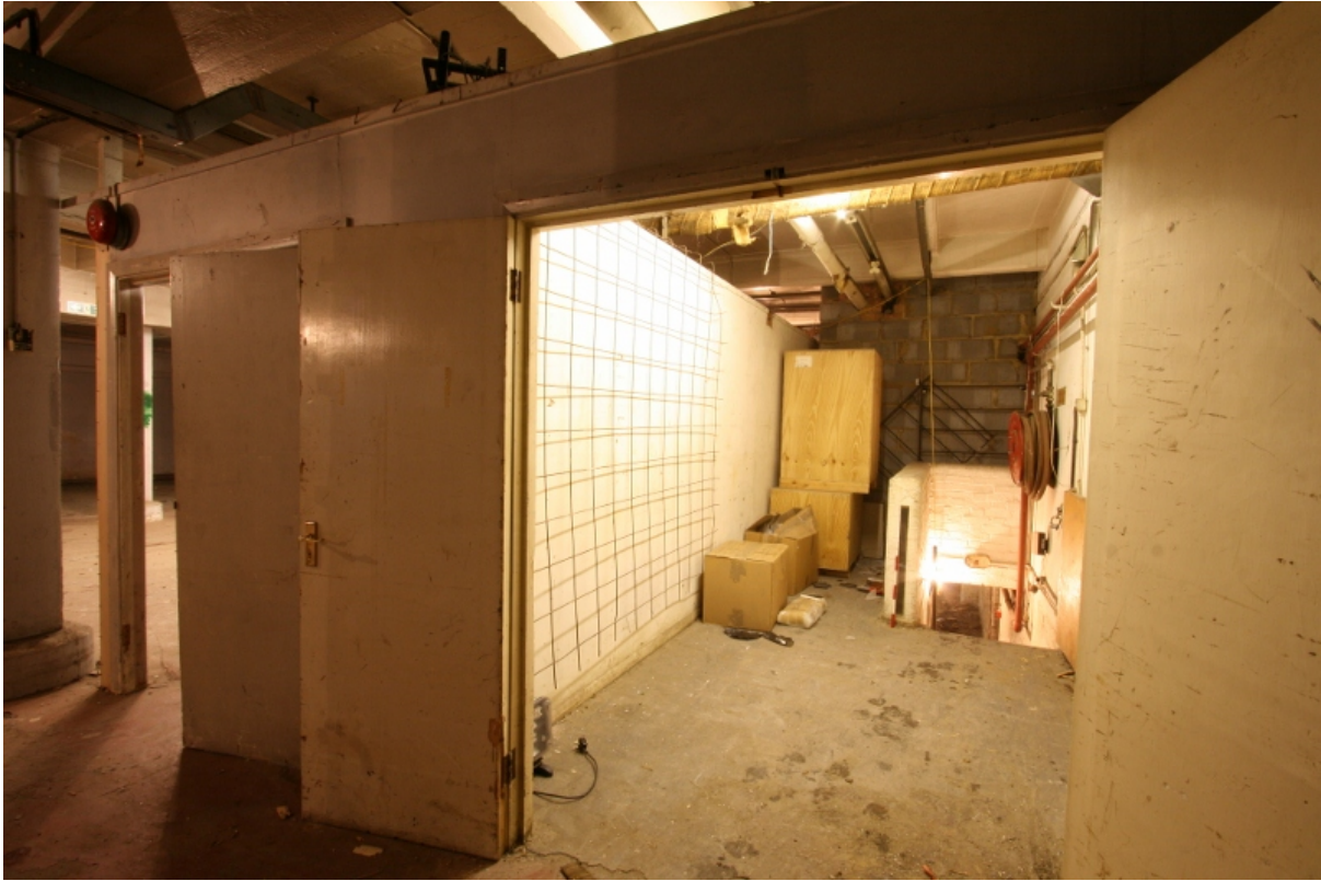
Plate 45: Entrance from ground floor room B2G3 to staircase down to the basement, looking south (VAL14 D100 (52))
