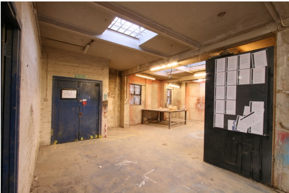
Plate 26:Rear work area in room B1G3, looking south-east (VAL14 D100 (68))
