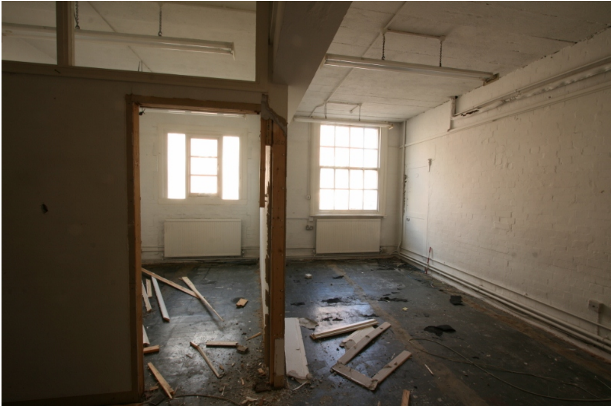
Plate 77: Inserted partitions in first floor room B2F2, looking south-west (VAL14 D100 (94))
