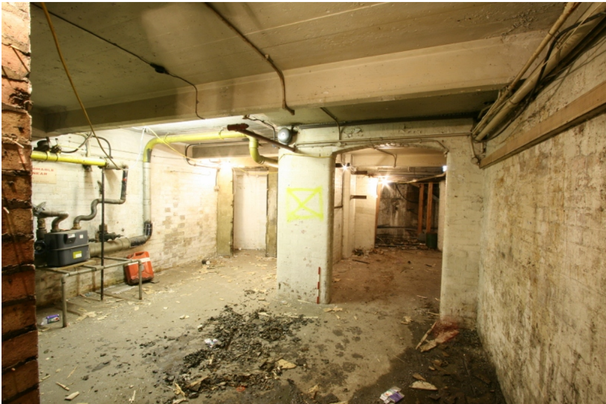
Plate 46: Basement room B2B1, looking south (VAL14 D100 (54))
