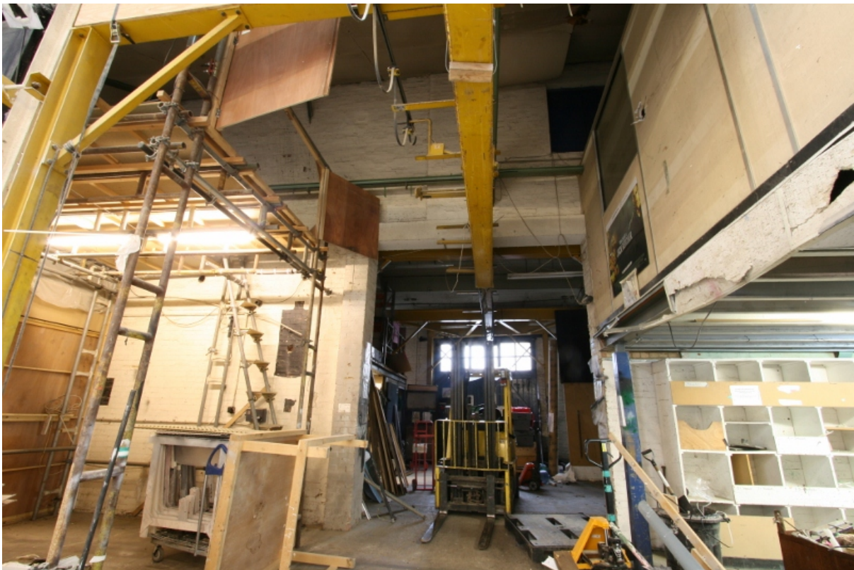
Plate 19: Room B1G1 with inserted mezzanine level (right), looking west (VAL14 D100 (132))
