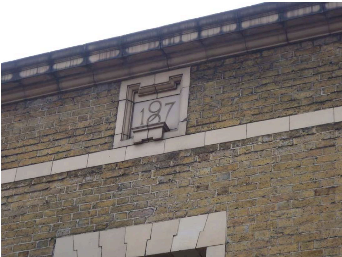
Plate 32b: Date plaque '1907' on the Valentine Place (west) elevation of nos 17-19 Valentine Place/no. 21 Webber Street, looking east (CAM P9110050.JPG)
