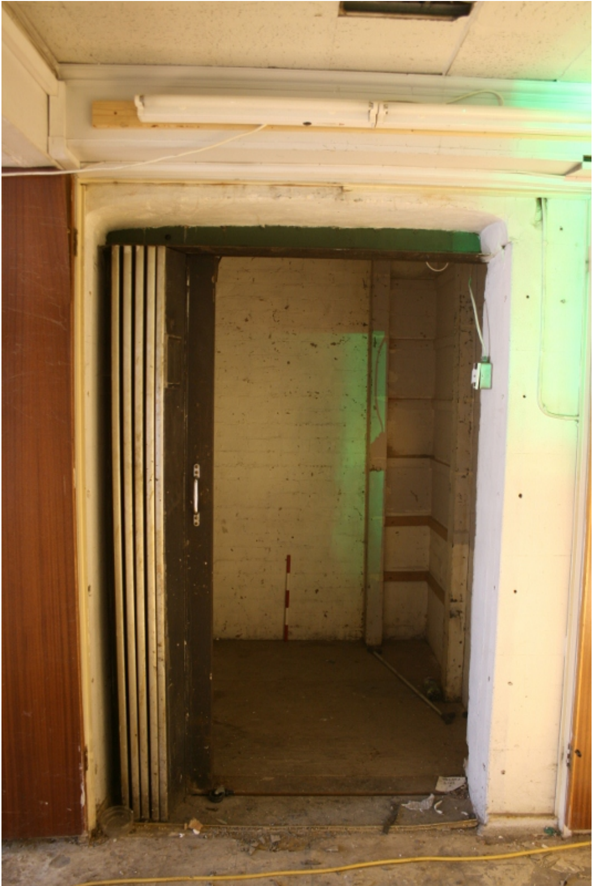
Plate 60: Converted lift shaft in corridor 3 at ground floor level, looking west (VAL14 D100 (40))
