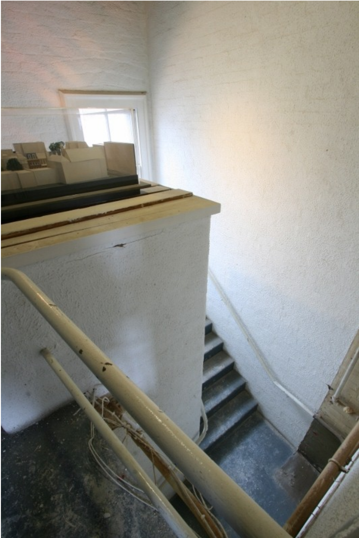
Plate 89: Stairwell 1, looking (VAL14 D100 (126))
