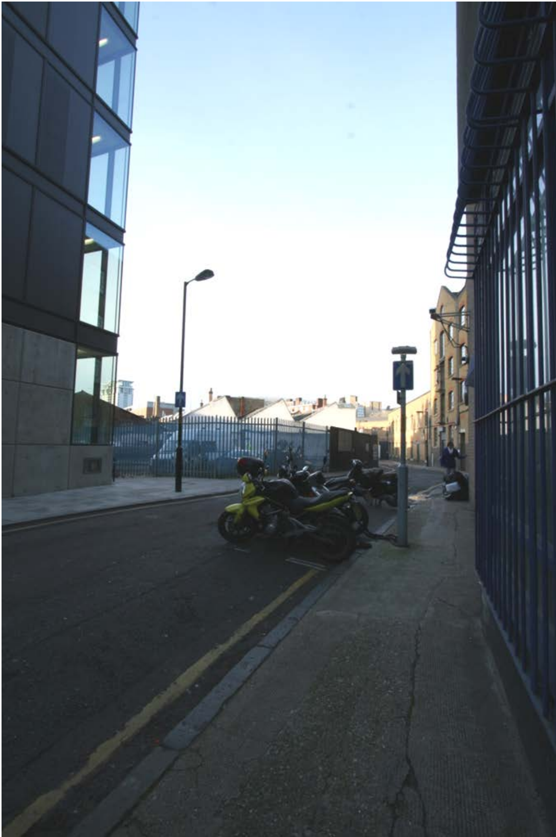
Plate 1: Distinctive saw-tooth roof of nos 3-5 Valentine Place, looking south (VAL14 D100 (1))
