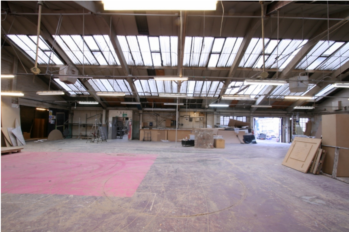
Plate 23: Two entrance in room B1G3, looking west (VAL14 D100 (65))
