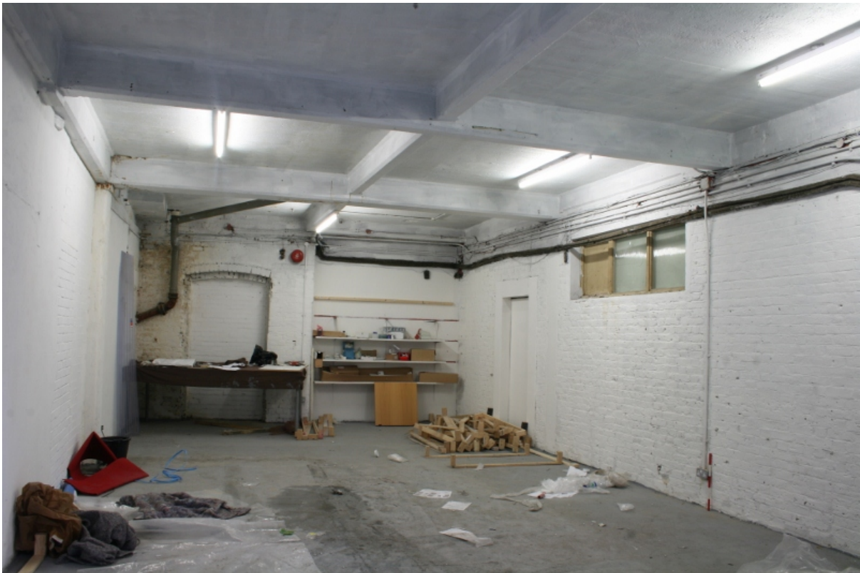
Plate 39: Two blocked doorways in room B2G1, looking south (VAL14 D100 (27))
