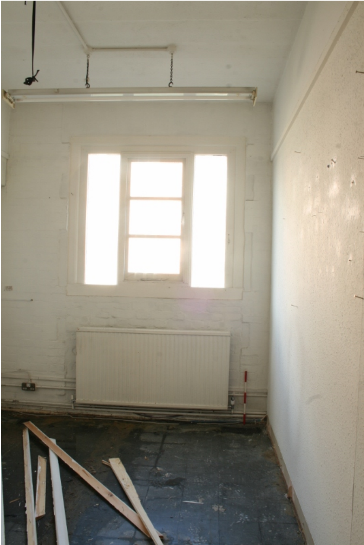
Plate 78: Replacement window in first floor room B2F2, looking west (VAL14 D100 (96))
