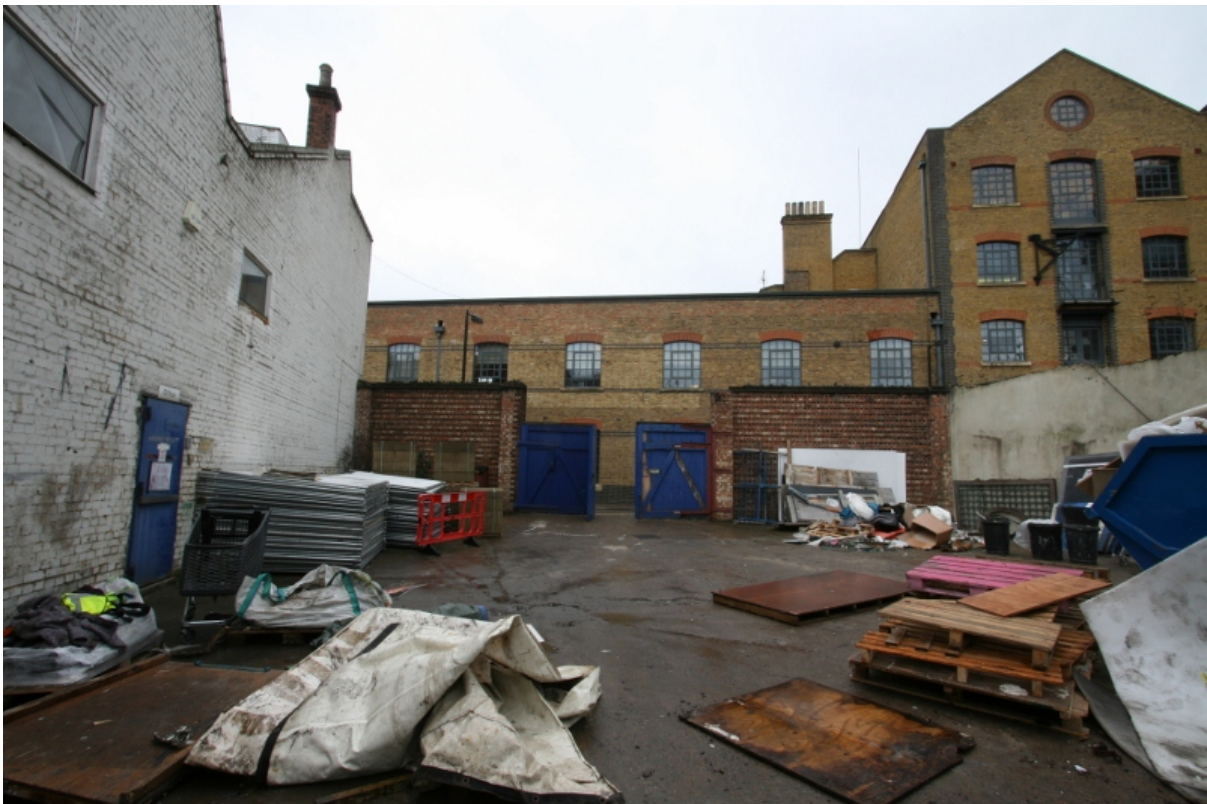
Plate 13: Rear view (west side) of entrance gate and wall of nos 3-5 Valentine Place, looking west (VAL14 D100(136))
