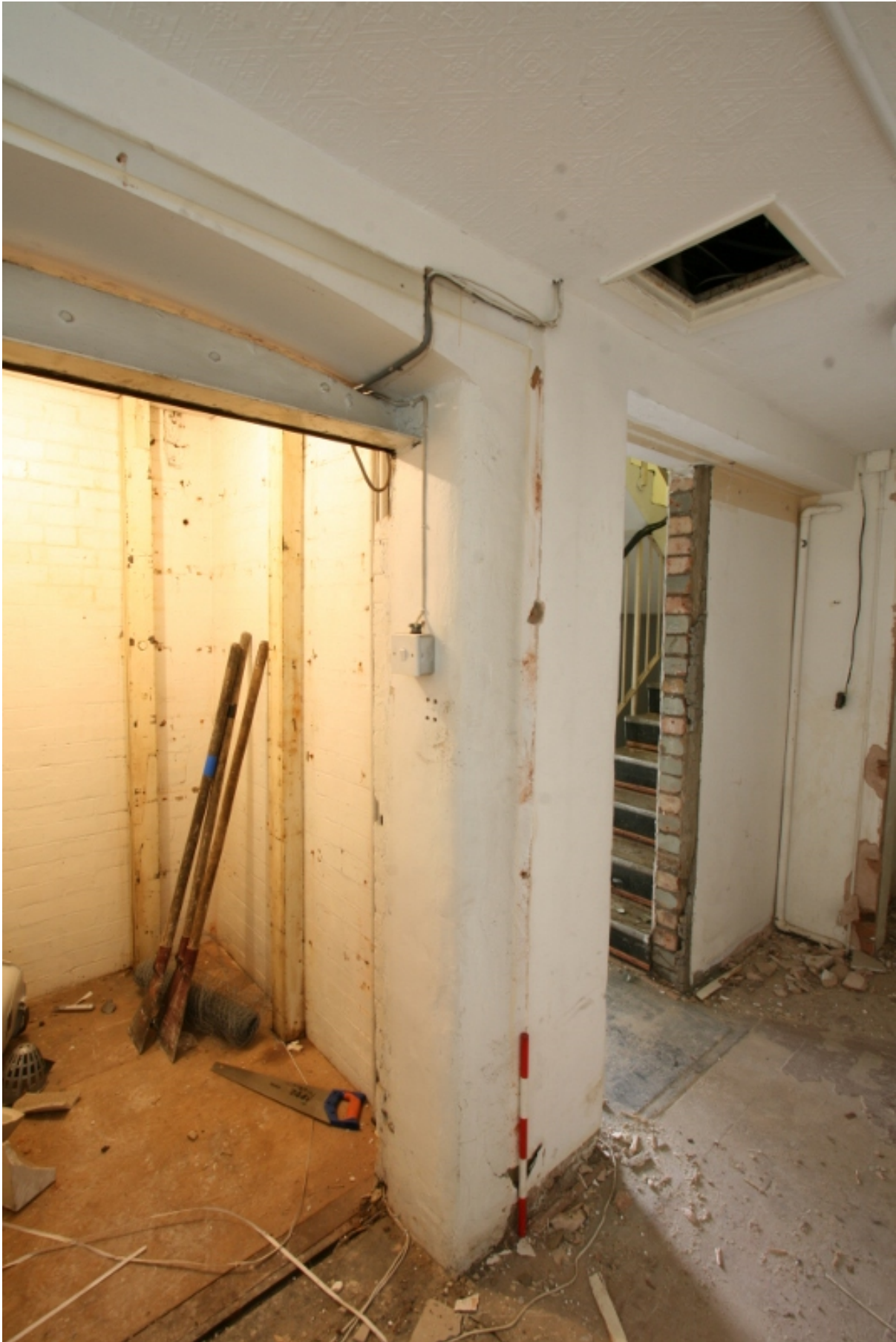
Plate 76: Converted lift shaft and inserted stairwell, looking north-west (VAL14 D100 (92))
