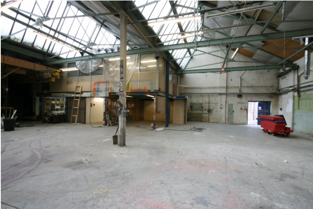
Plate 18: Room B1G1 with inserted mezzanine level and saw-tooth roof, looking north (VAL14 D100 (131))
