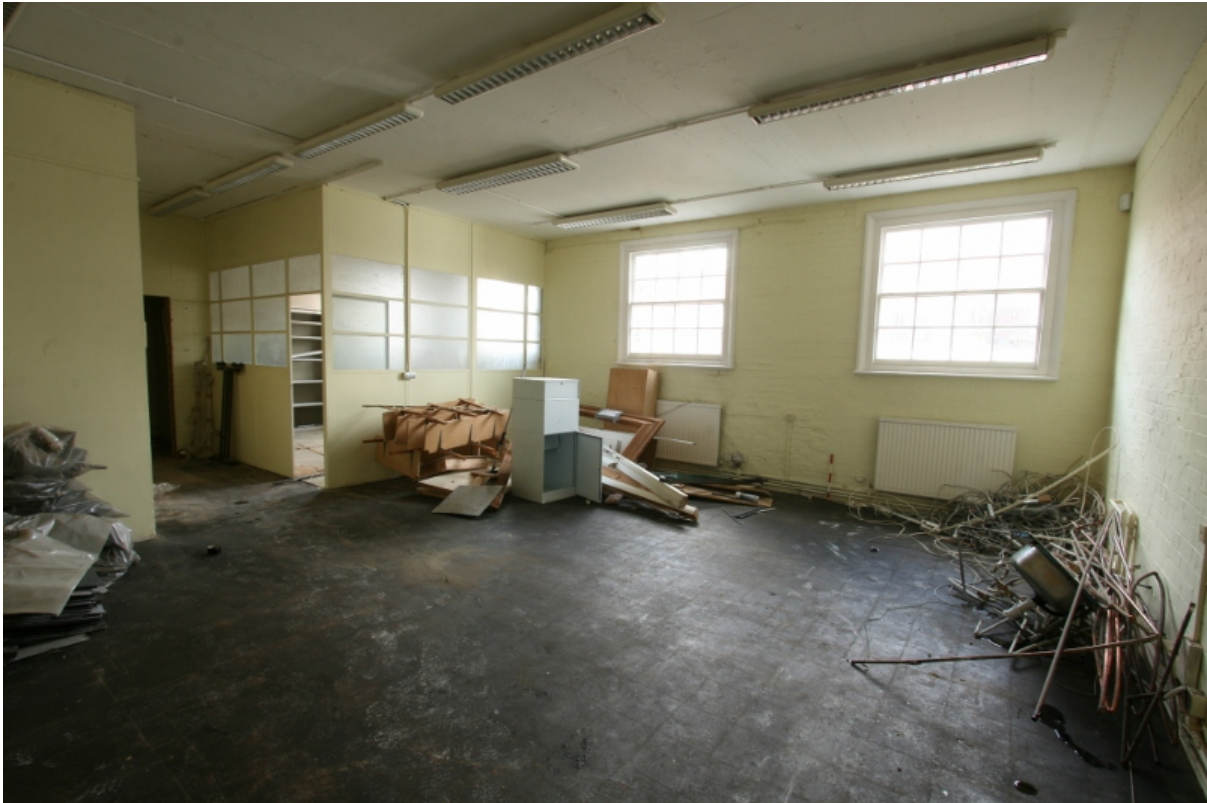
Plate 85: Inserted partitioning in second floor room B2S1, looking south-west (VAL14 D100 (99))
