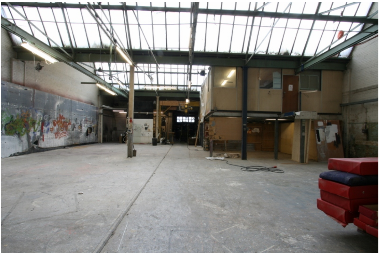
Plate 15: Room B1G1 with inserted mezzanine level (right), looking west (VAL14 D100 (128))
