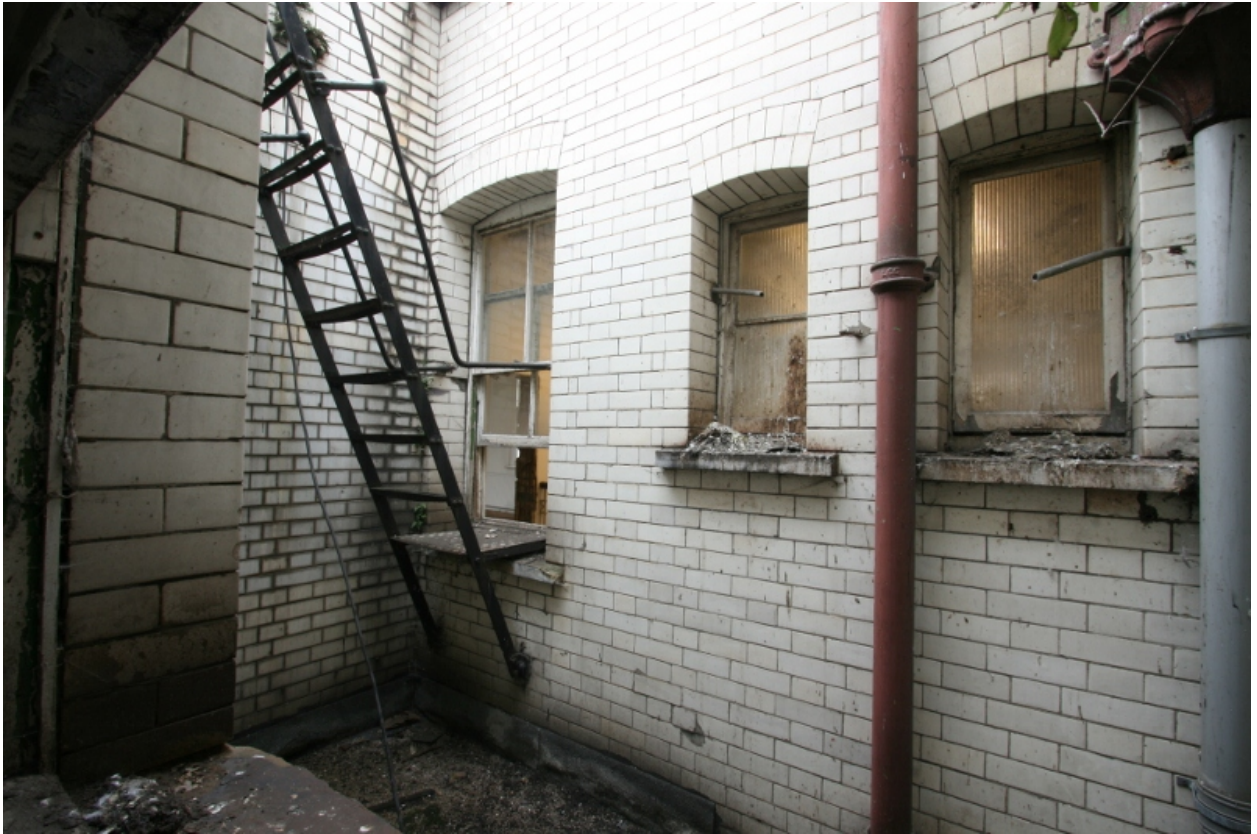
Plate 75: Lightwell in first floor, looking south-west (VAL14 D100 (117))
