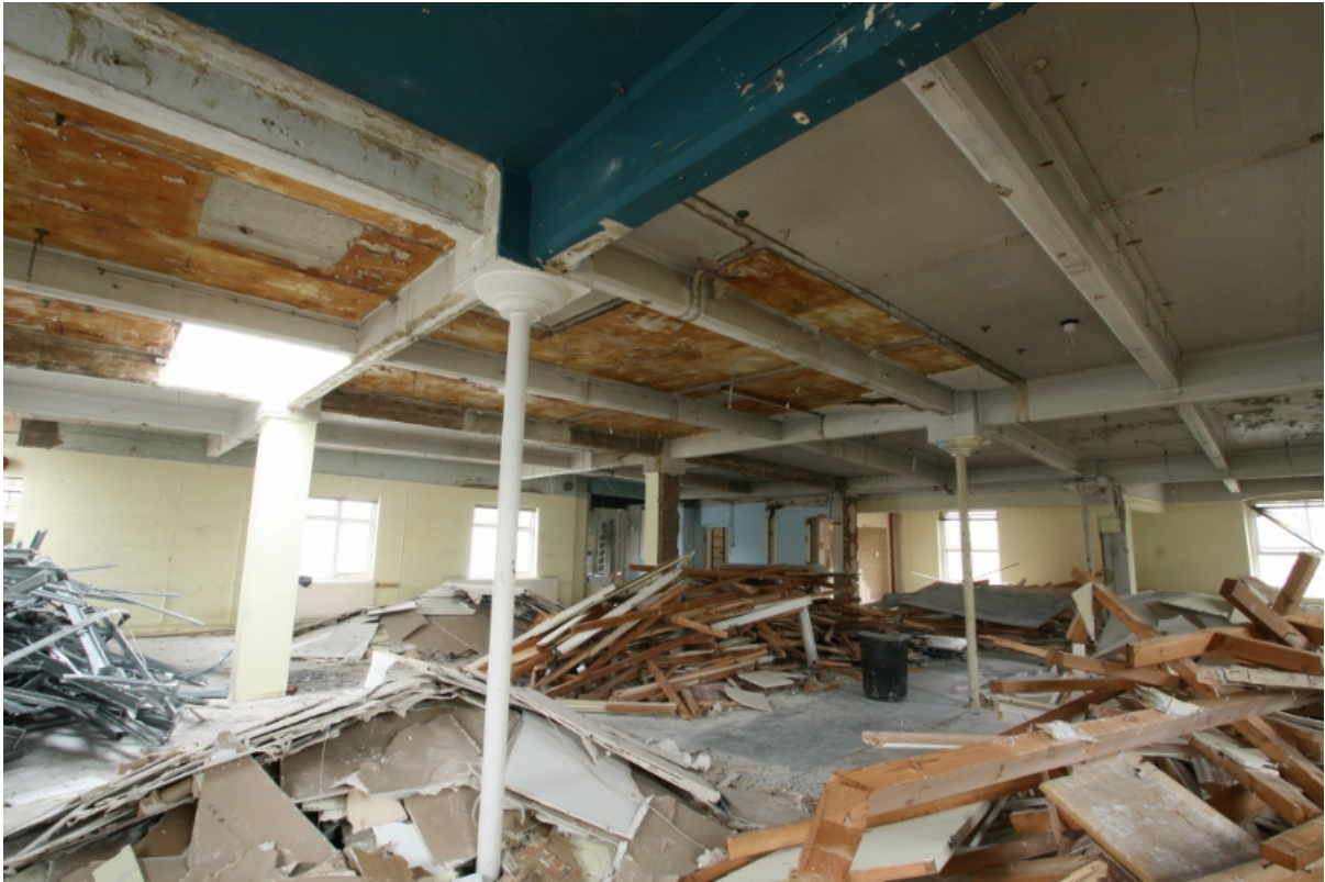
Plate 87: Original cast iron columns in foreground and concrete encased columns behind in second floor room B2S2, looking north-east (VAL14 D100 (121))
