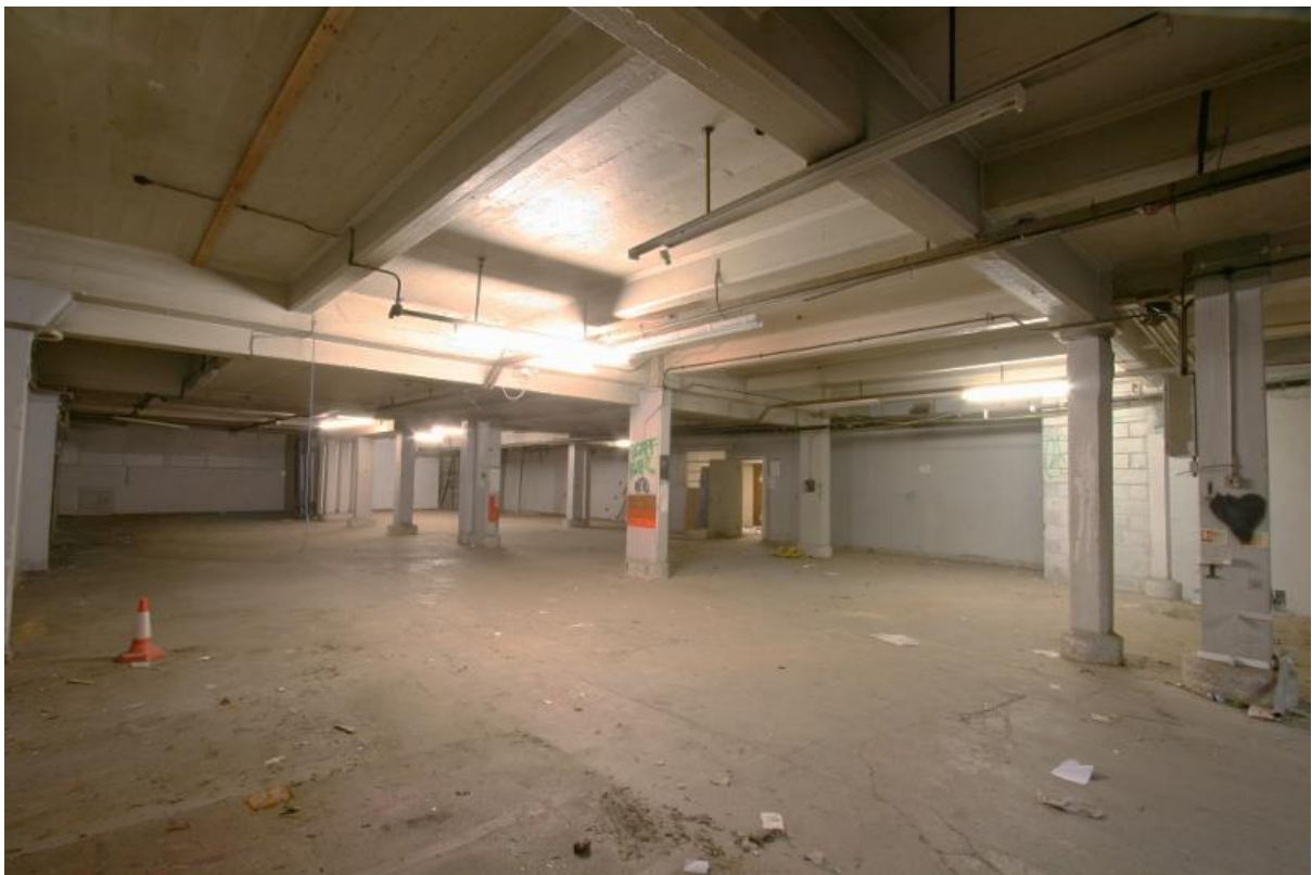
Plate 44: Concrete columns in ground floor room B2G3, looking south-west (VAL14 D100 (20))
