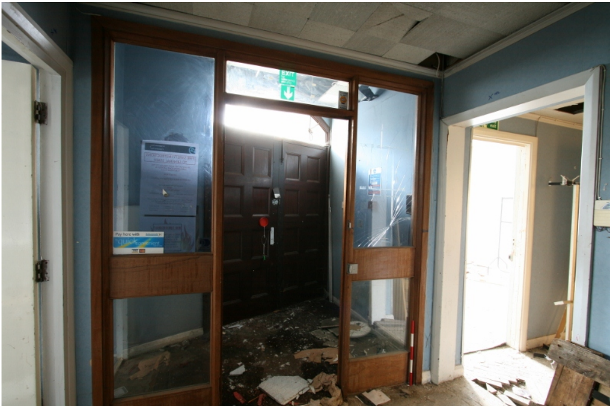
Plate 64: Webber Street entrance hallway, looking south-west (VAL14 D100 (47))
