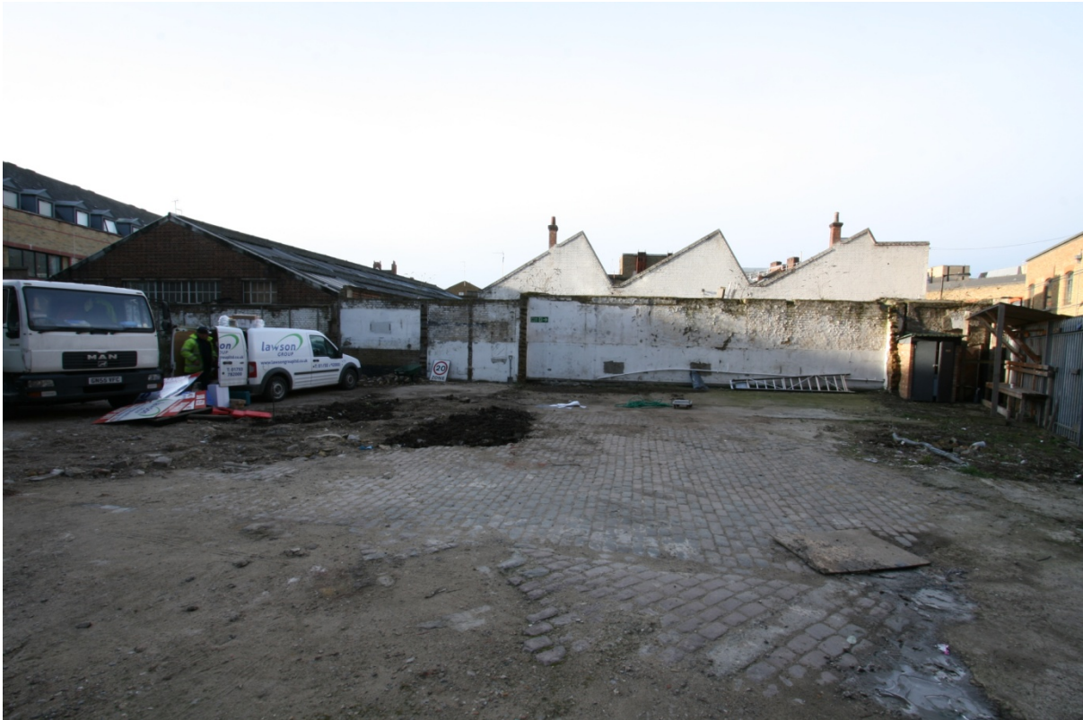
Plate 2: External south walls and yard area of former no. 1 Valentine Place immediately in front (north) of nos 3-5 Valentine Place, looking south (VAL14 D100 (3))
