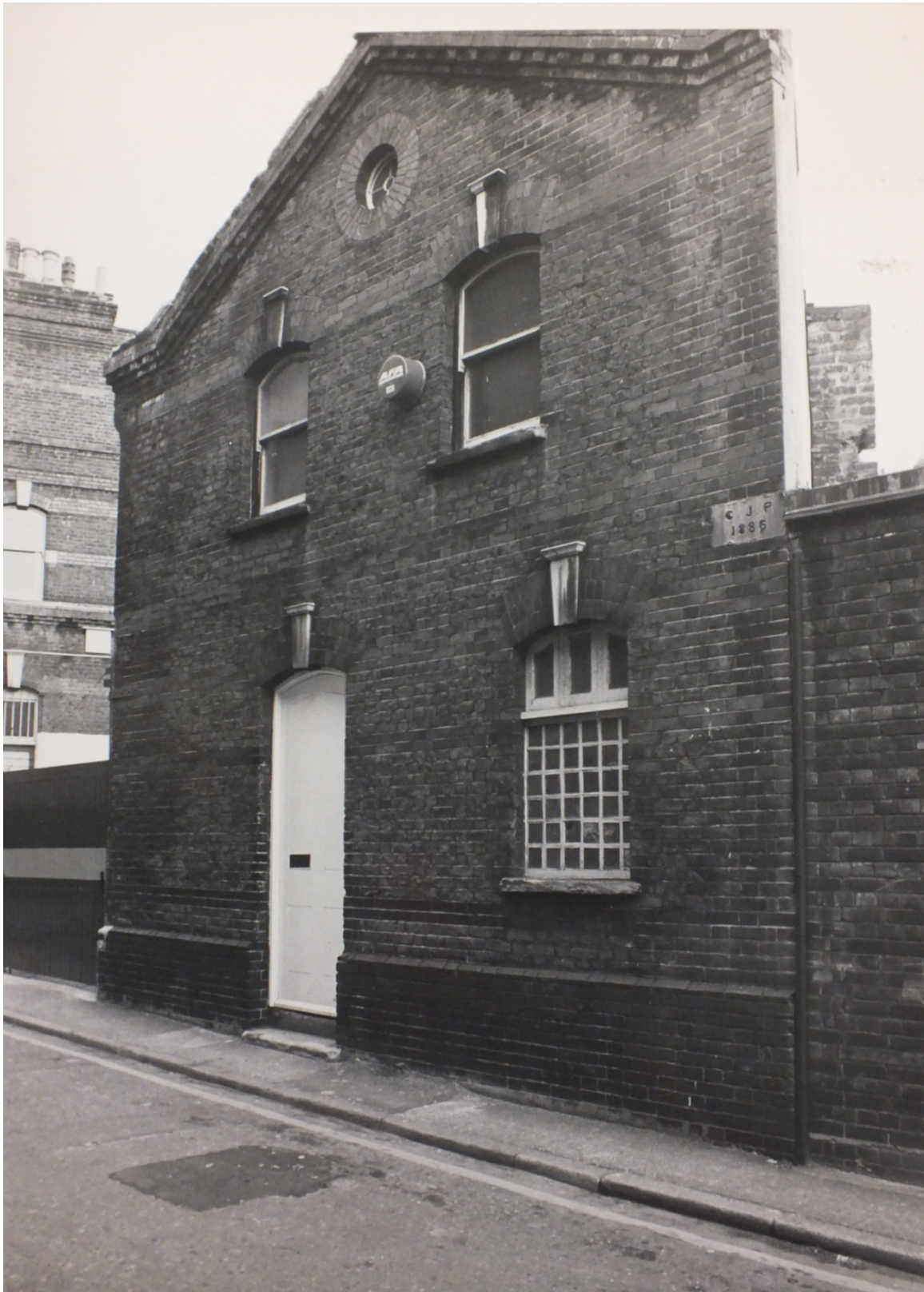
Plate A: Photograph taken in 1977 of No. 1 Valentine Place when it was occupied by Gladding Construction Company, looking north-east (courtesy of Southwark Local Studies Archive)
