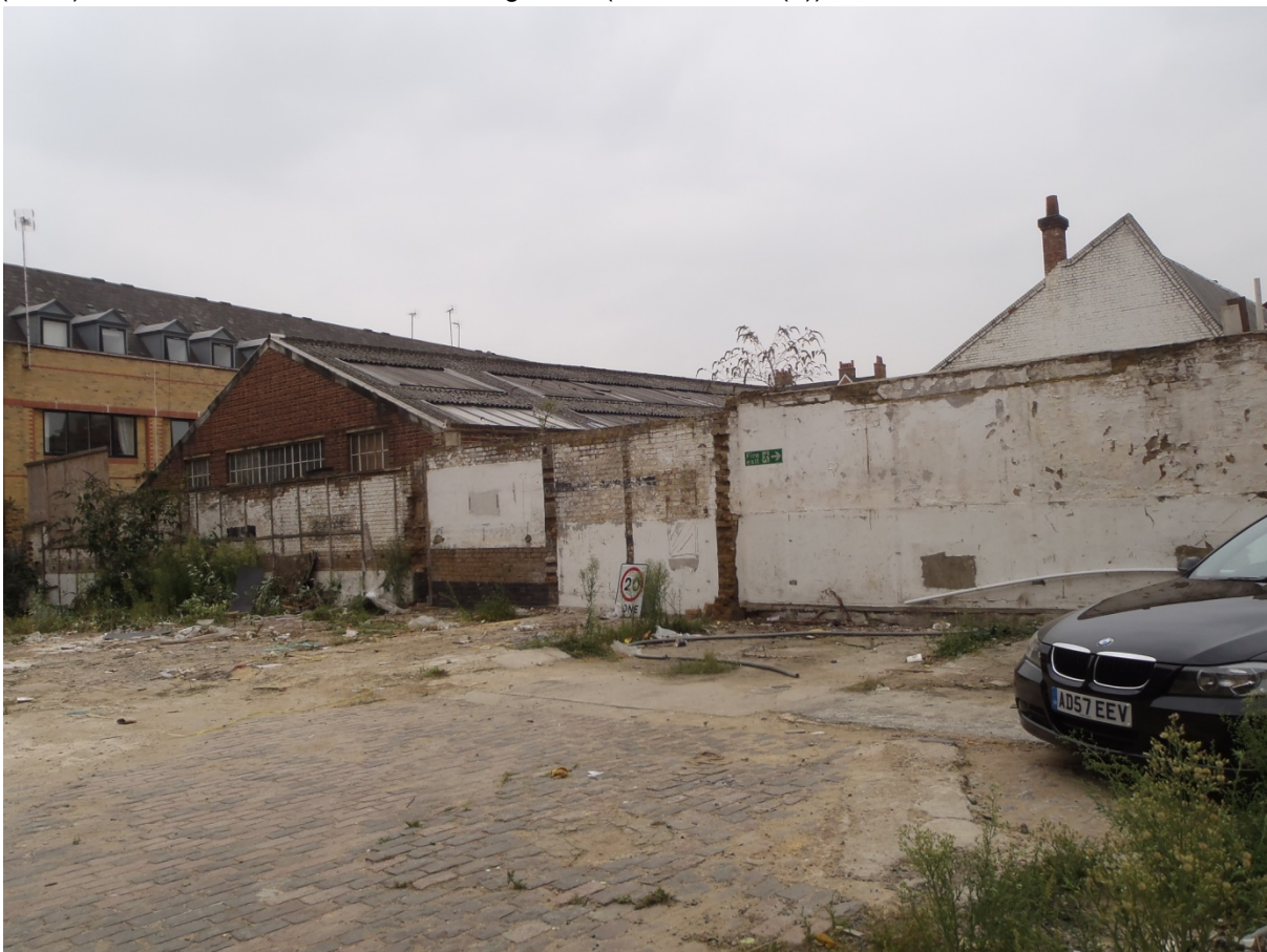
Plate 3: External south walls and yard area of former no. 1 Valentine Place immediately in front (north) of nos 3-5 Valentine Place, looking south-east
