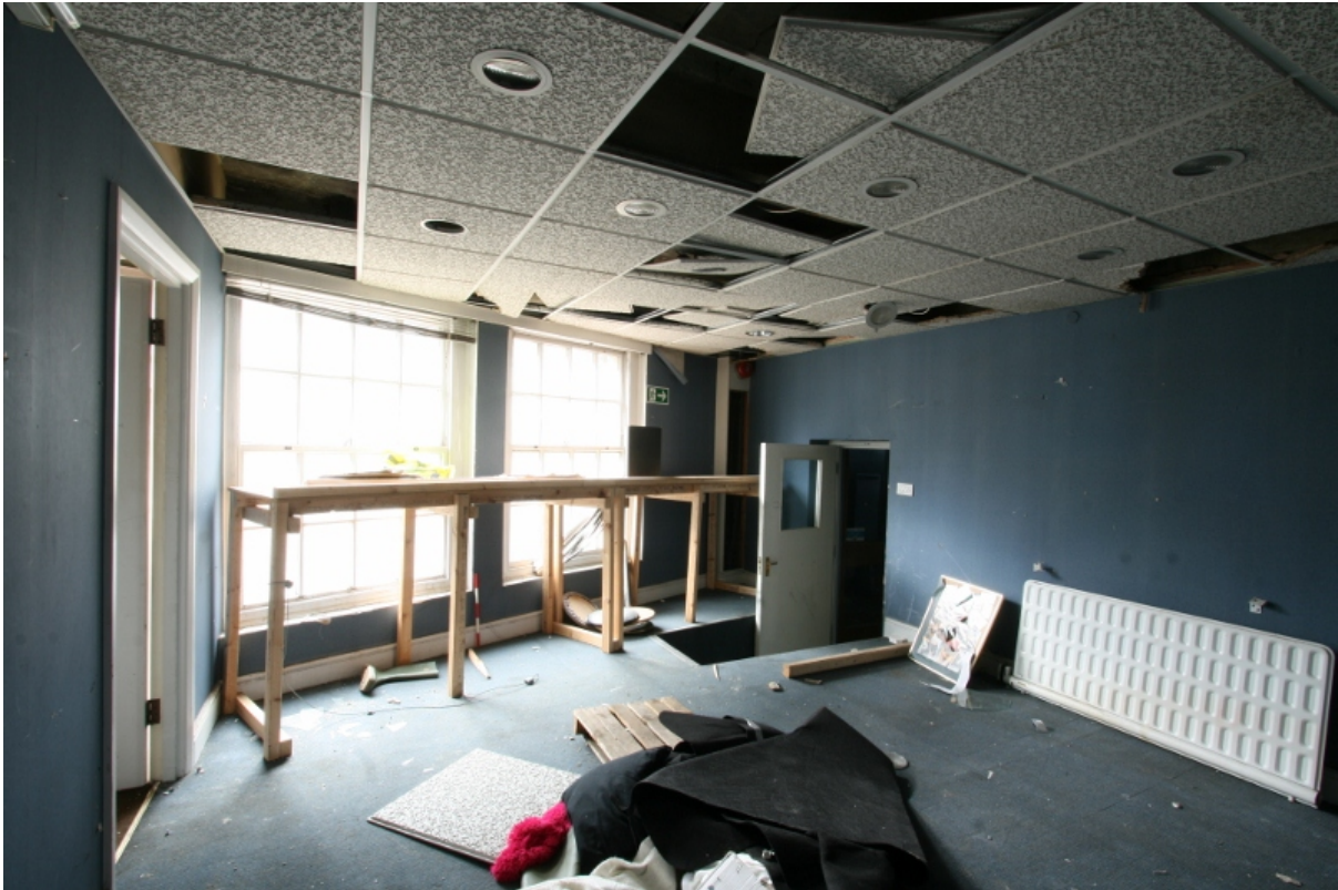
Plate 65: Ground floor room B2G18 with modern raised floors and suspended ceiling, looking southwest (VAL14 D100 (48))
