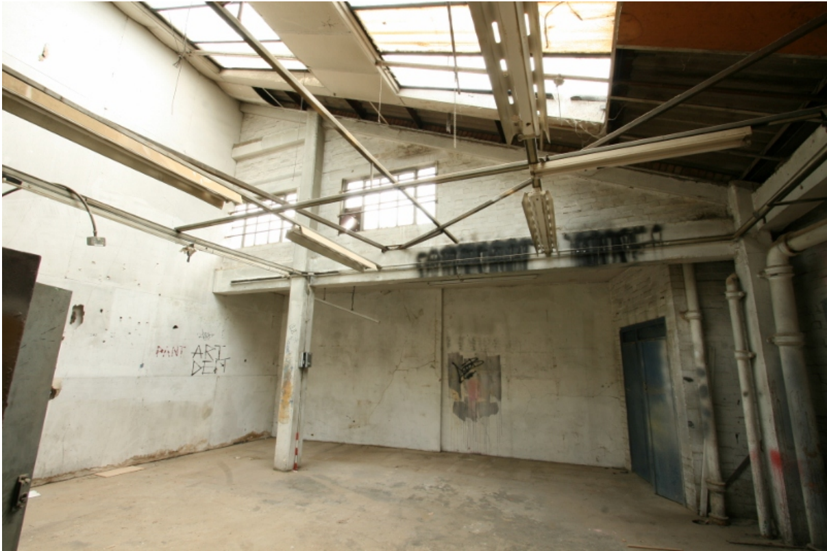
Plate 29: Room B1G5, looking north (VAL14 D100 (73))
