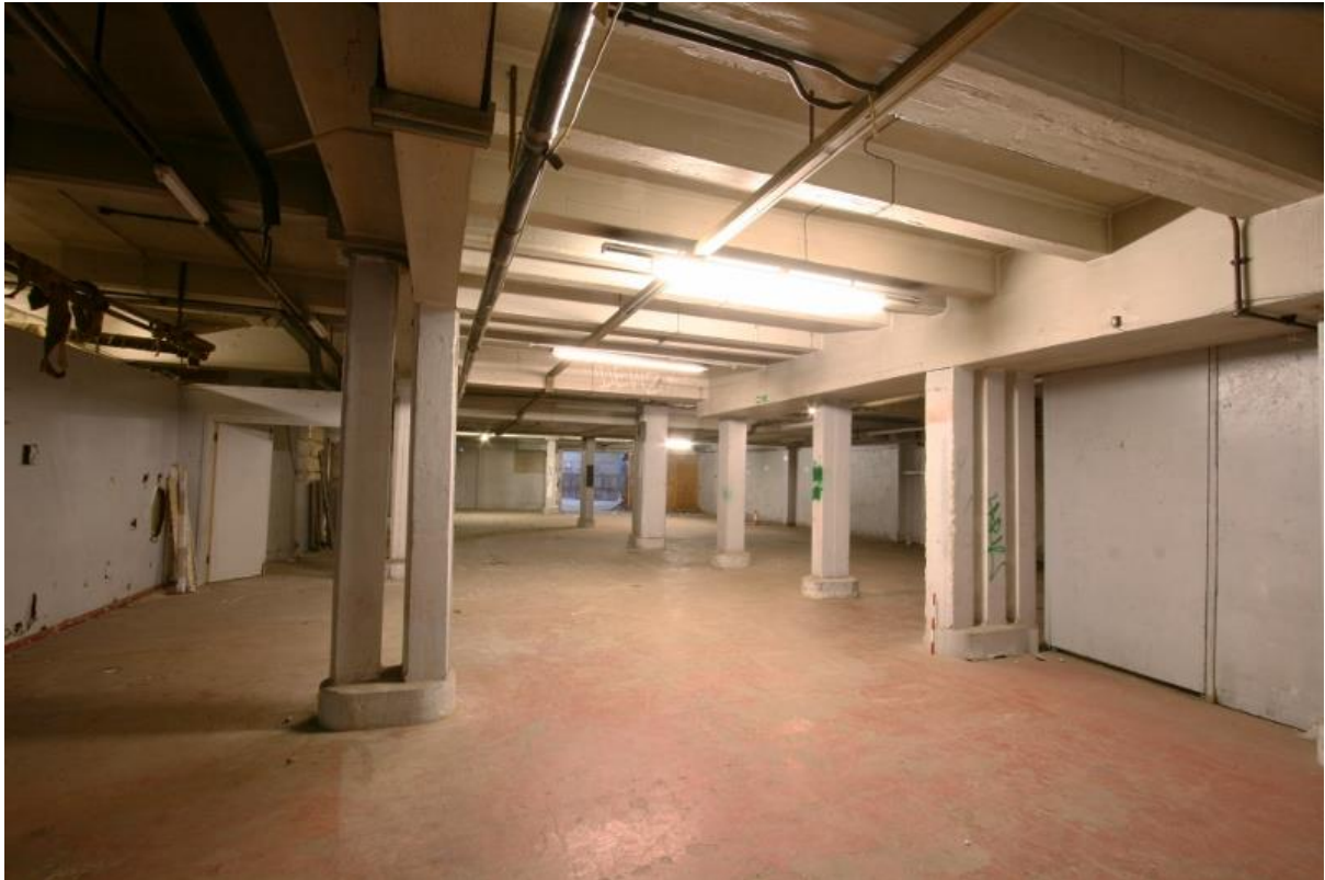
Plate 43: Concrete columns in ground floor room B2G3, looking north-east (VAL14 D100 (21))
