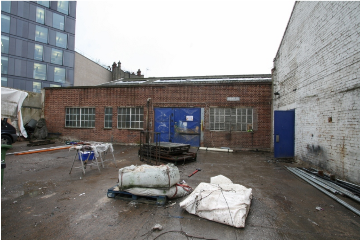
Plate 12: Single storey north-south aligned warehouse of nos 3-5 Valentine Place, looking east (VAL14 D100(135))
