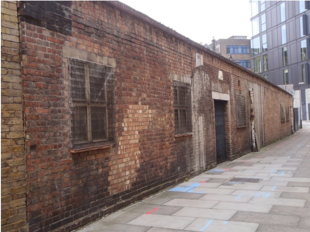
Plate 9: Rear (east) of nos 3-5 Valentine Place fronting onto Valentine Row, looking north-west
