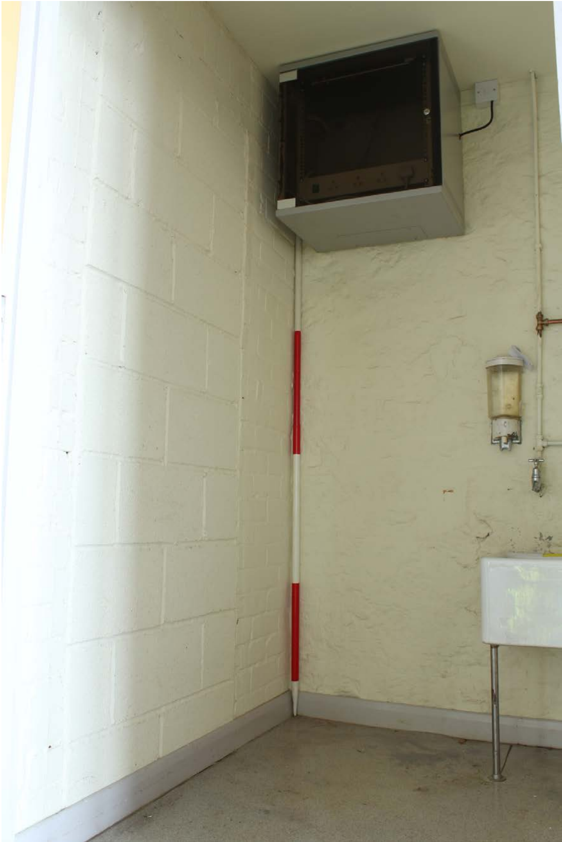
Plate 28: Blocked doorway in room B1G2, looking south-east (WDS15 D1 (39))
