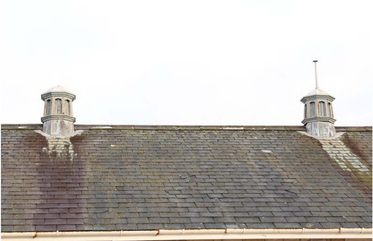
Plate 27: Vents on roof, looking up and east (WDS15 D1 (35))
