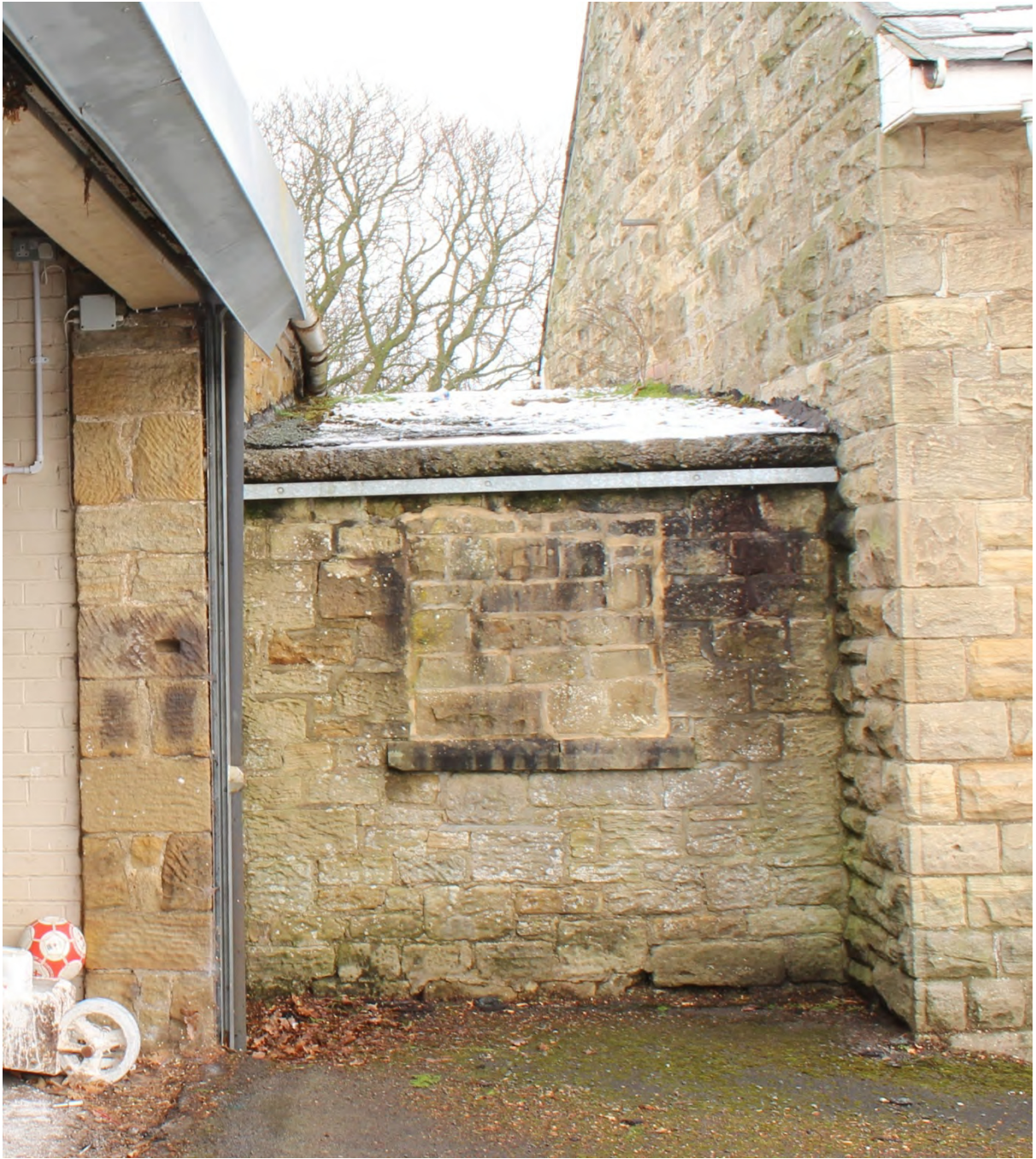
Plate 33: Blocked rear window of link room, looking east (WDS15 D1 (22 zoomed in))
