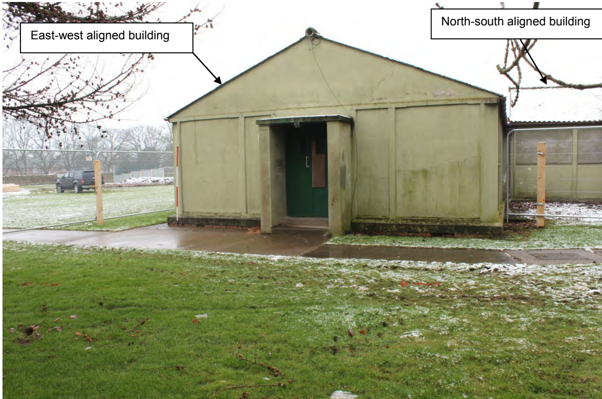
Plate 1: Front entrance into the Pavilion, looking west (WDS15 D1 (7))
