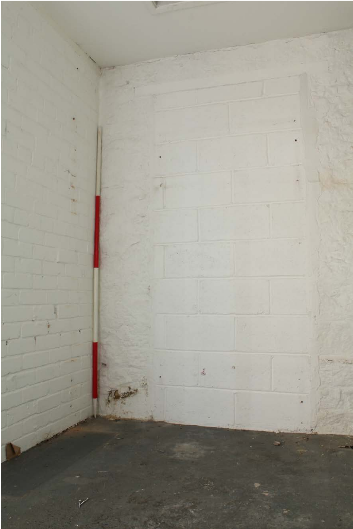
Plate 30: Blocked doorway and inserted brick wall in room B1G6, looking west (WDS15 D1 (42))
