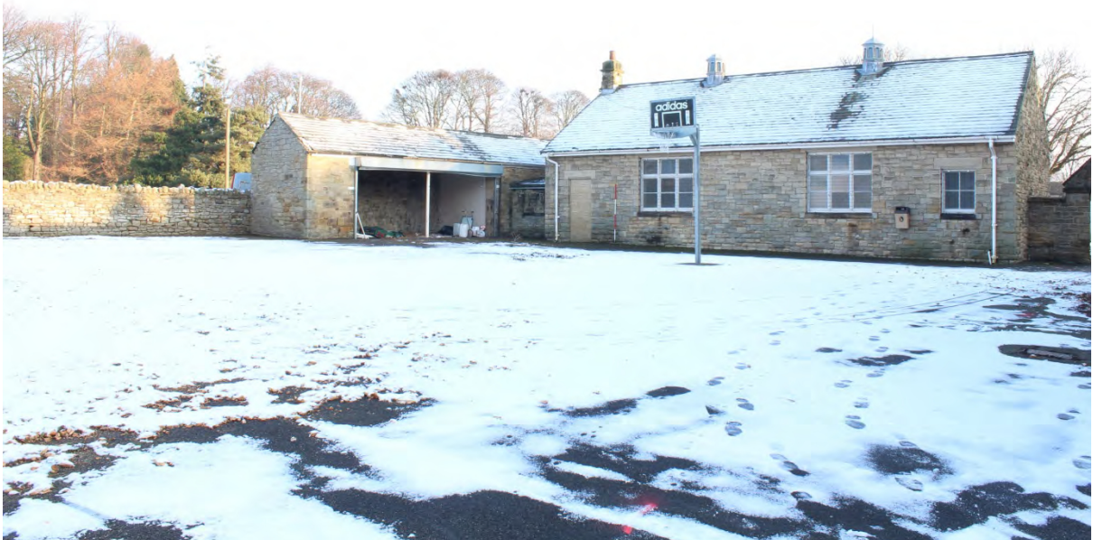
Plate 22: West elevation of music room outbuilding and south elevation of converted outbuilding, looking west (WDS15 D1 (16))
