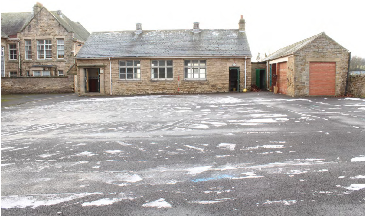
Plate 20: East elevation of music room outbuilding, looking west (WDS15 D1 (32))
