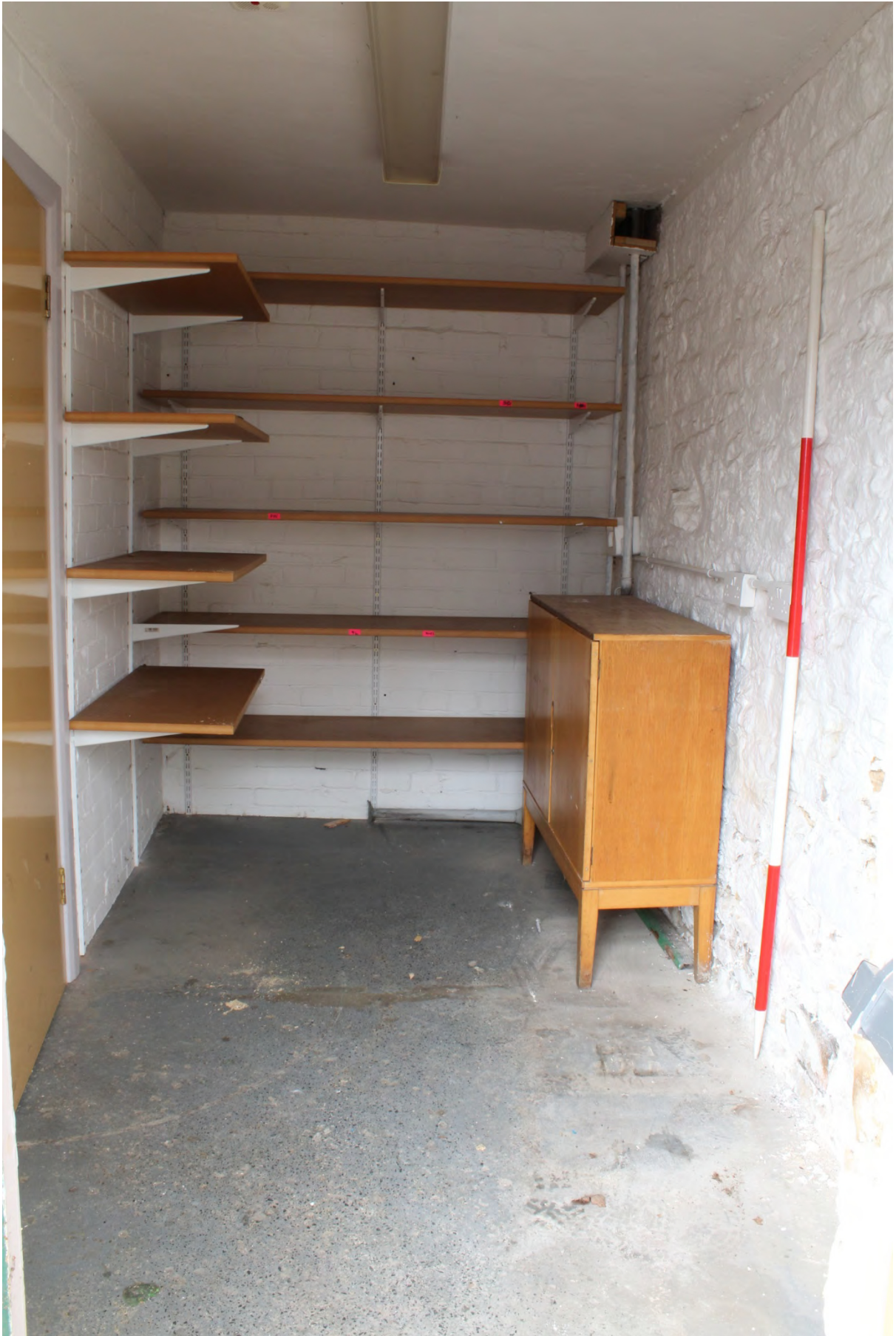
Plate 31: Brick walls in room B1G5, looking west (WDS15 D1 (43))
