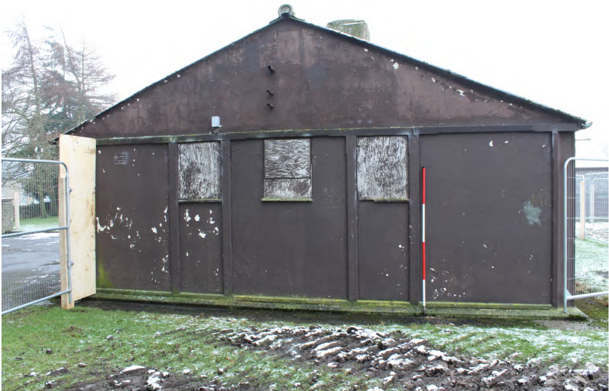
Plate 4: North gable end elevation of the Pavilion, looking south (WDS15 D1 (3))
