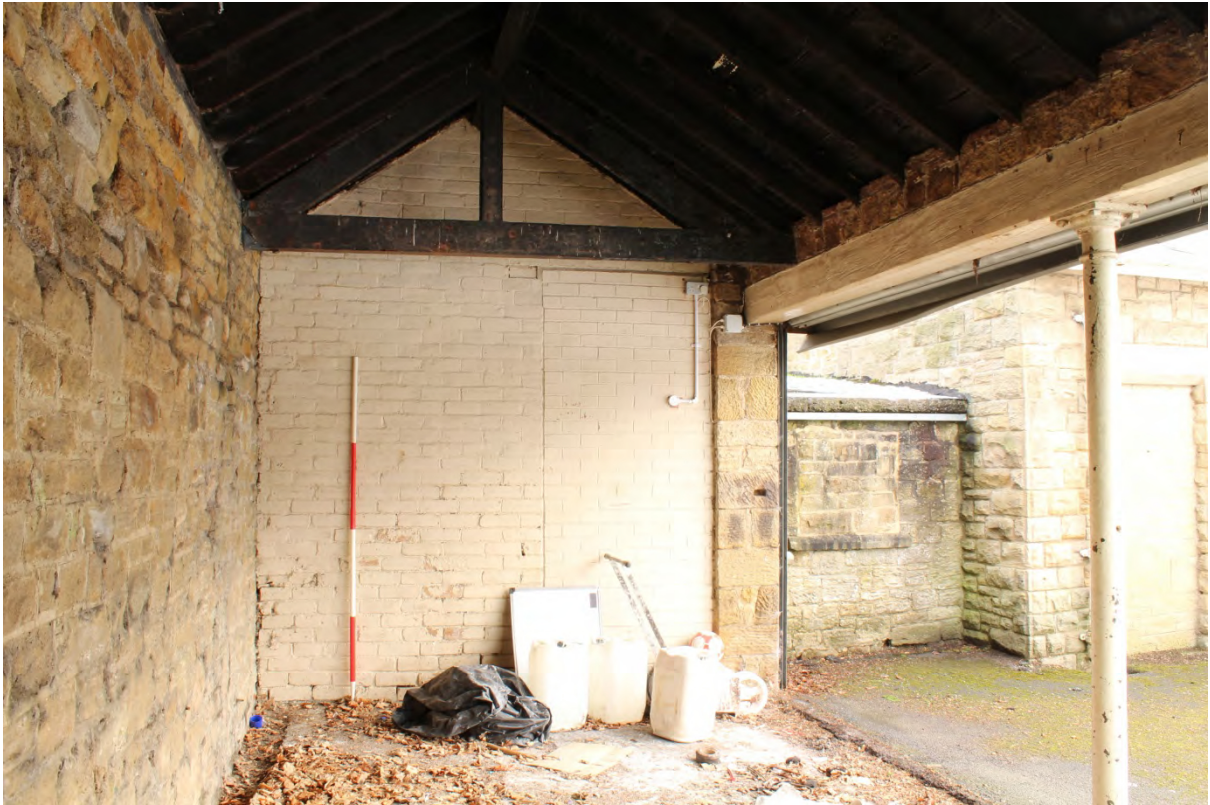
Plate 37: Interior of storage space (B2G1) showing blocked doorway, looking east (WDS15 D1 (23))
