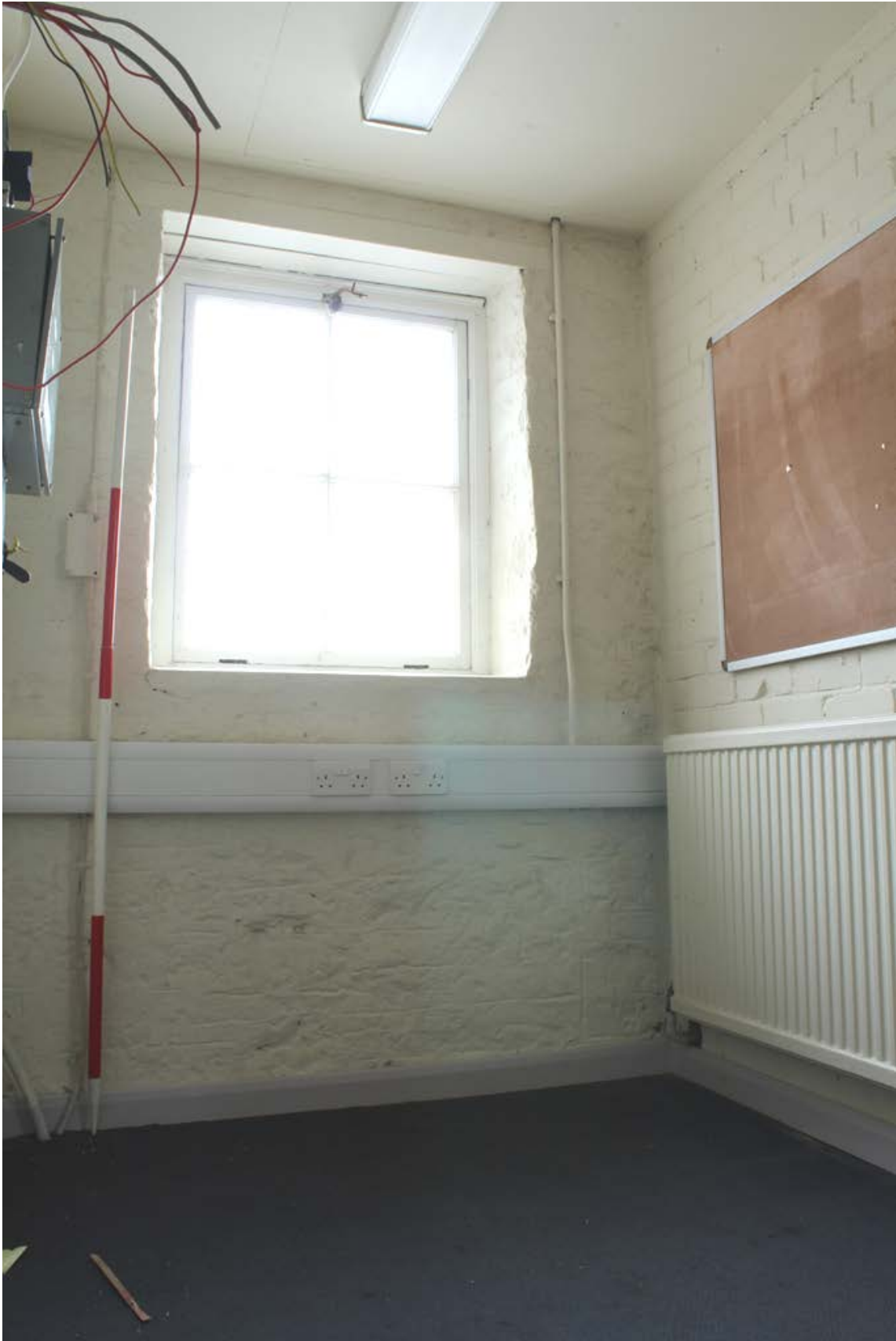
Plate 29: Window in west wall of room a and inserted brick wall on right, looking north-west (WDS15 D1 (40))
