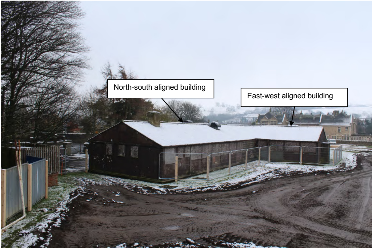
Plate 3: Rear elevations of the Pavilion, looking south-east, (WDS15 D1 (1))
