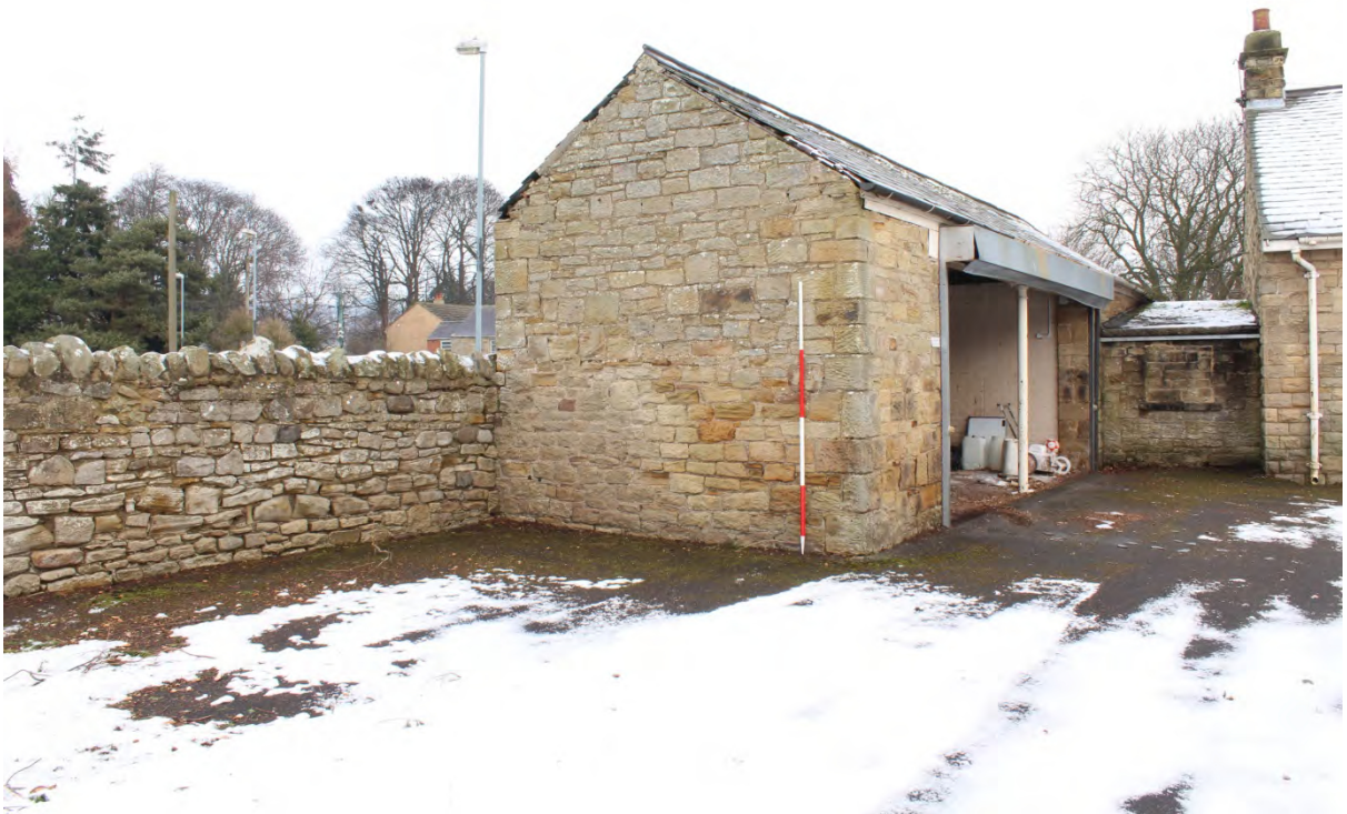
Plate14: Low perimeter wall and converted outbuilding, looking north-east (WDS15 D1 (21))
