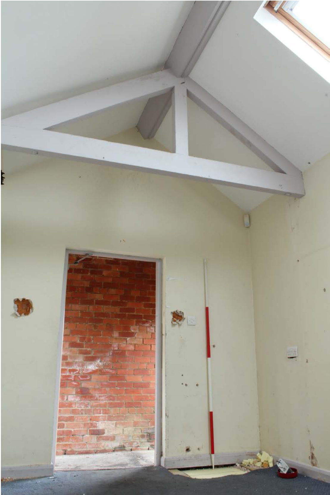
Plate 42: Room B2G4 with overhead timber truss, looking west (WDS15 D1 (47))
