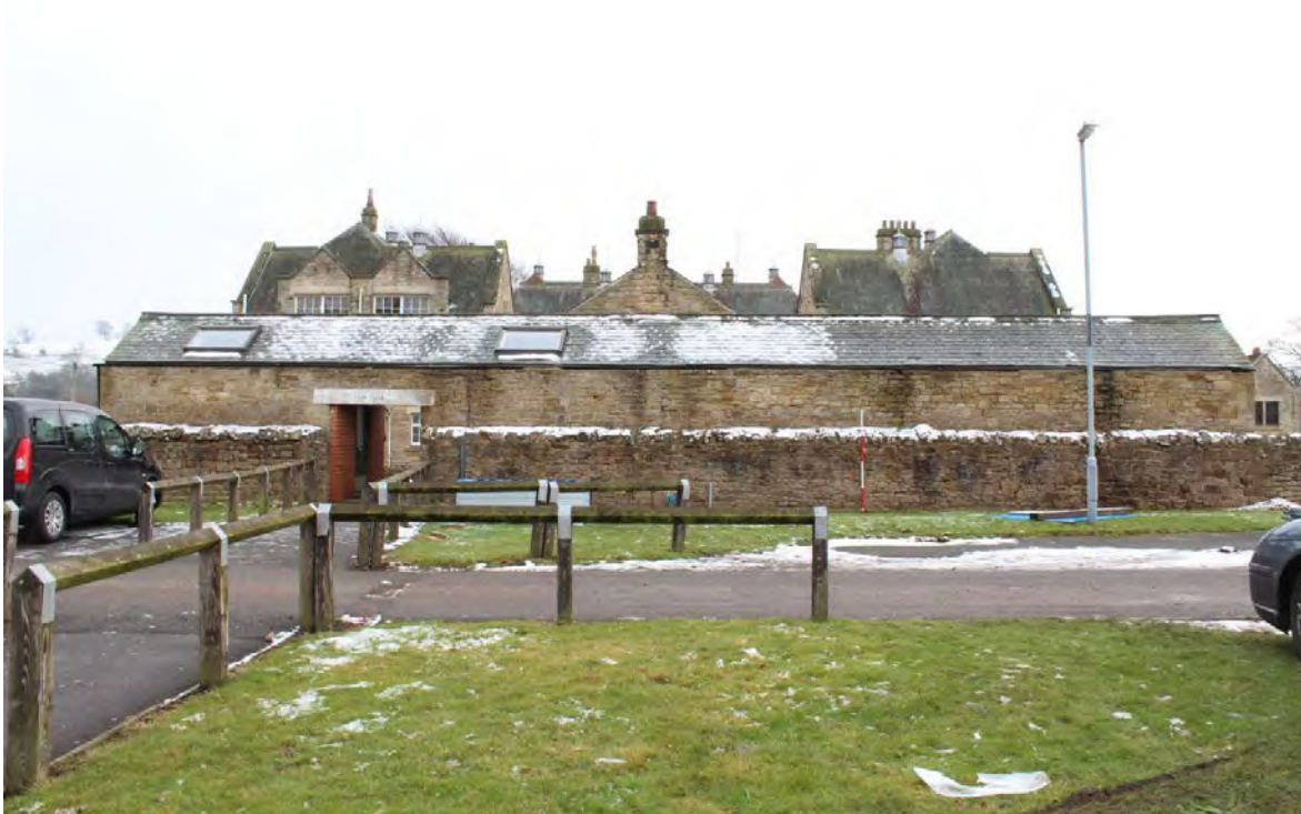
Plate 8: Low perimeter wall with outbuilding and school building behind, looking south (WDS15 D1 (29))
