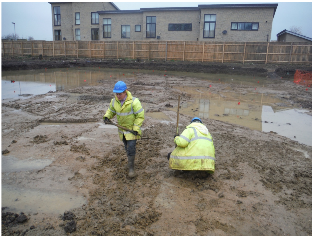
Plate 3: Working shot of trench cleaning in wet conditions, view north-west
