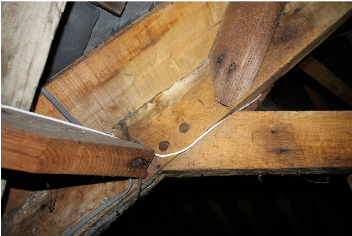
Plate 39 Pegging to Oak Hip Rafter and Collar (Stable C)
