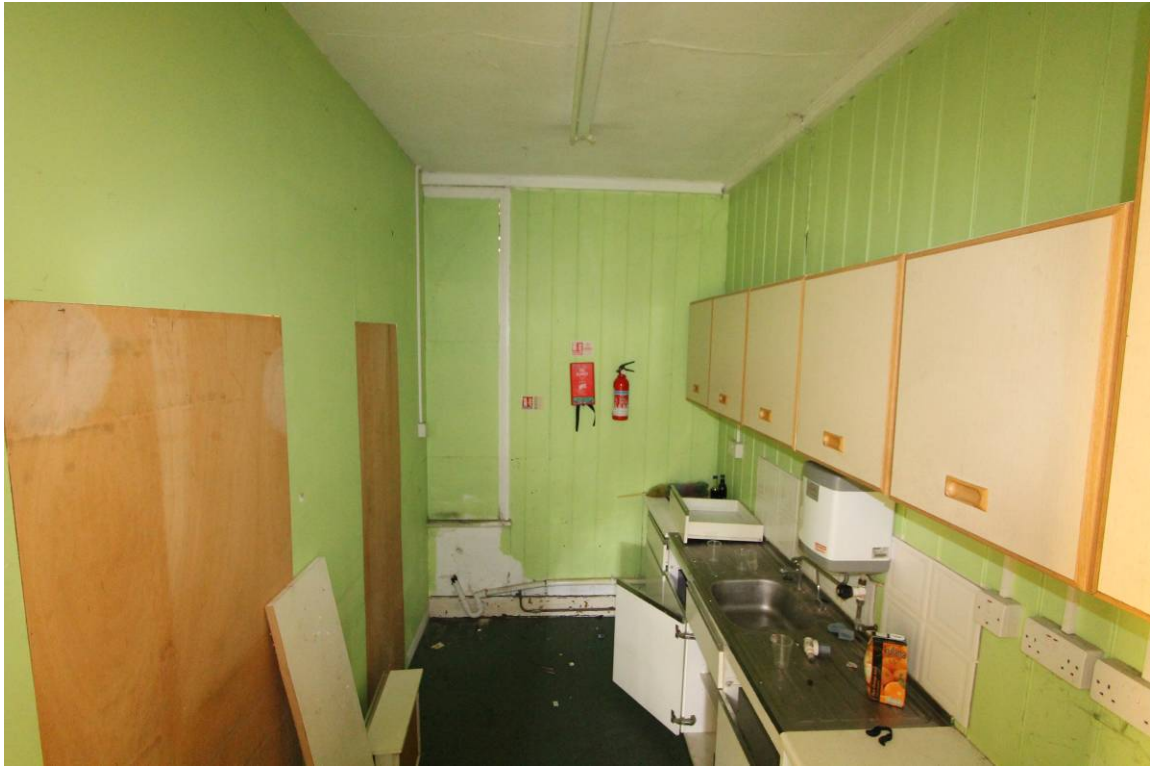
Plate 20 Kitchen (B2) looking W
