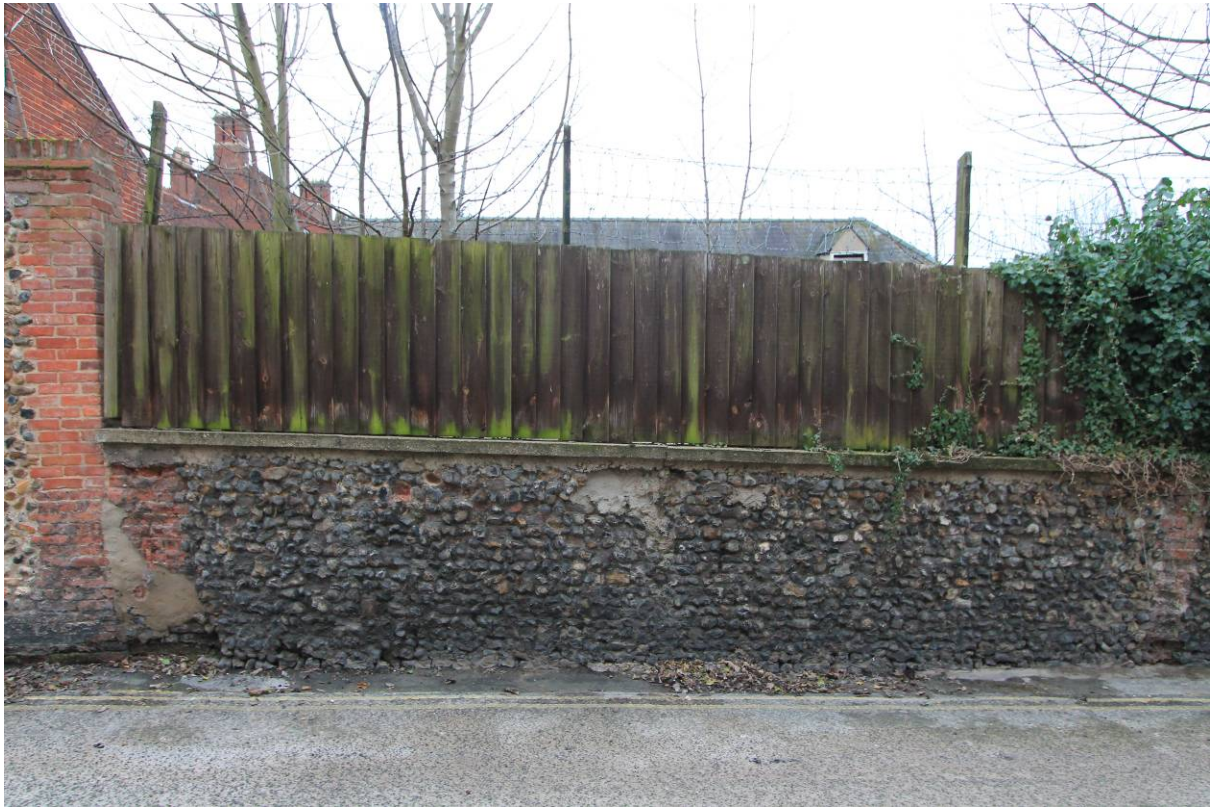
Plate 45 Friars Lane Boundary Wall adjacent to Stable (A)
