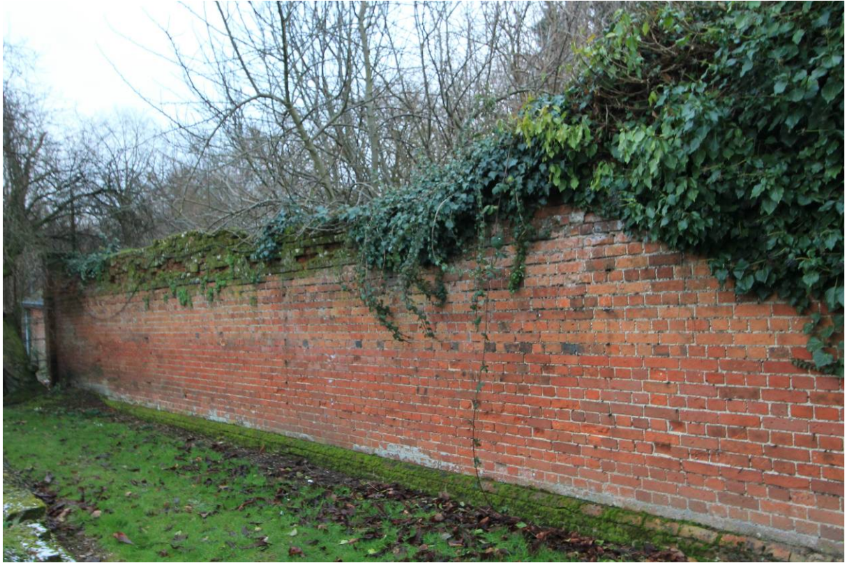
Plate 43 West Garden Wall (W2) looking SW
