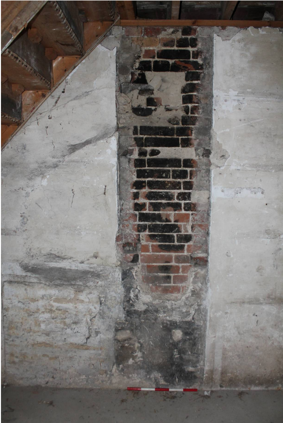
Plate 33 Former Fireplace/Flue in (C5) looking S
