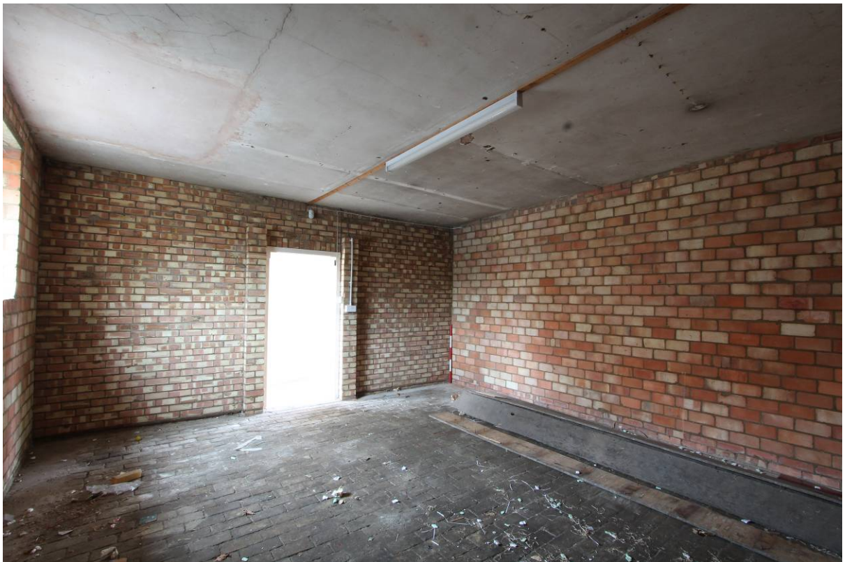
Plate 35 Stable (C) Room (C2) looking NE
