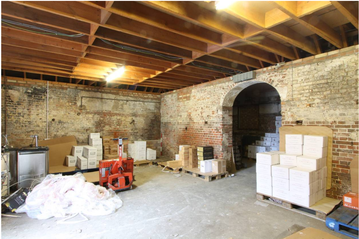
Plate 36 Former Stable (C1) looking SE
