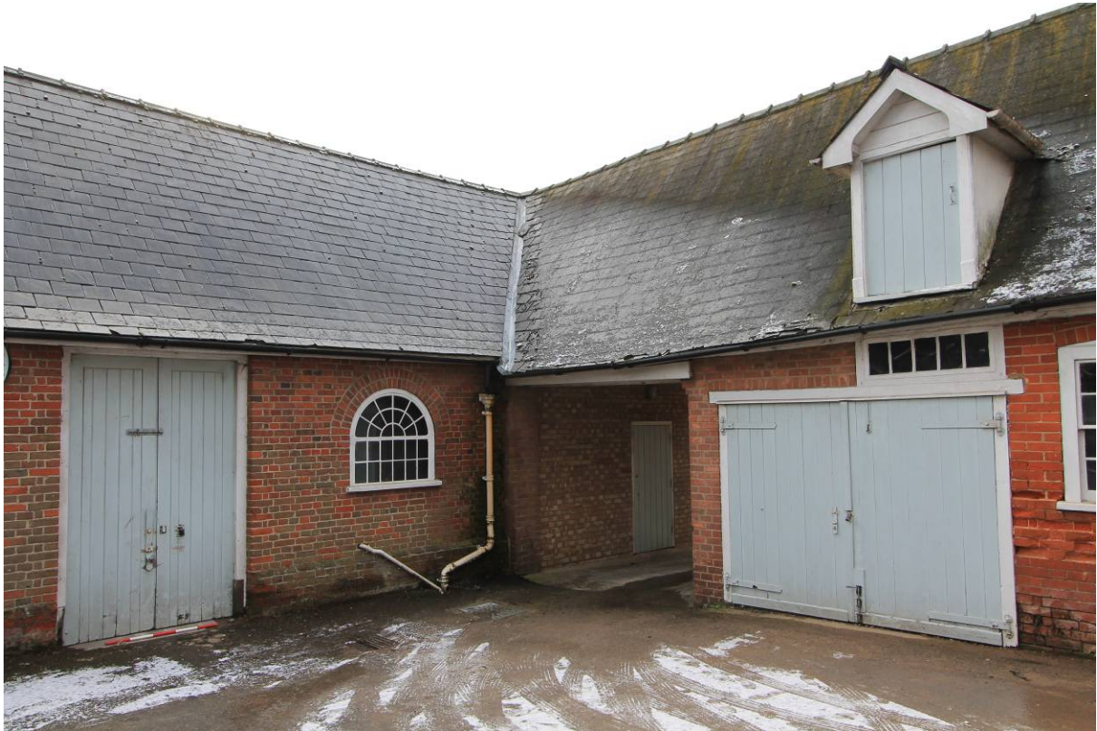
Plate 25 Stable (C) looking SW to Carriageway
