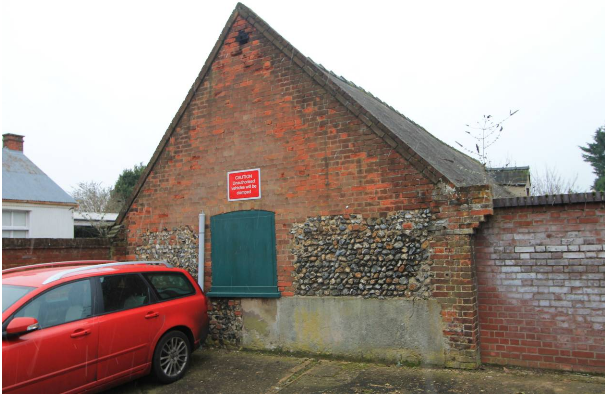
Plate 27 Stable (C) North Gable Elevation looking S
