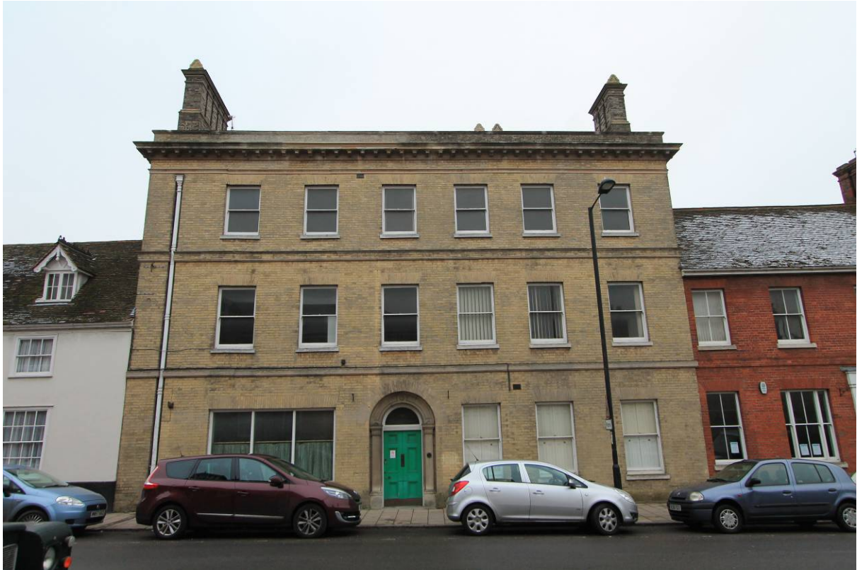
Plate 52 Westgate House, looking S
