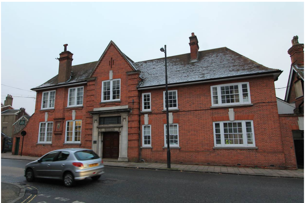
Plate 57 Greene King Offices, looking SE
