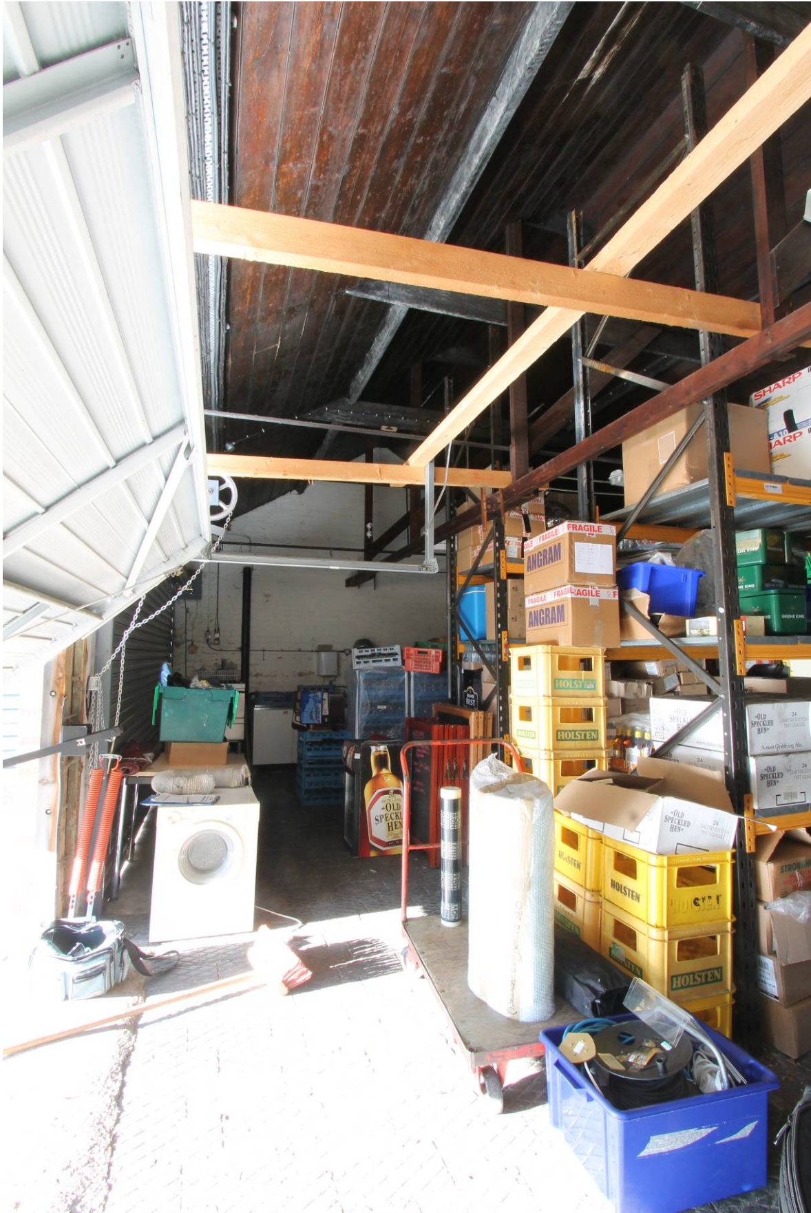
Plate 11 Stable (A) Store (former stabling) (A5) looking W
