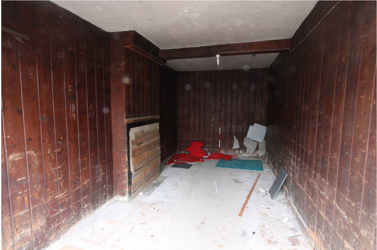
Plate 34 Former Office (C4) looking W
