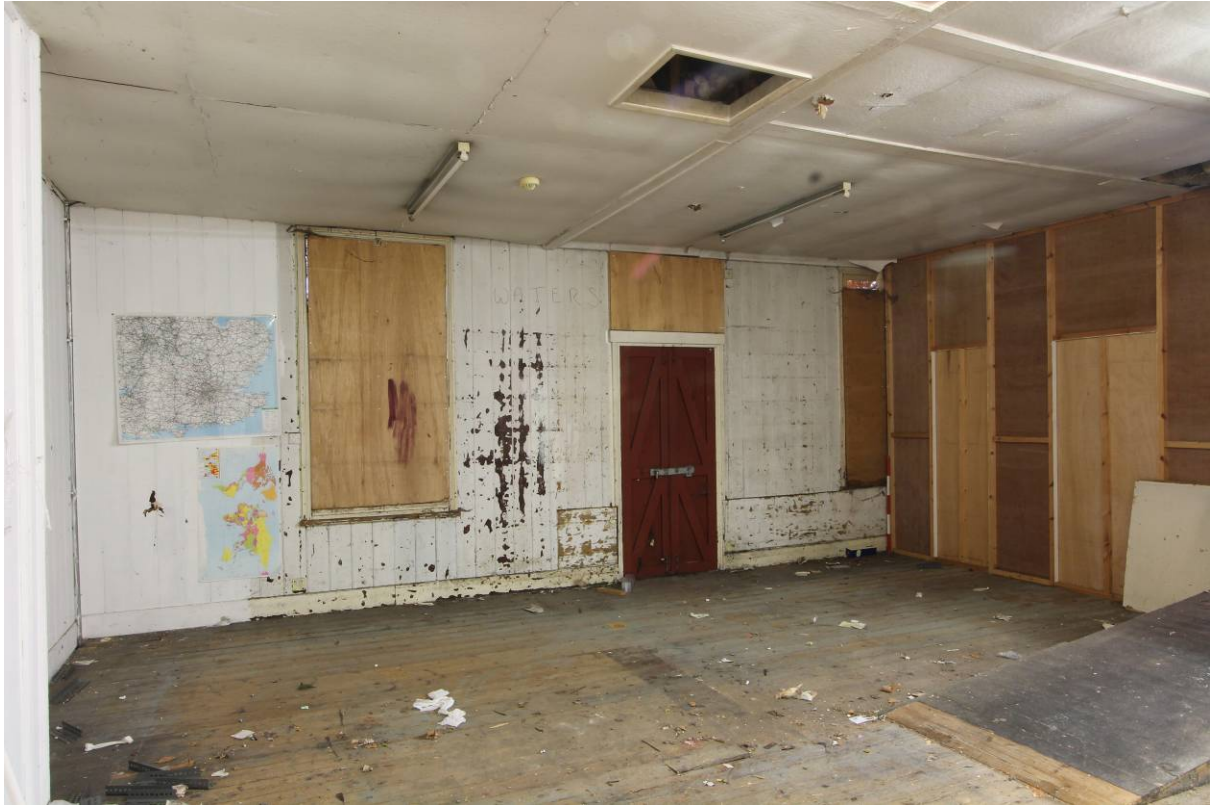
Plate 18 Building (B) looking NW
