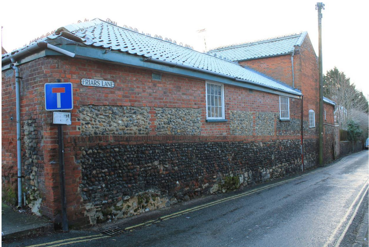
Plate 5 Stable (A) Friars Lane Elevation, looking SE
