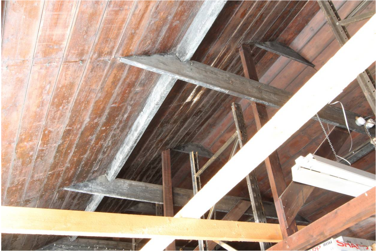
Plate 12 Close boarded roof structure over (A5)
