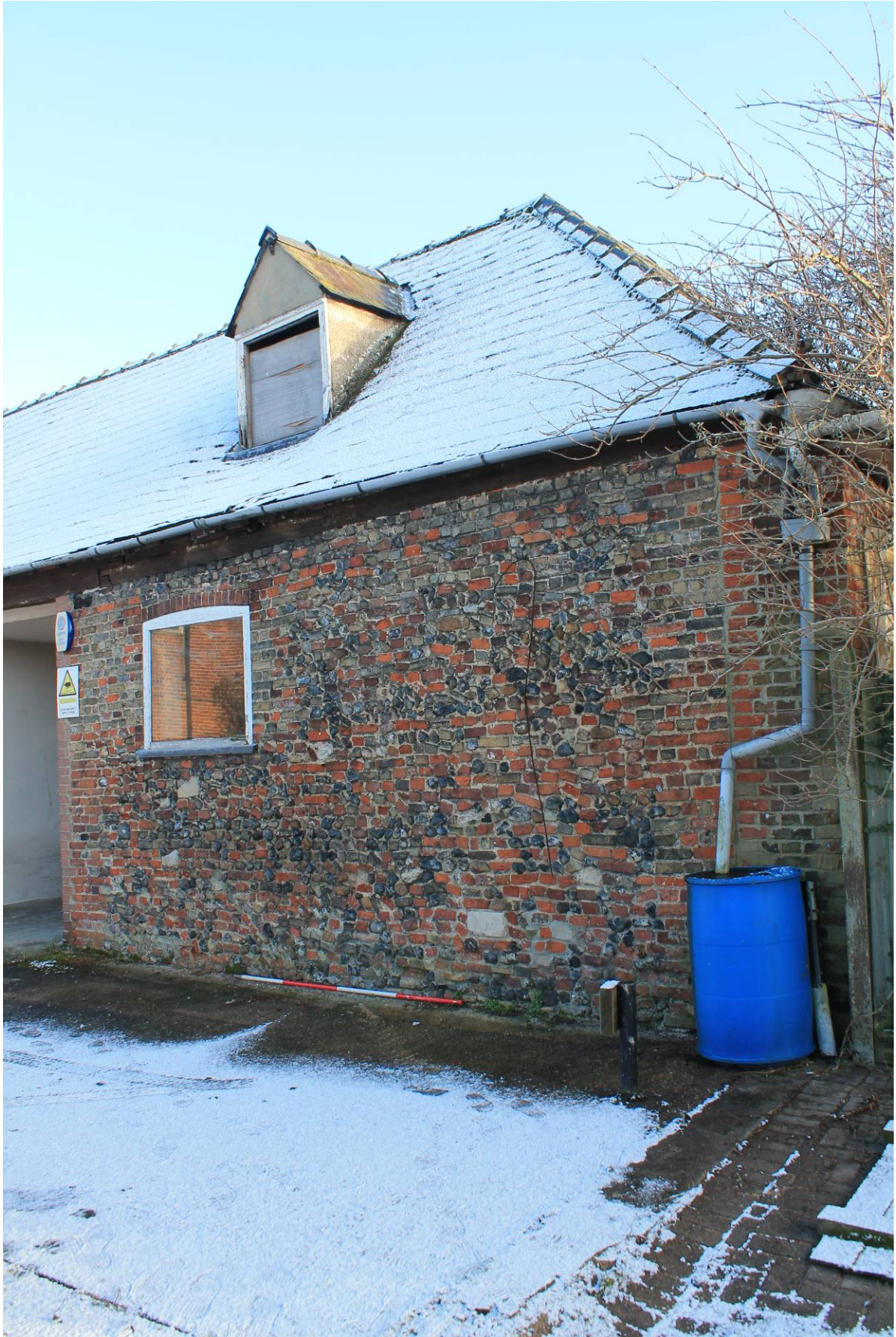
Plate 29 Stable (C) Western Elevation looking NE
