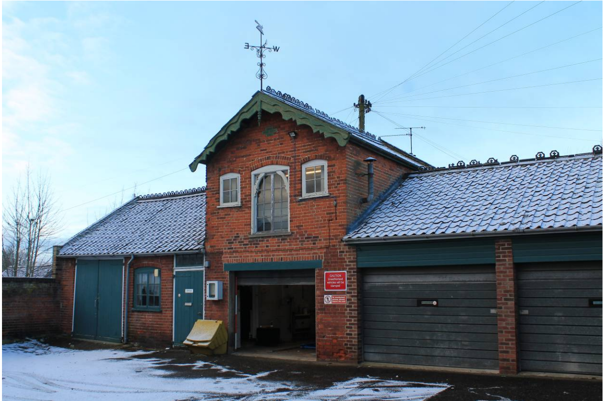
Plate 1 Stable Block (A) looking SW
