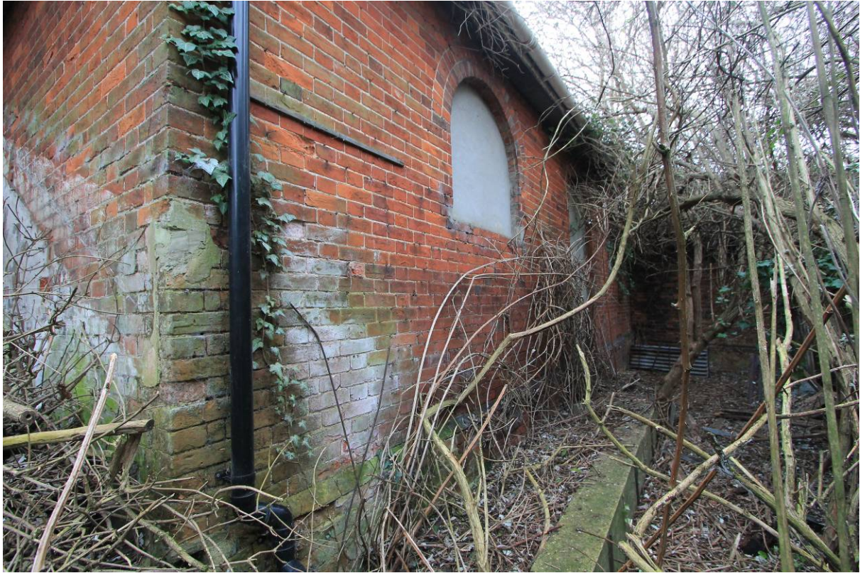
Plate 30 Stable (C) Southern Extension looking E
