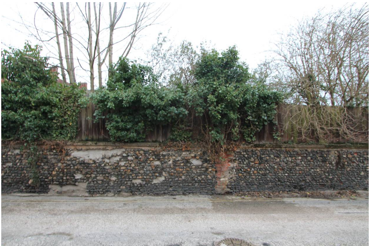
Plate 46 Friars Lane Boundary Wall, next section to south
