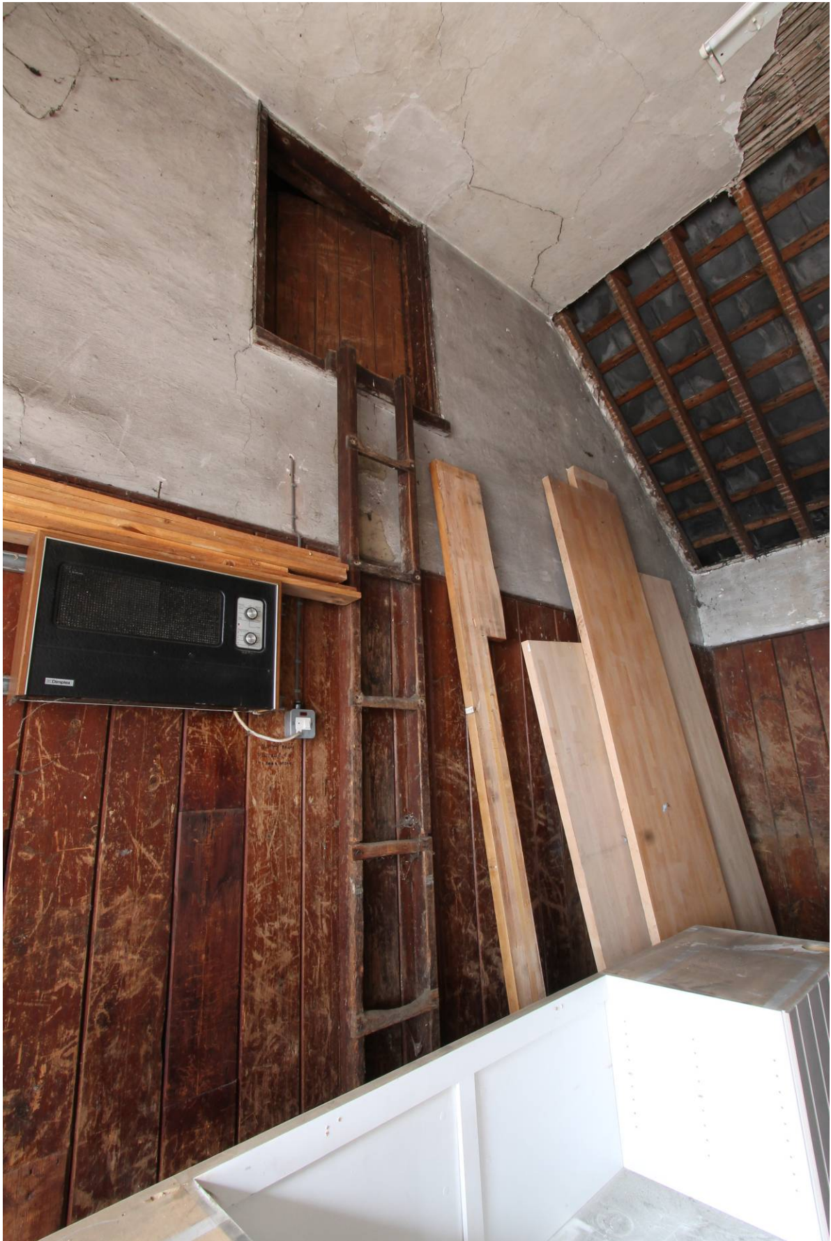
Plate 31 Former Stable (C6) looking SW
