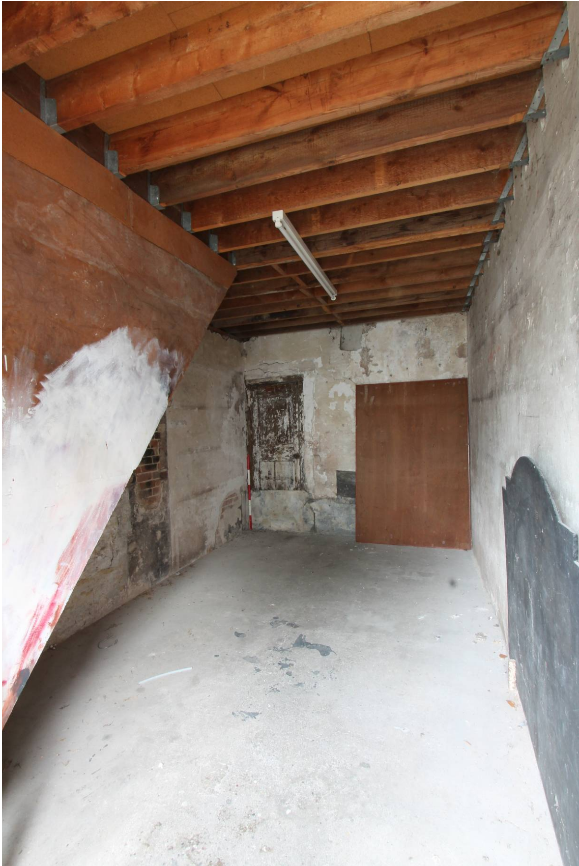
Plate 32 Former Tack Room (C5) looking W
