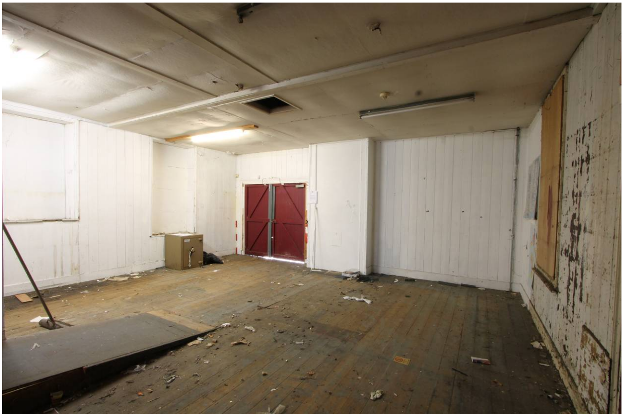
Plate 19 Building (B) looking SE
