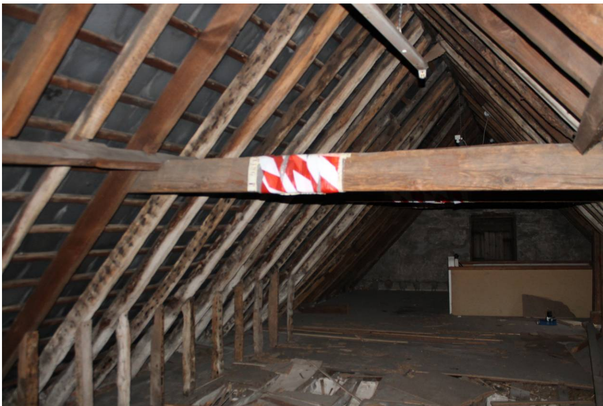
Plate 37 Stable (C) Side Purlin Roof over Hayloft
