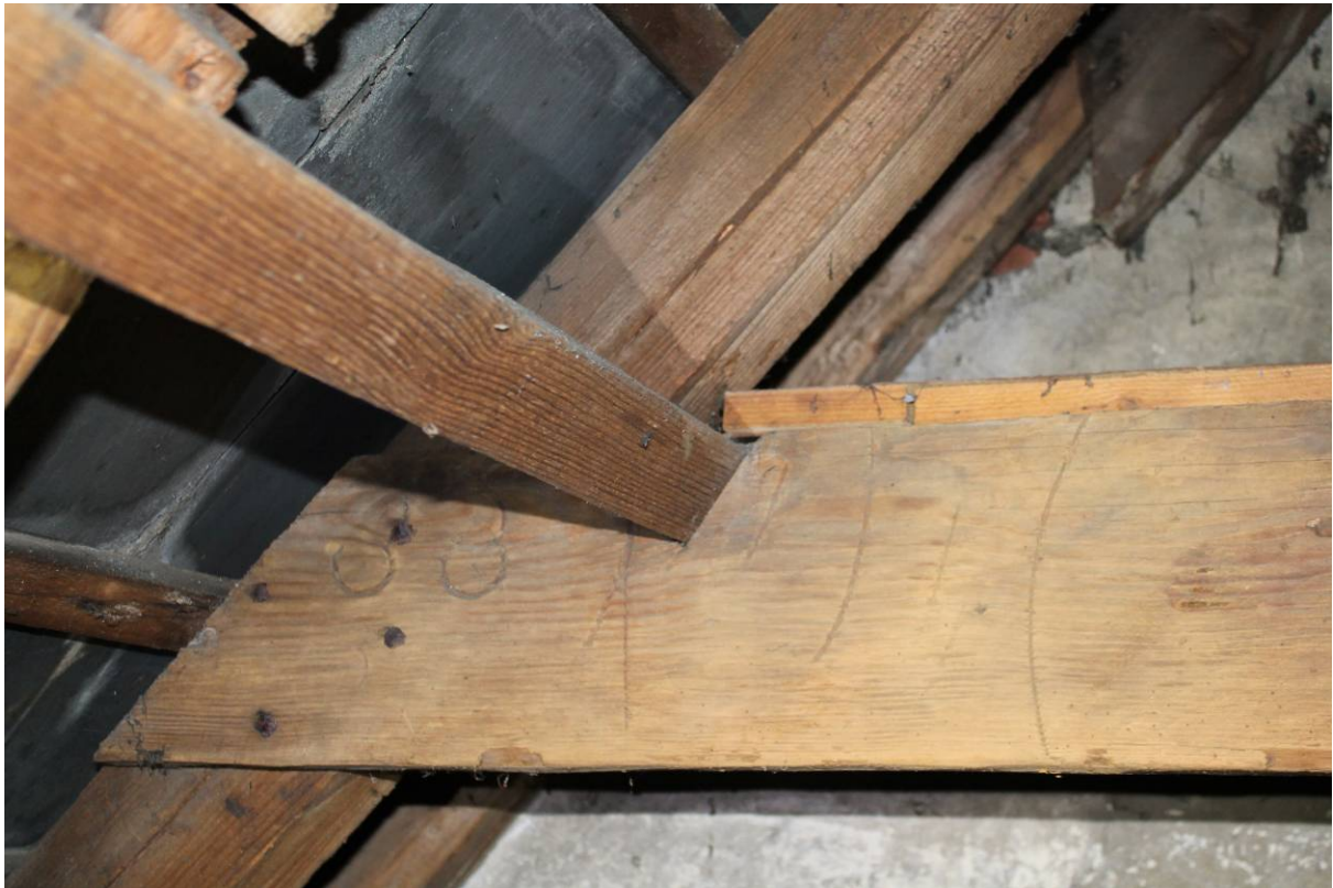
Plate 40 Baltic Marks on Collar in Hayloft, looking N
