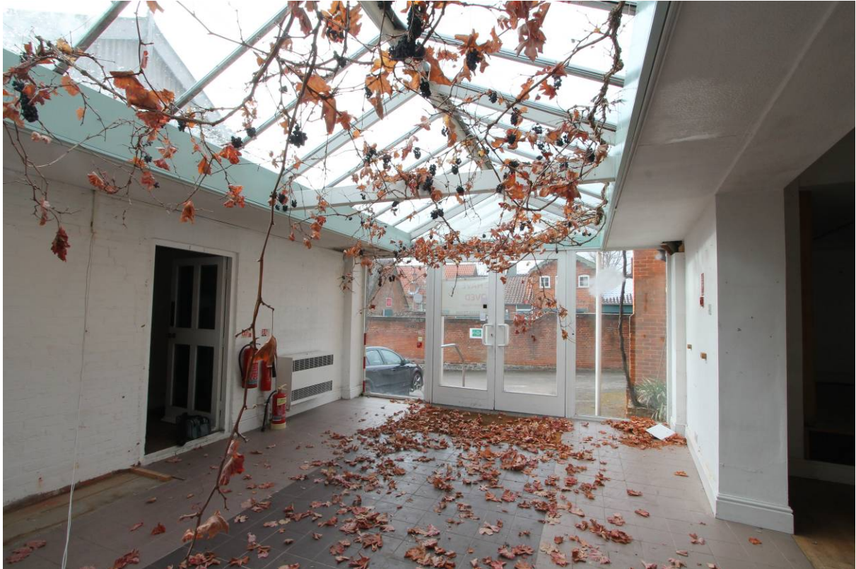
Plate 23 Entrance Foyer (B6) Looking W
