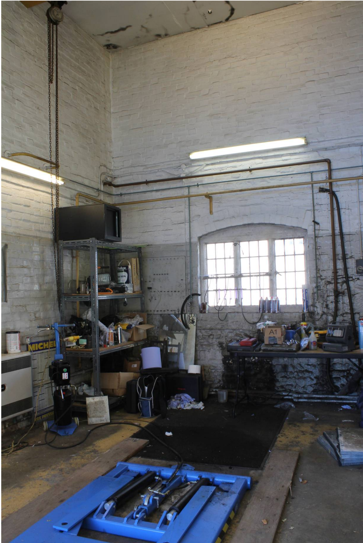
Plate 9 Stable (A) Workshop (A3) looking W
