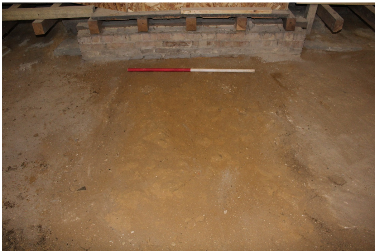
Plate 6: Demolition rubble (109) of dividing partition, view west
