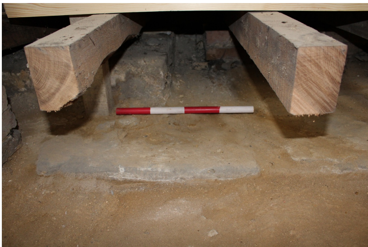
Plate 4: Foundation 105 and column base 115, view west
