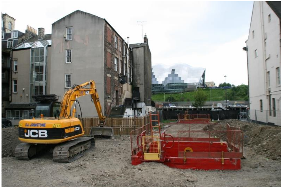
Plate 10. Trenches 1 (fore) and 2 (rear) with shoring installed, working shot; looking south-east
