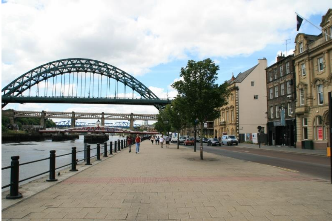
Plate 1. Overview of site location on the Newcastle Quayside; the site is the open space in the street frontage to the right; looking south-west
