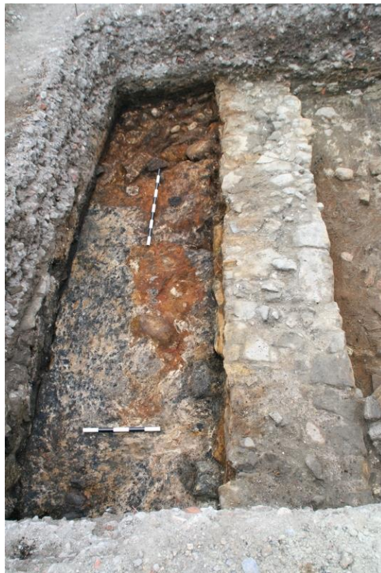
Plate 20. Trench 1 (prior to shoring installation), Phase 2 remains: wall [12] (original height); clay surface [21] (left, fore); looking north-west (1m and 0.5m scales)
