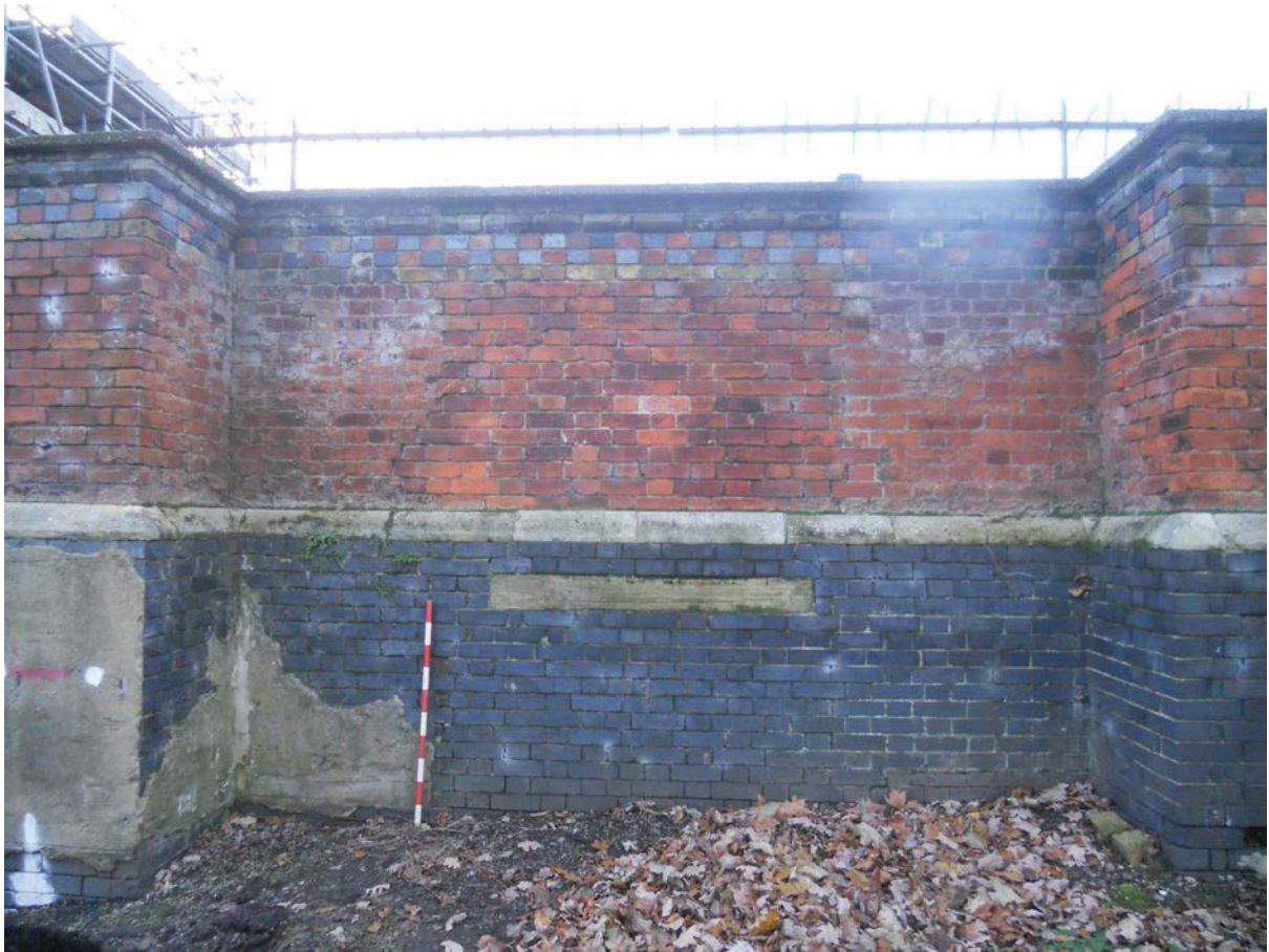
Plate 7: Blocked doorway in the north elevation of the church between buttresses 5 and 6, looking south
