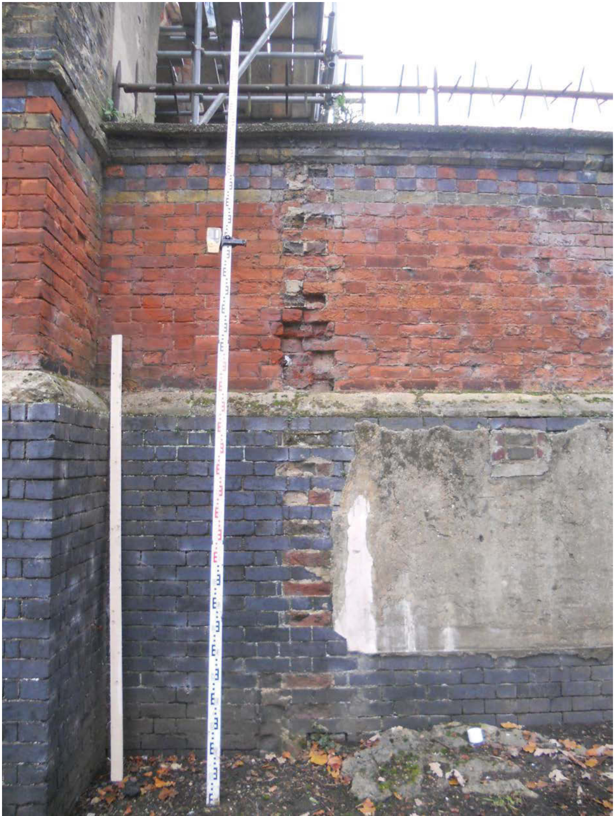
Plate 8: Wall scar in the north elevation of the church to the west of buttress 7 (right), looking south
