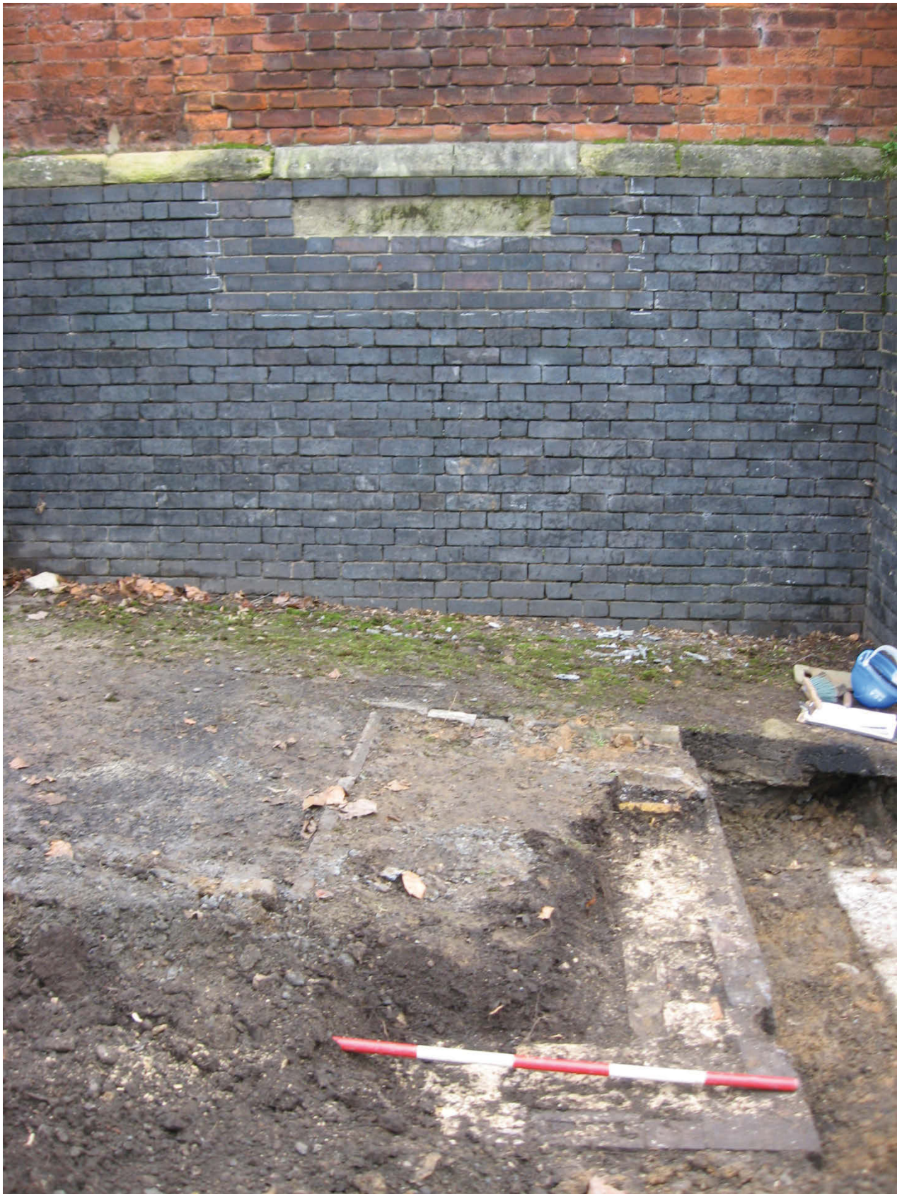
Plate 19: Blocked opening in the south elevation of the church to the north of wall 48, looking north
