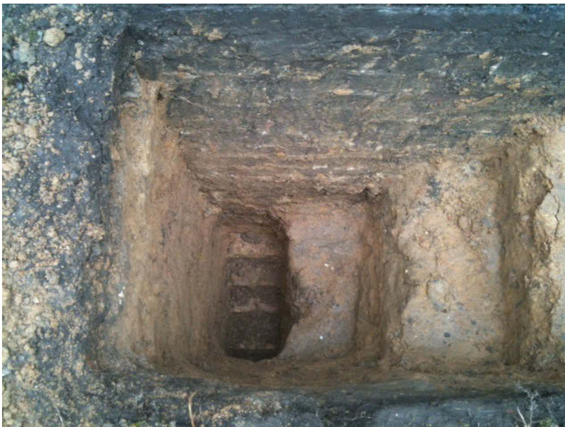
Plate 4: TP 1 Stepped foundations of the south elevation of the Garrison Church of St George, looking north
