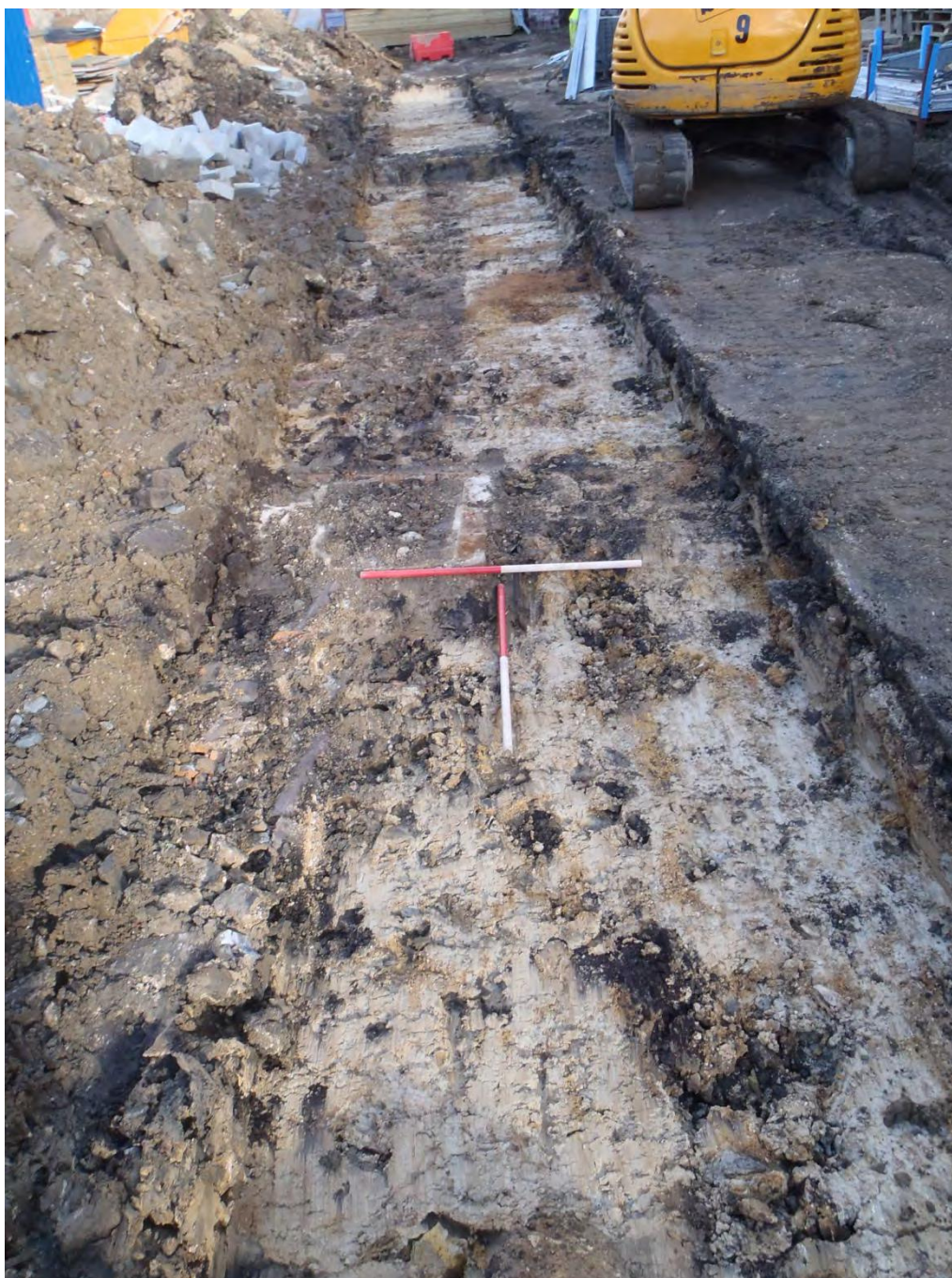
Plate 3: Trench 3, view east
