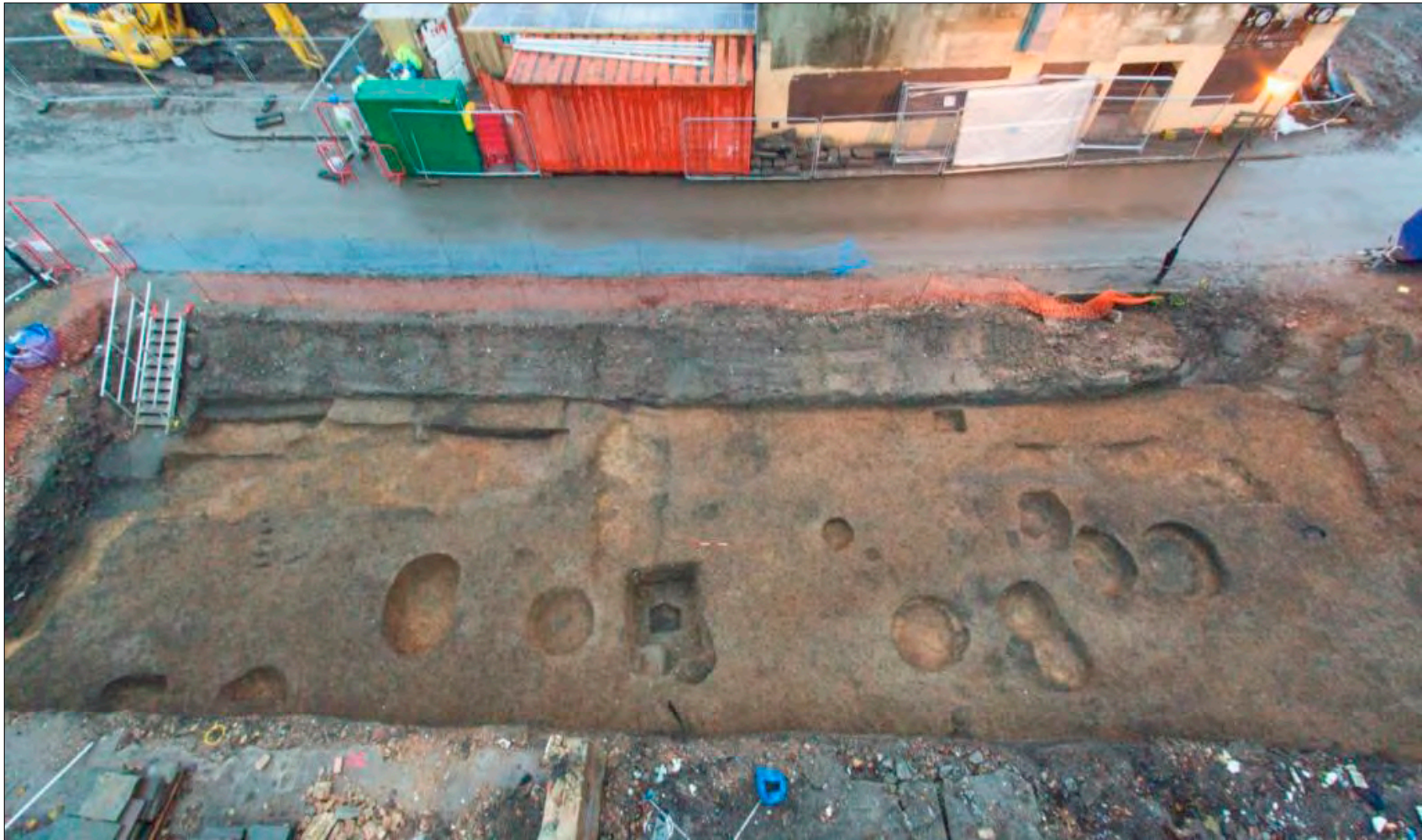
Plate 1: The Excavation Area, Looking North
