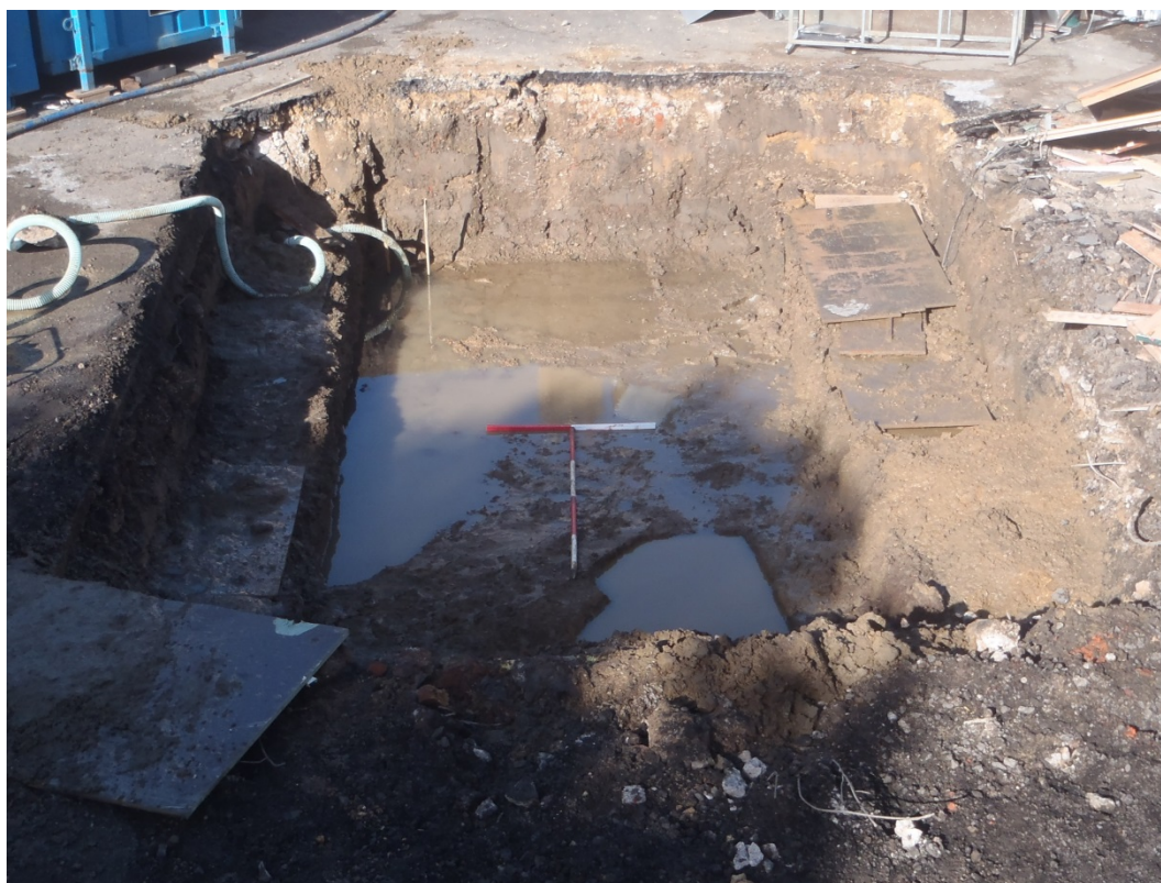
Plate 1: Trench 2, view north-west
