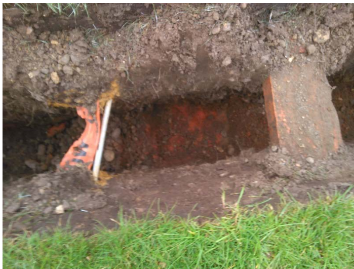
Plate 8: Truncated wall [7] and location of modern security cables
