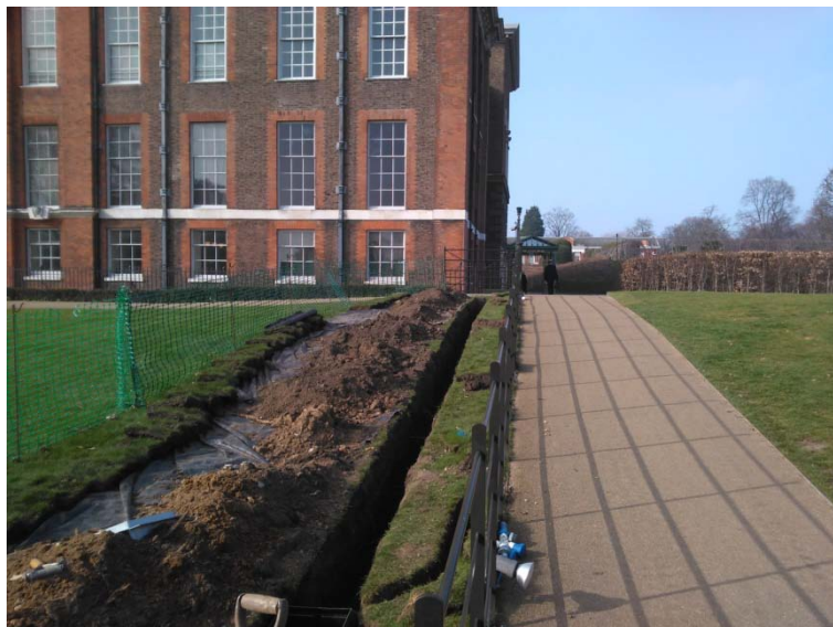
Plate 3: Northern length of cable trench –view north
