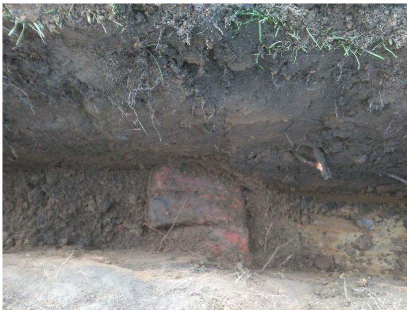
Plate 10 West view of wall [12]
