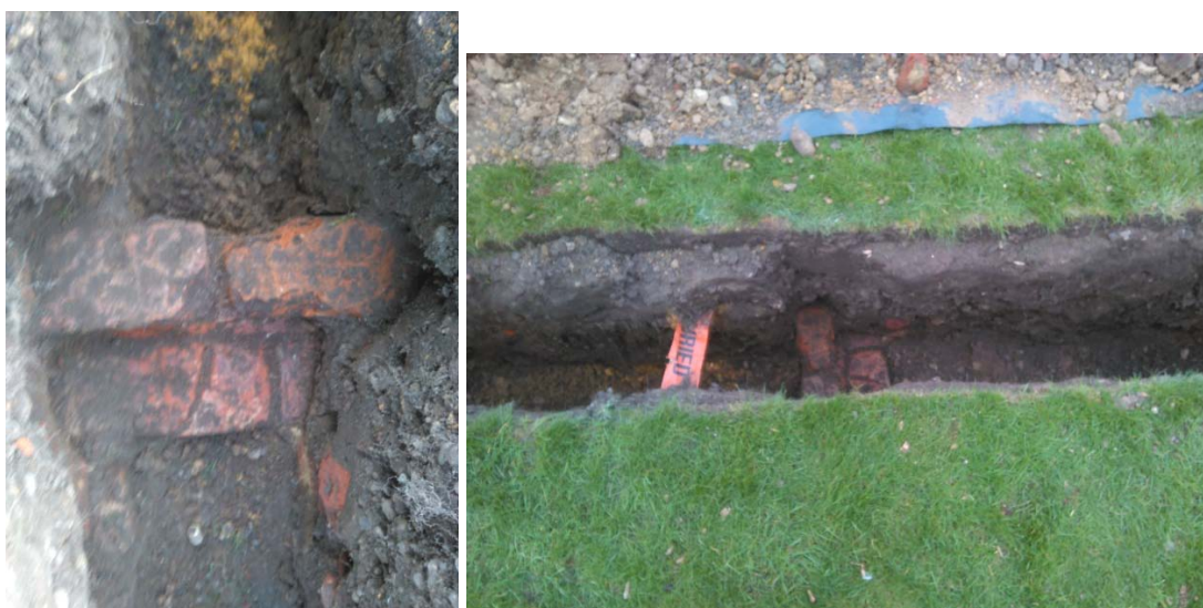
Plates 6 and 7: South and west views of wall [6]
