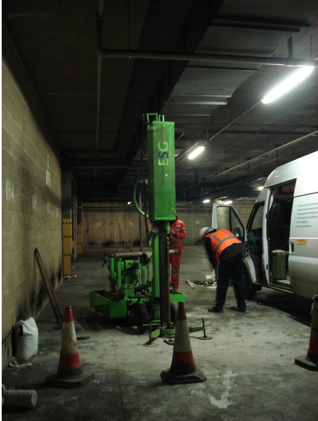
Plate 3: Environs of Window Sample 9, from the east facing west
