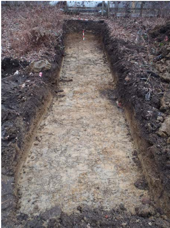
Plate 1. Trench 1, looking North. Scales 2m x 0.4m
