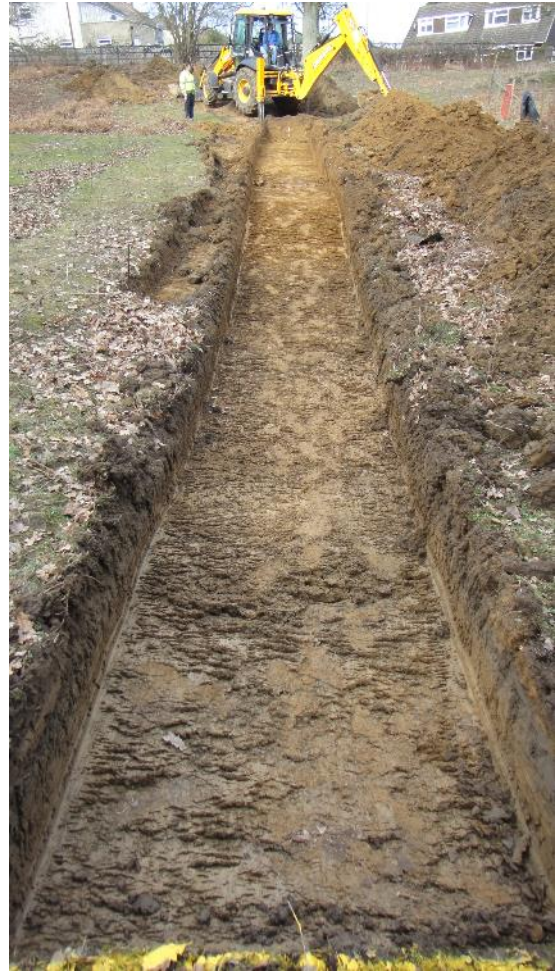
Plate 8. Trench 3, looking North. Scales 2 x 0.4m
