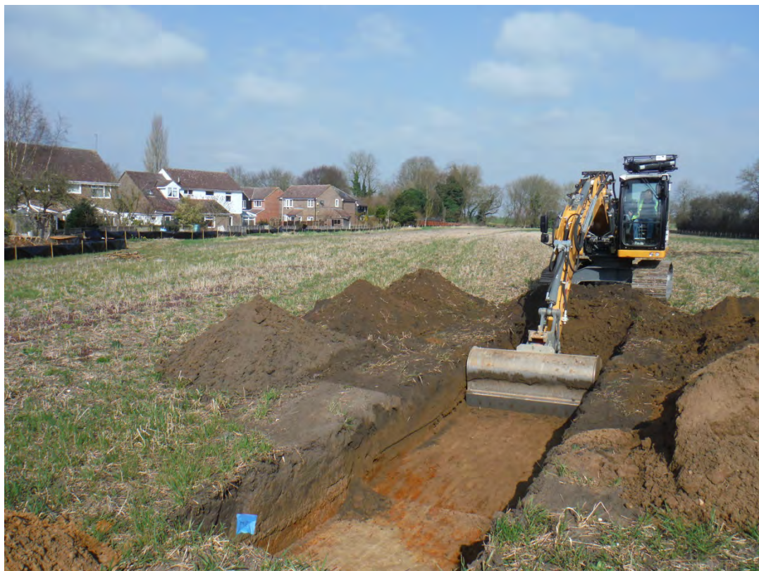
Plate 2: Machining, view north-west
