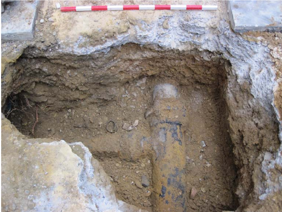
Plate 3: Trench 2A facing east, scale 1m
