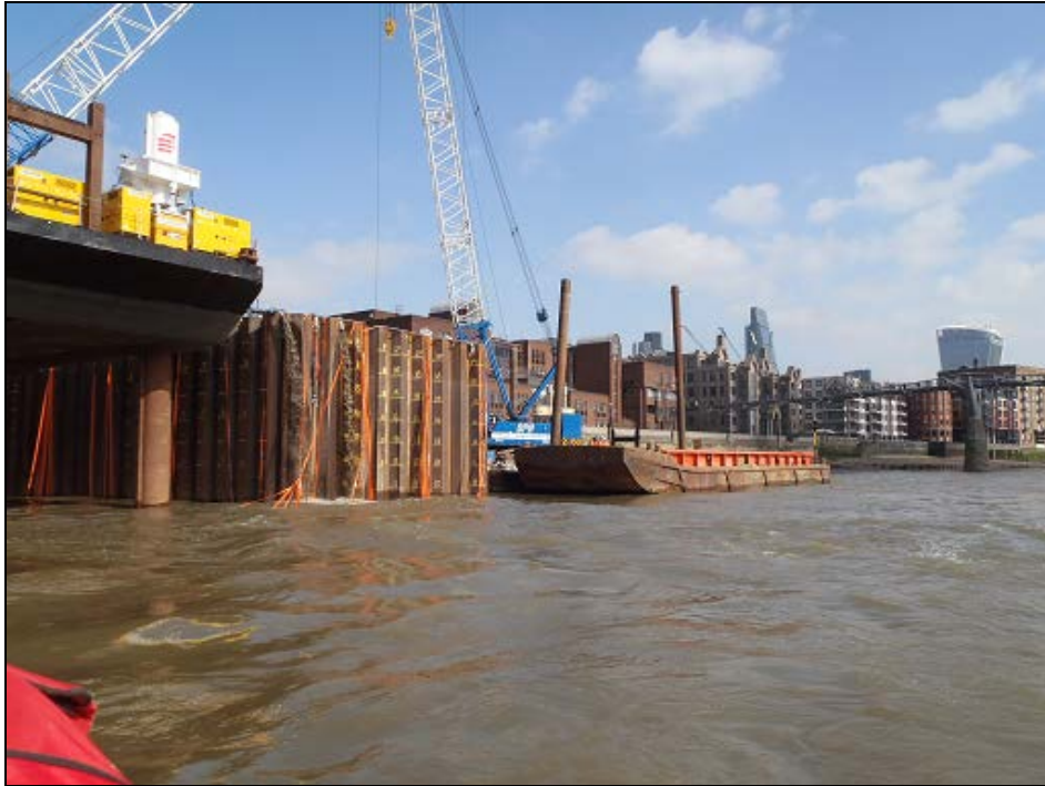
Plate 1: North-east facing shot of coffer dam with associated barge to east
