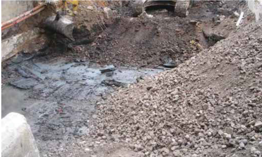
Plate 4: Ground reduction exposing upper Alluvium [55]. Looking SE.
