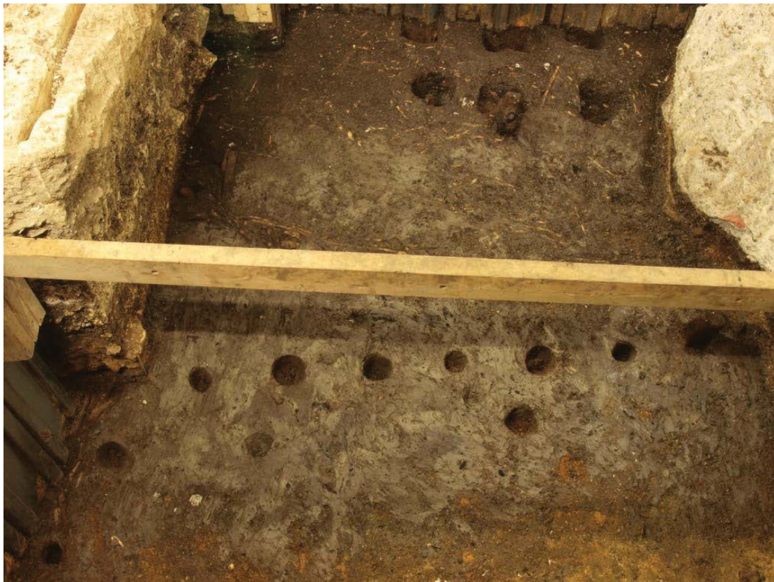
Plate 3: Waterfront 2. Demolished post and plank revetment
