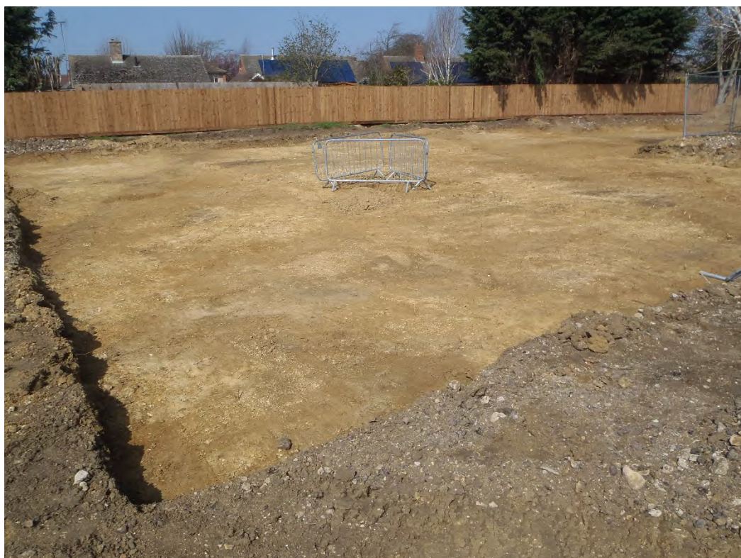
Plate 4: Excavation area, view north-west
