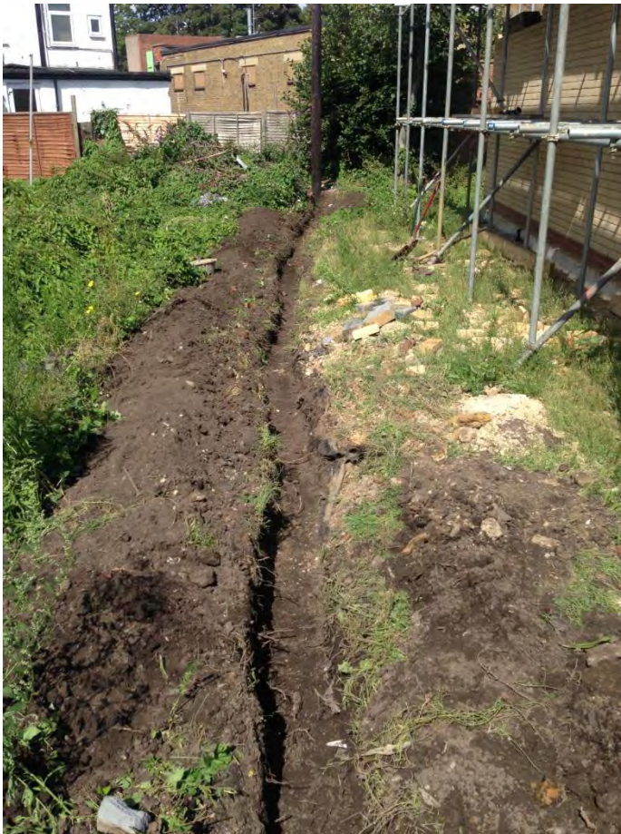
Plate 4 – Trench 2 looking north to the new telegraph pole (Trench 1). Note concrete raft to the right.
