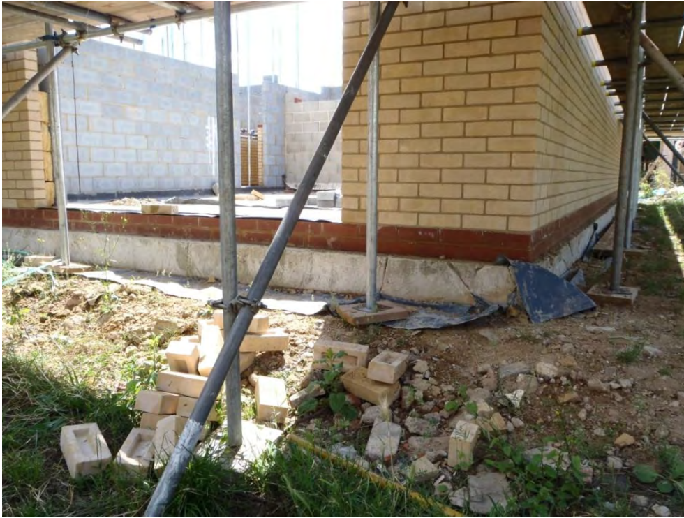
Plate 1 – View showing the nature of the non-intrusive concrete raft, on which the houses were constructed. Landscaping will include the importing of soil to build up the level of the site to the top of the raft.
