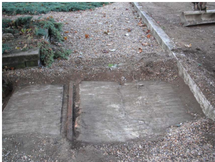
Plate 7: Travelling crane rail [6] set in concrete in Trench 6, view northwest
