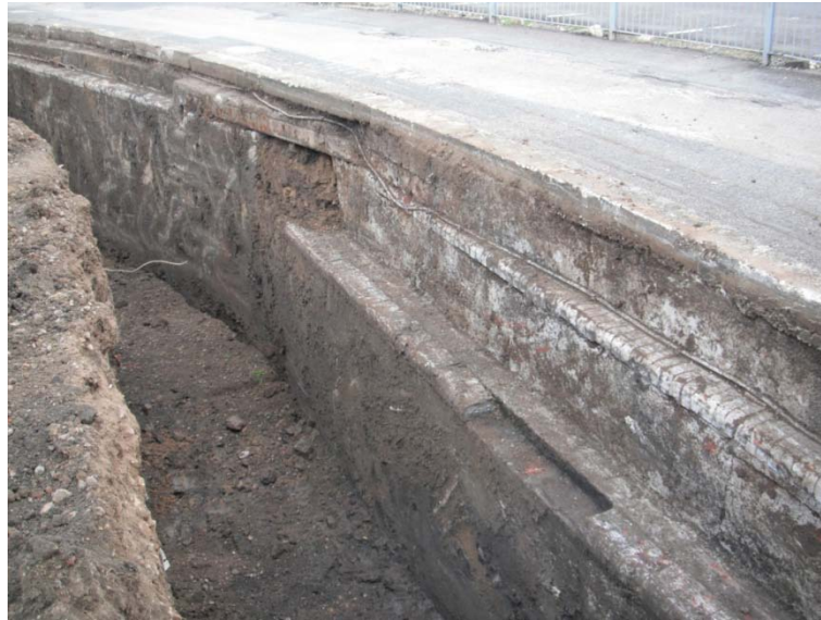
Plate 4: Extended dock wall [1] in Trench 2, view north
