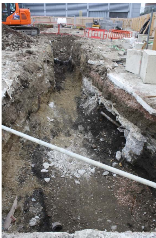
Plate 1: Made ground deposit [3] within Trench 8, view SE
