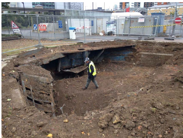
Plate 9: Staircase structure [5], view northeast
