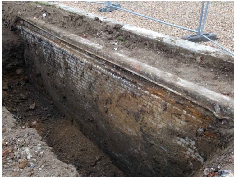
Plate 3: Extended dock wall [1] in Trench 1, view southwest
