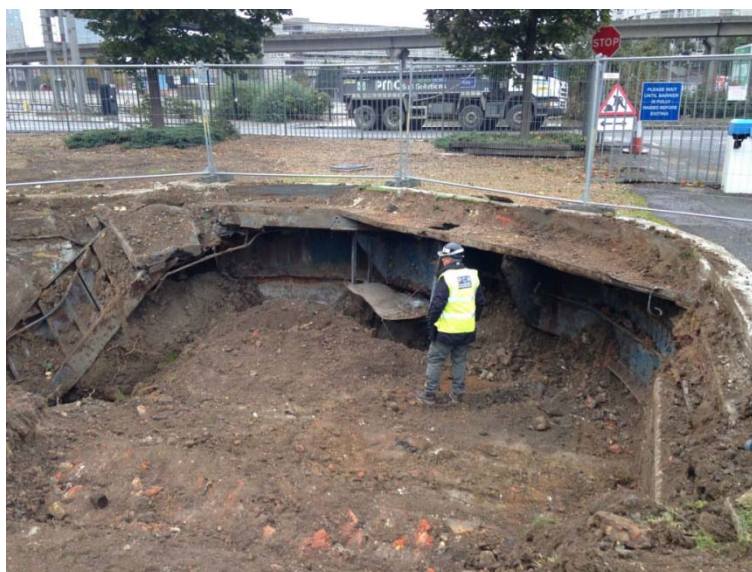
Plate 8: Staircase structure [5], view north
