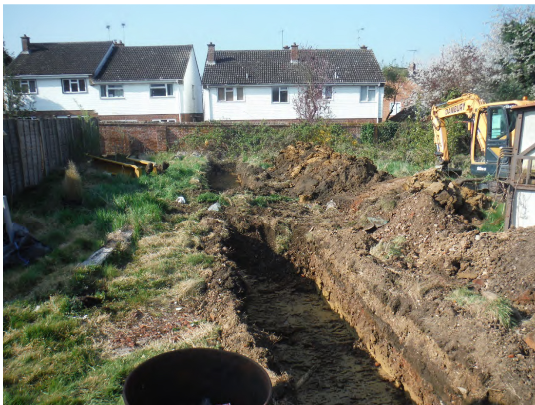
Plate 1: Trench 1, view west across site
