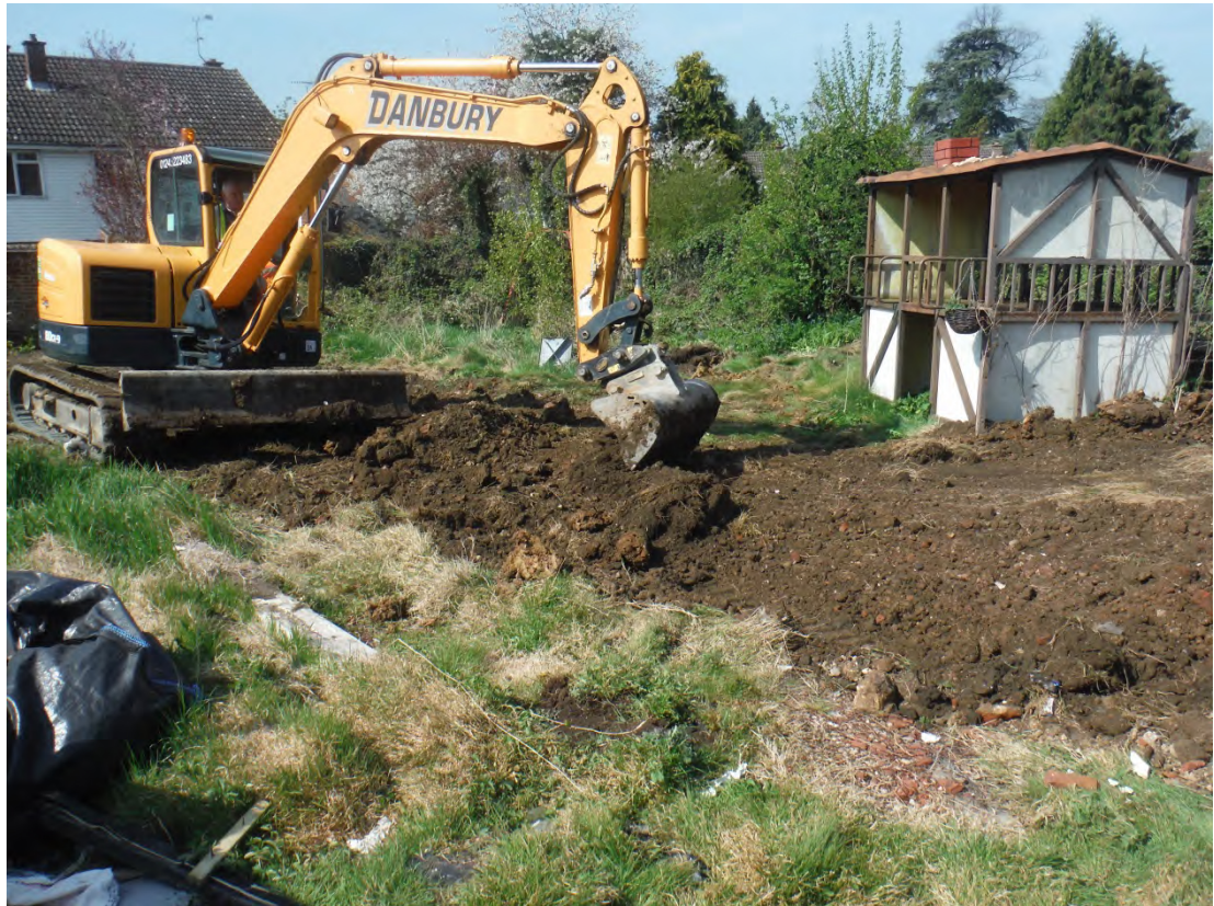
Plate 5: North-western view of Backfilling Trenches 1 & 2
