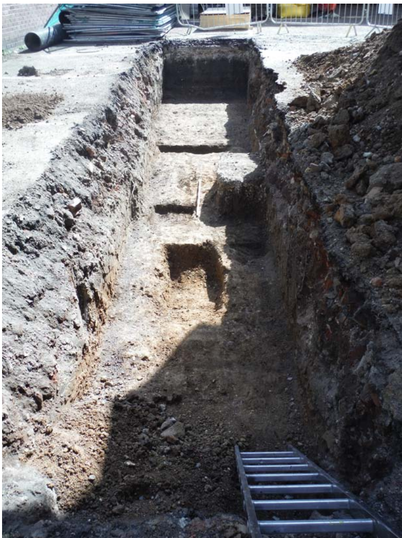
Plate 3 – South facing view of Trench 5 (1m scale)
