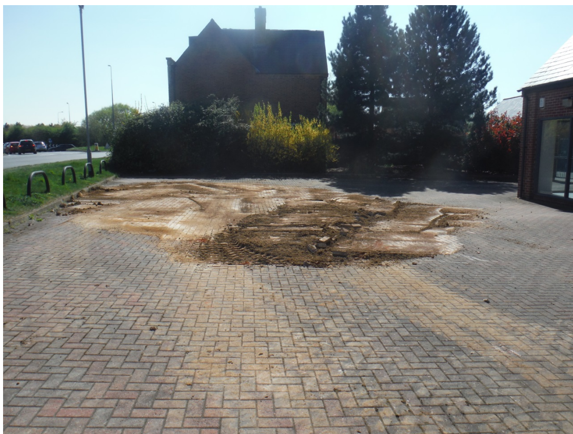
Plate 10: Trench 2, S facing view following reinstatement
