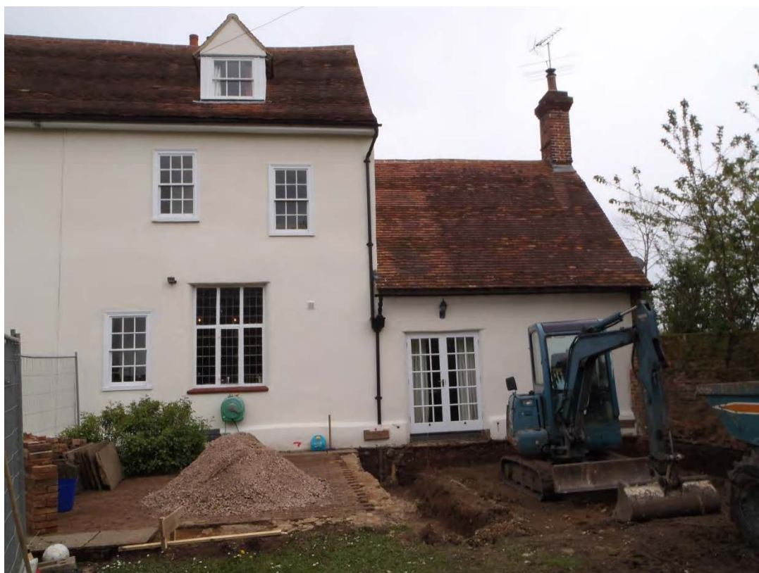
Plate 1: The site, view south-east
