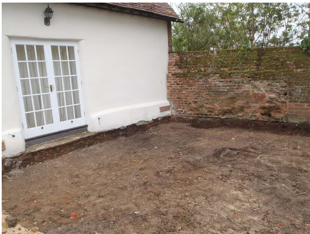
Plate 2: After initial ground reduction, view south
