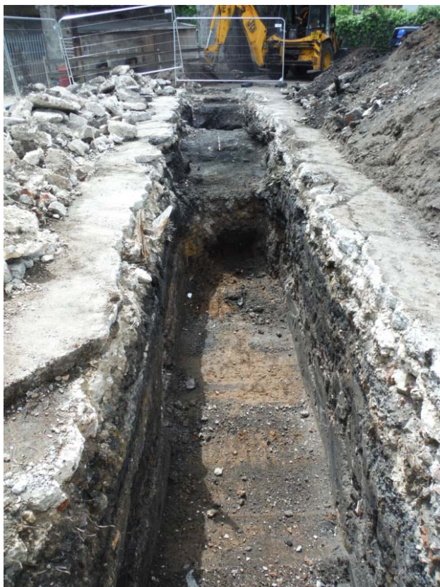
Plate 1: Trench 1, looking south-west
