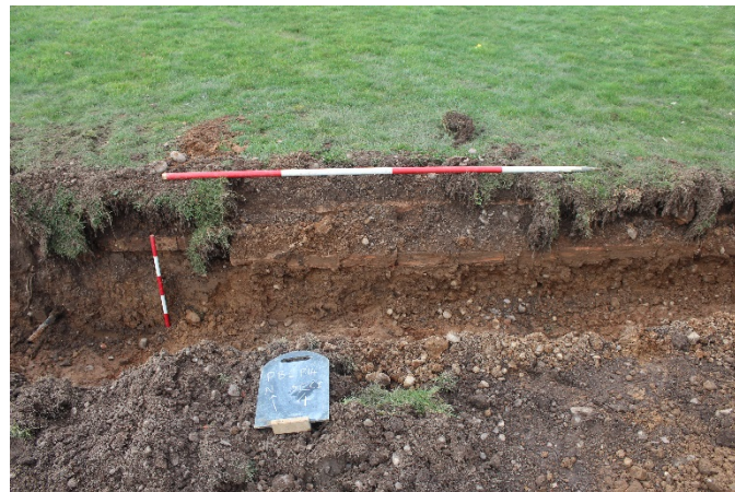
Plate 6. South-facing section of foundation trench for garden wall (Section 4). Scales 1 x 2m; 1 x 1m.
