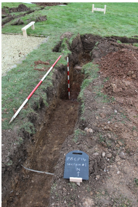
Plate 1. East-facing section of foundation trench for garage (Section 1). Scales 1 x 2m; 1 x 1m.
