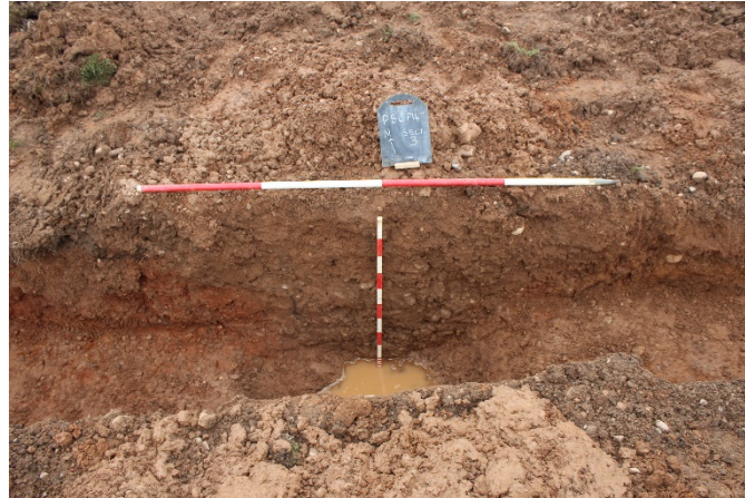
Plate 5. North-facing section of foundation trench for garden wall (Section 3). Scales 1 x 2m; 1 x 1m.
