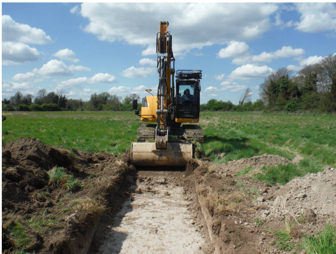
Plate 3: Trench 29, north-west facing view of Machining
