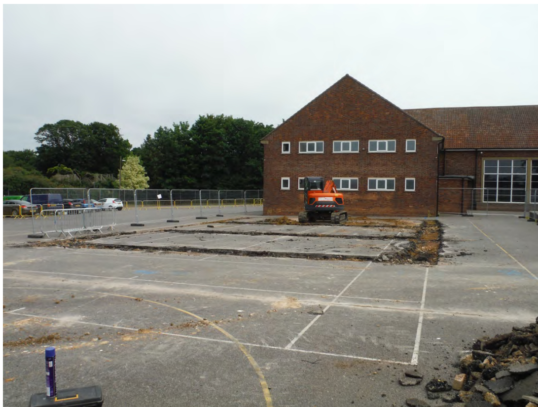
Plate 3: Area 3, view north-west
