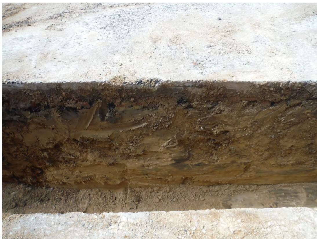
Plate 4: Area 3 foundation, view south
