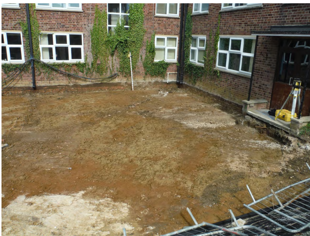
Plate 2: Area 2, view north-west
