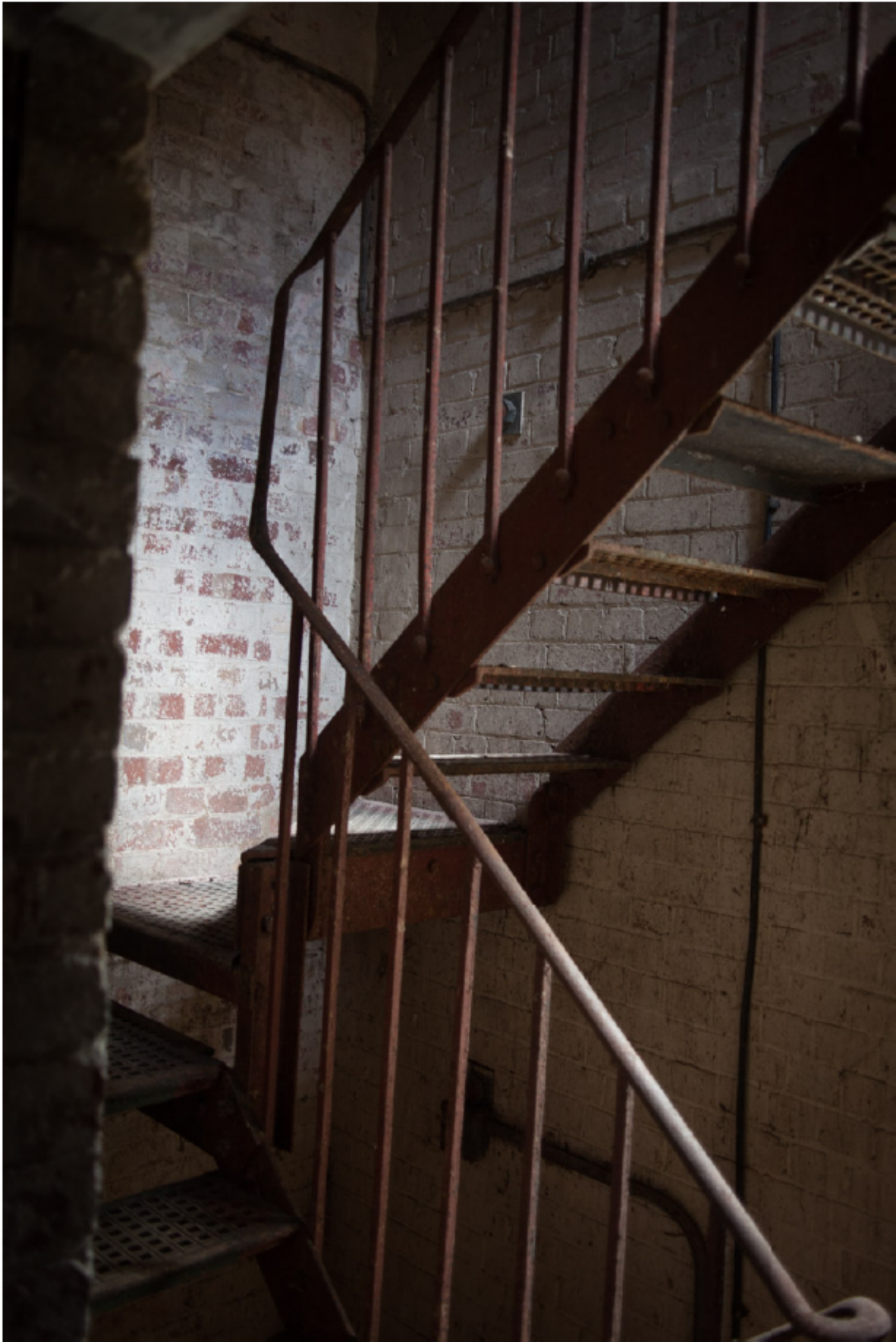
Plate 38 Rear fire escape stairs 2.03 and access to second floor, looking south-east
