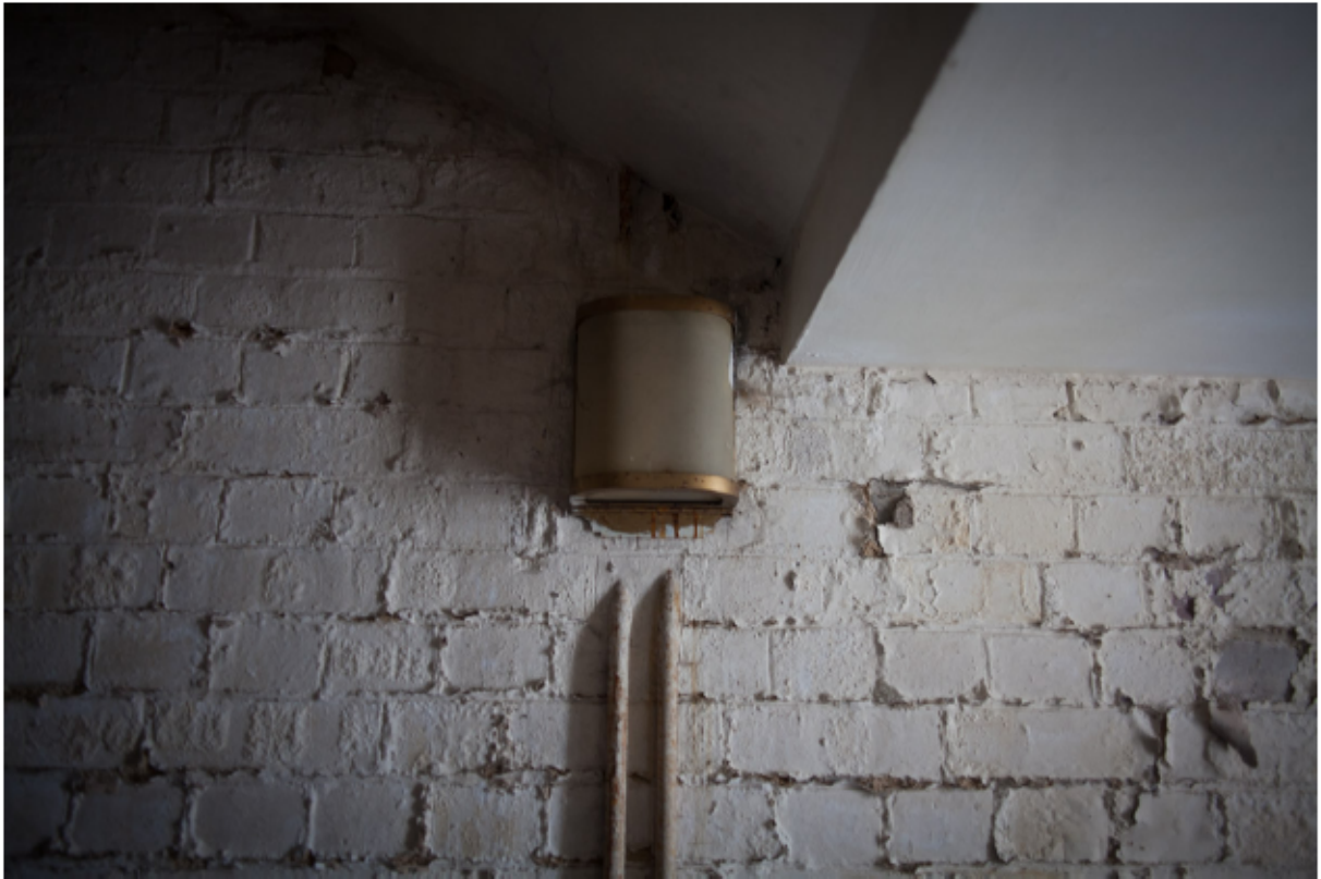
Plate 33 Original glass light fitting in stairwell 2.08, looking south
