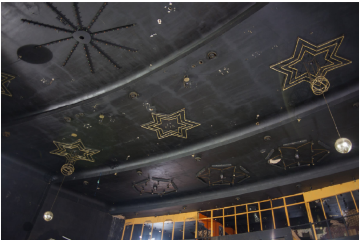
Plate 25 Ceiling with modern light fittings over circle 2.01, looking south
