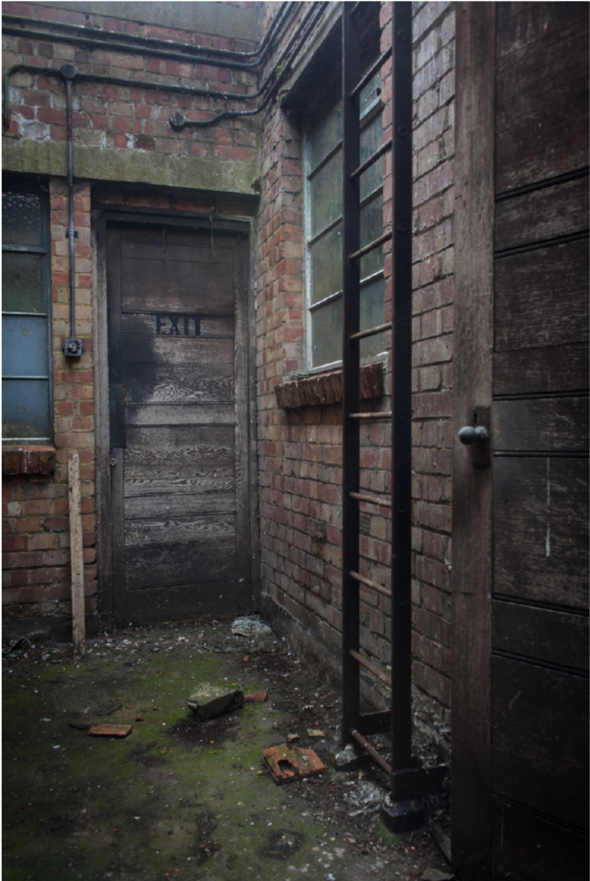
Plate 44 Open well 3.07 and fixed ladder to flat roof, looking west
