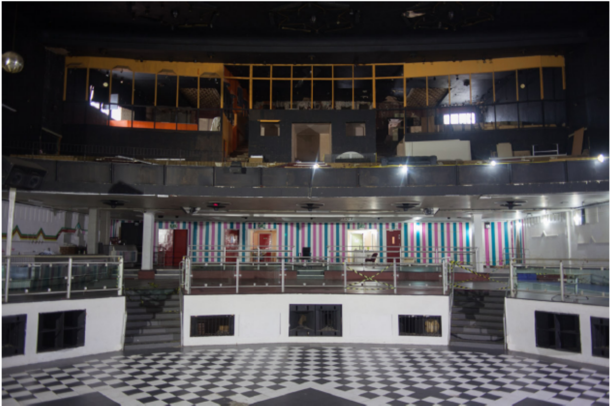
Plate 15 Upper tier of auditorium G.13 and circle 2.01, looking south
