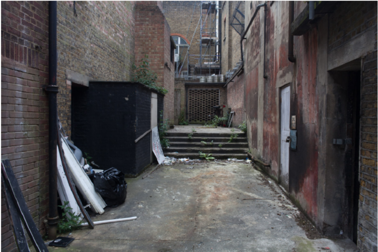
Plate 7 Rear service yard, looking west towards the Town Hall
