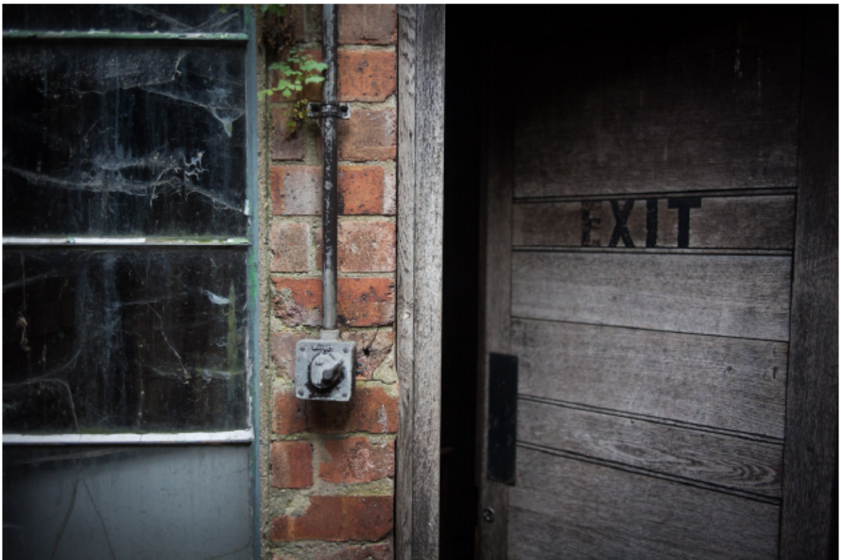
Plate 43 Original oak door to rewinding room 3.05, looking east
