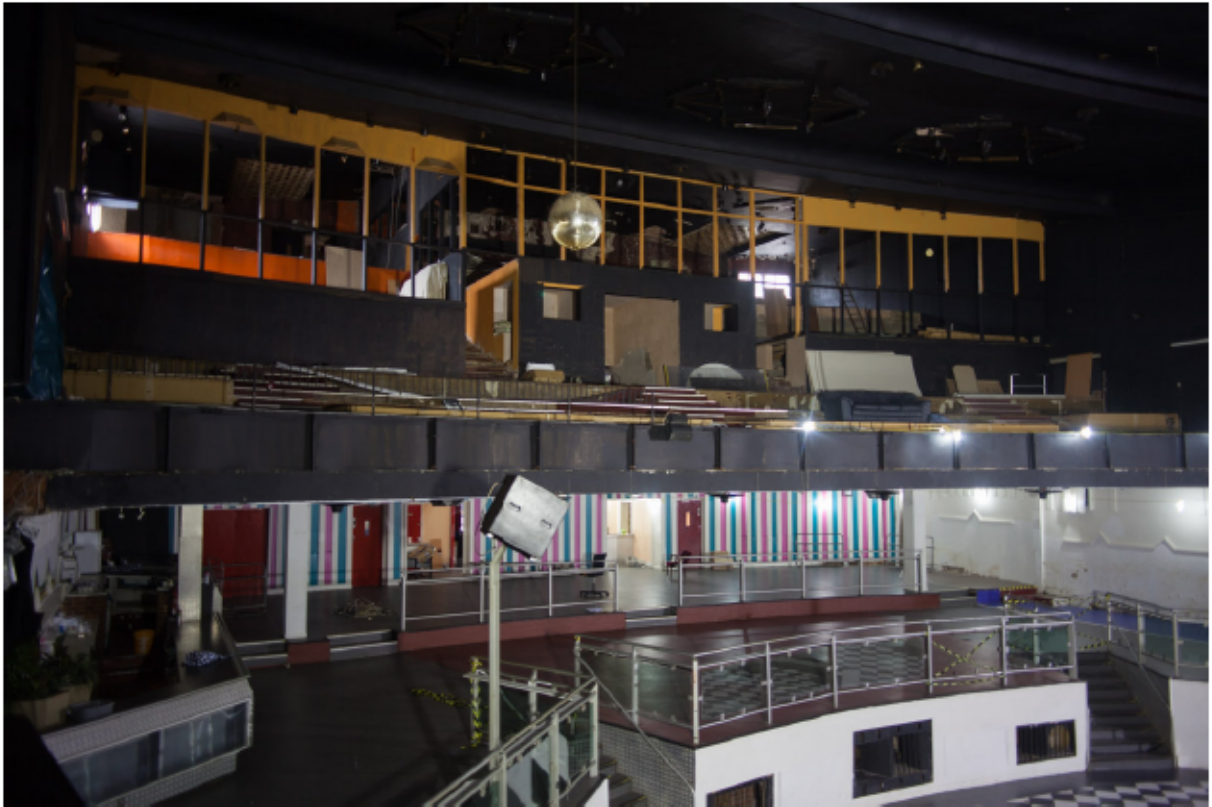
Plate 24 Circle 2.01, looking south-west from lower tier of auditorium G.12
