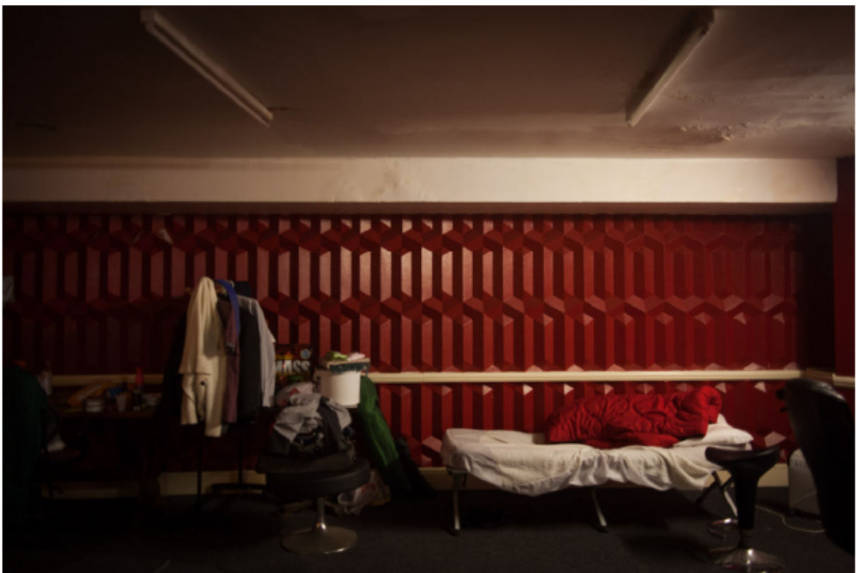
Plate 18 South wall to circle foyer 1.12 formerly open to the vestibule (G.26) below, looking south
