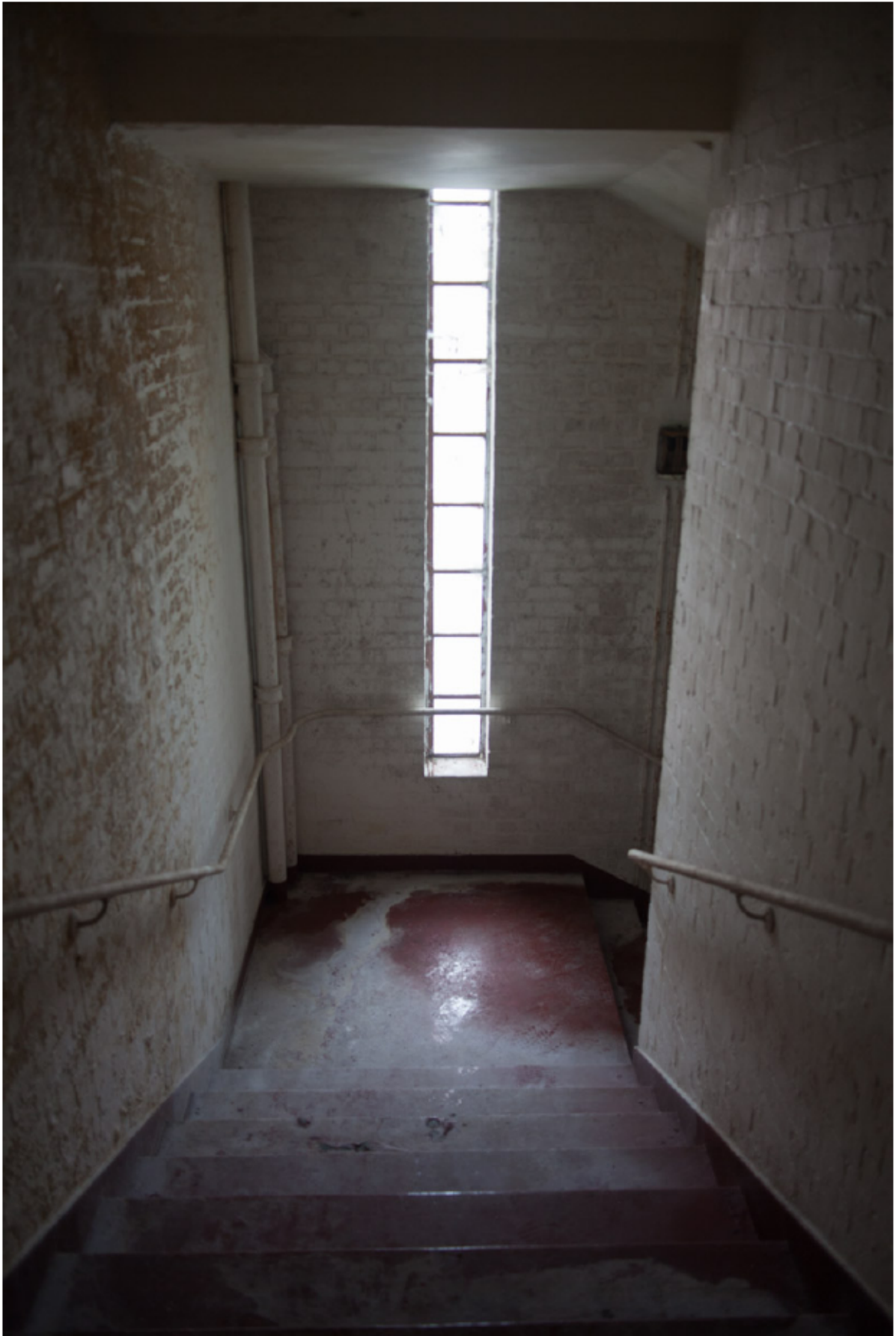
Plate 32 Exit stairwell 2.08 from circle 2.01, looking east
