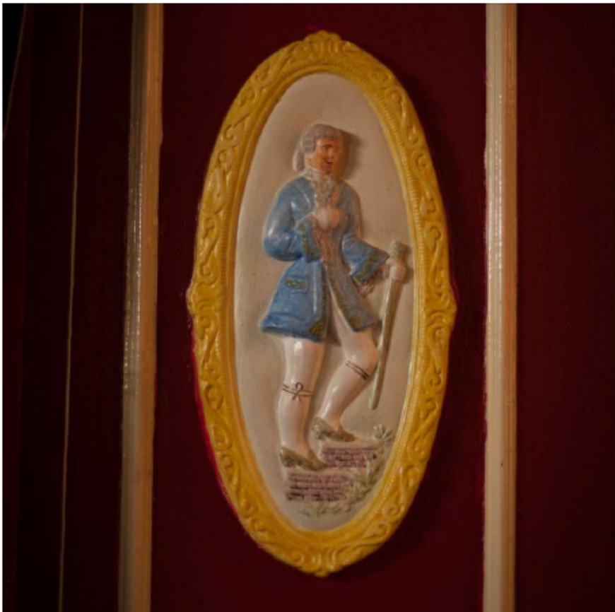
Plate 21 Ornamental plasterwork cartouches in circle foyer 1.12, presumably re-used from the previous theatre on the site, looking north
