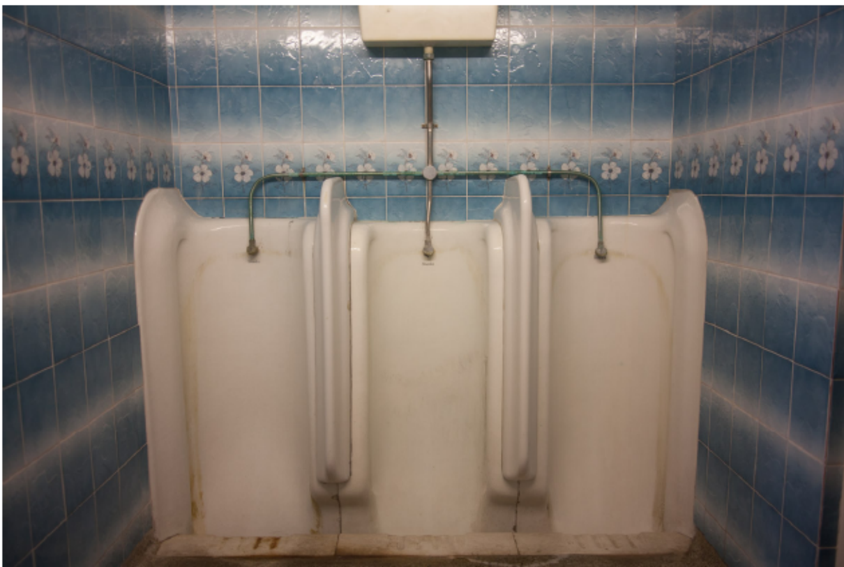
Plate 23 Original urinals within Gents toilets 1.09 accessed from circle foyer 1.12, looking south
