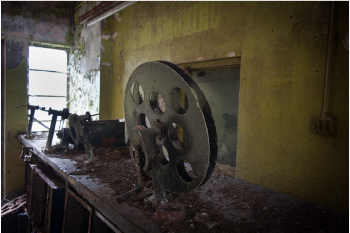
Plate 42 Rewinding room 3.05, looking west
