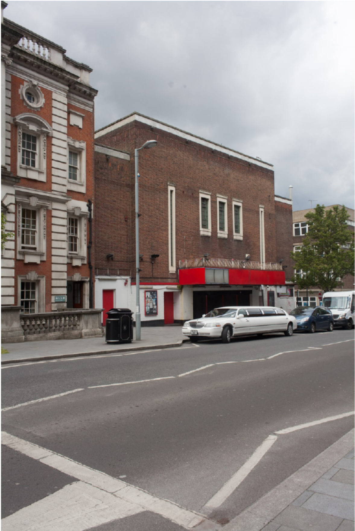
Plate 1 Woolwich Grand Theatre facade to Wellington Street, looking north-east
