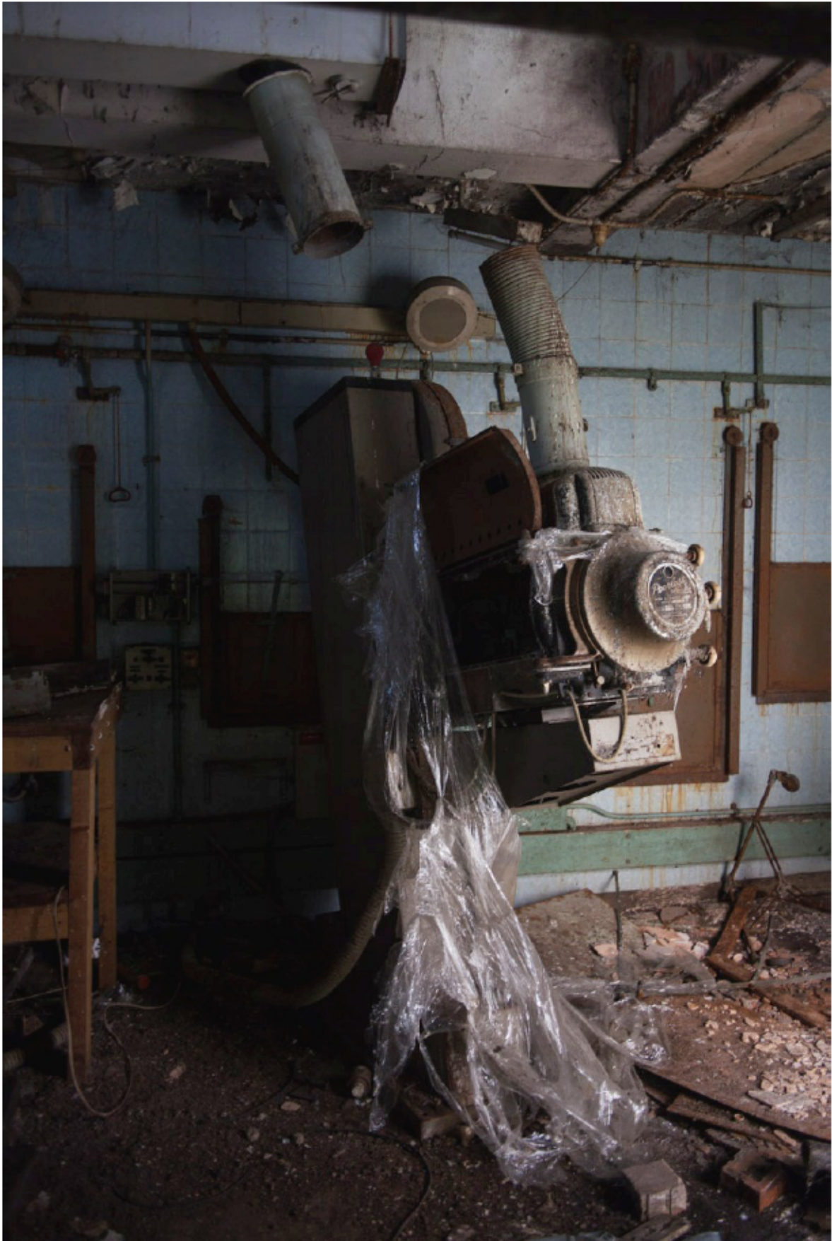
Plate 41 Detail of projector in projection room 3.04, looking north
