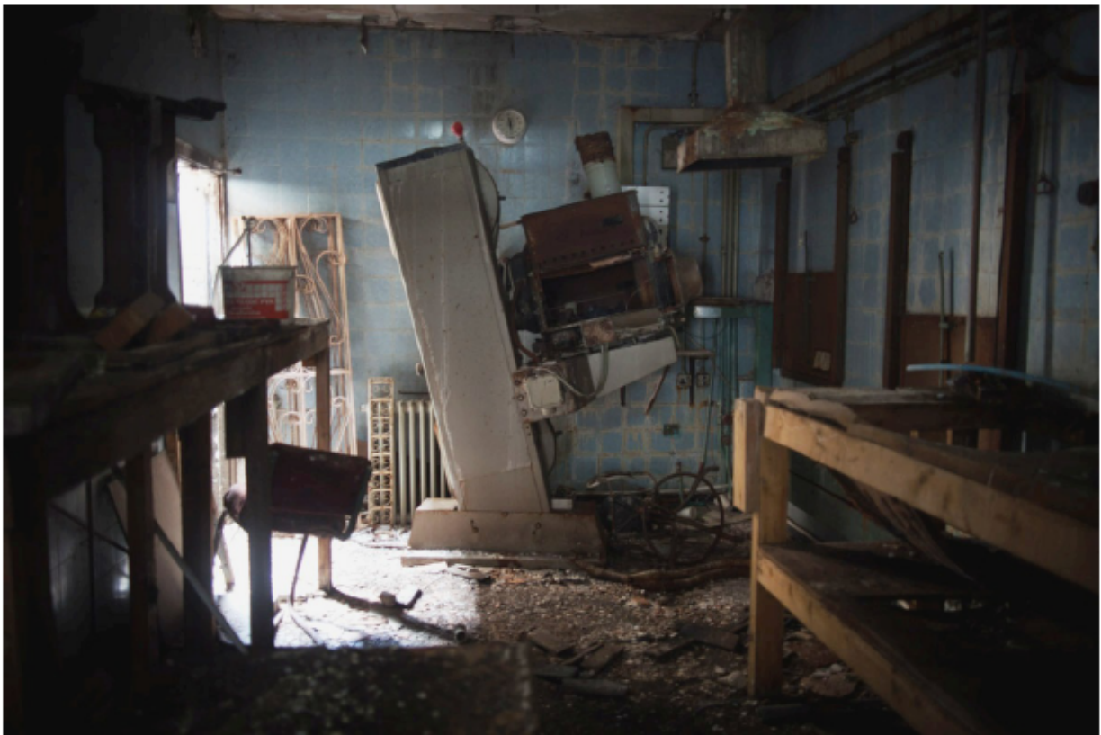
Plate 40 Projection room 3.04, looking west
