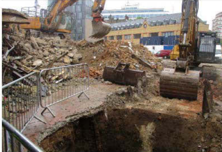
Plate 1: Trench 1 under excavation, view east
