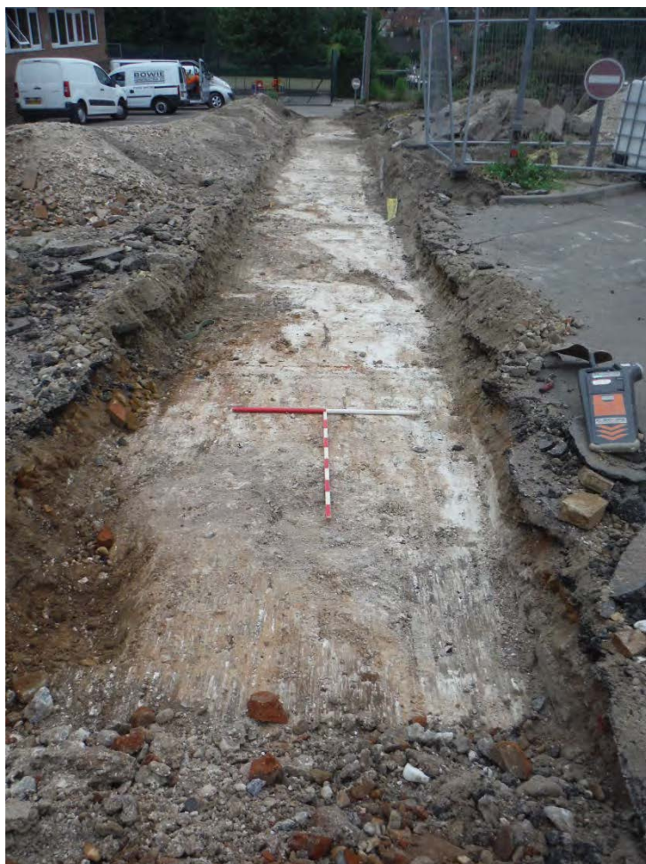
Plate 7: Trench 5, view south
