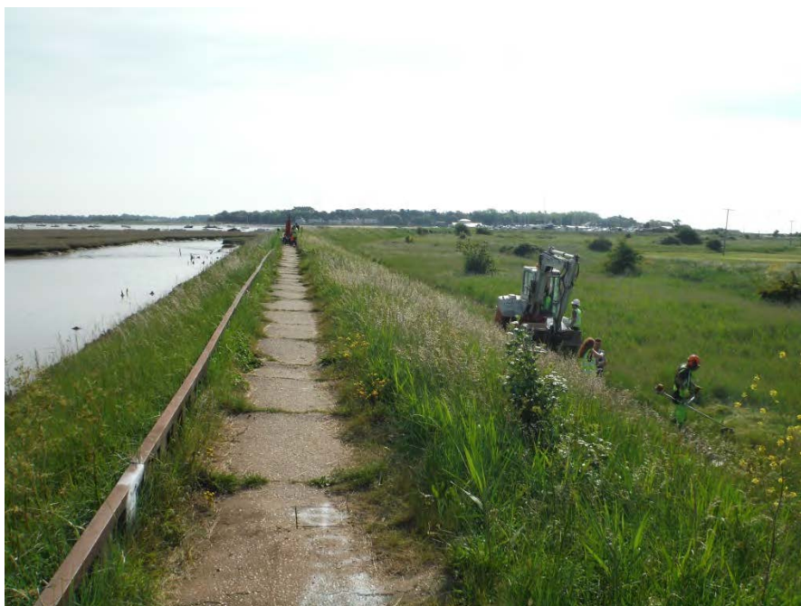
Plate 1: Felixstowe Ferry flood defences, view north-east
