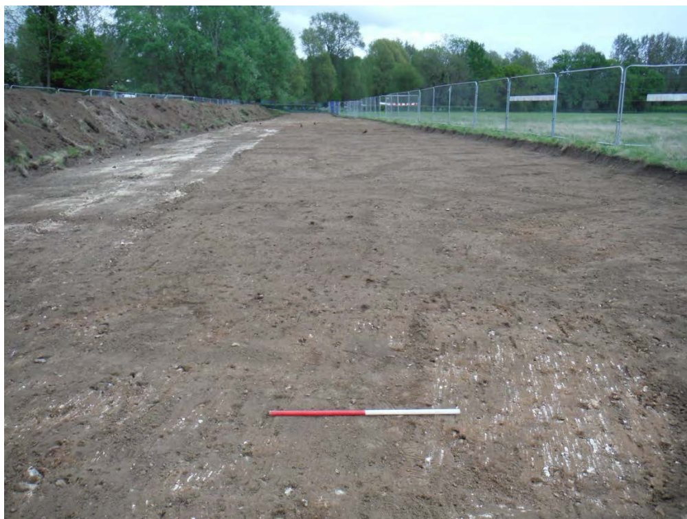
Plate 4: Pipe easement in field D, view east
