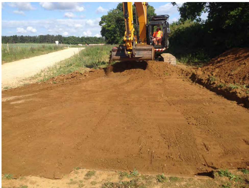
Plate 1: Pipe easement in field A, view north-west
