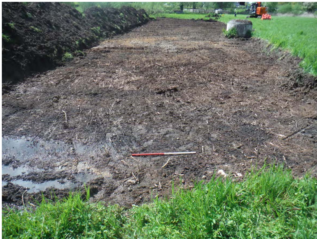
Plate 5: Pipe easement in field E, view east
