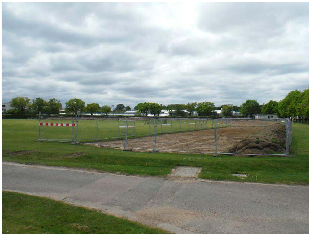
Plate 6: Pipe easement in field C after monitoring finished, view south-west
