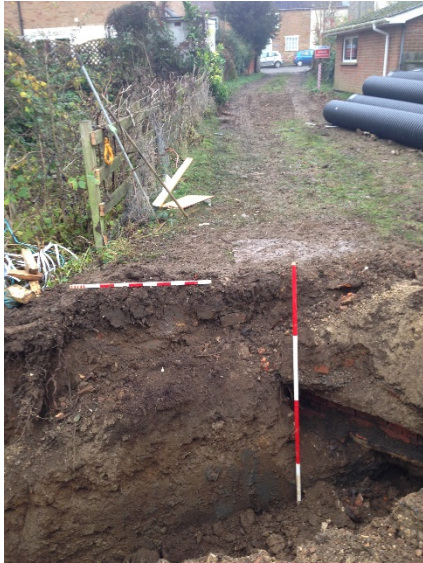
Plate 1. SW-facing section of pipeline trench (Section 6). Scales 1 x 2m; 1 x 1m.
