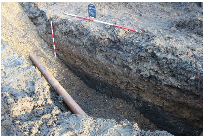
Plate 9. Northwest-facing section of pipeline trench wall (Section 13). Scales 1 x 2m; 1 x 1m.
