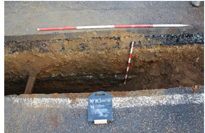
Plate 8. South-facing section of pipeline trench (Section 12). Scales 1 x 2m; 1 x 1m.
