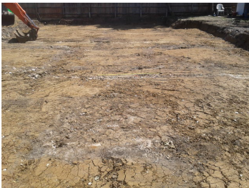
Plate 2: Area A, facing east
