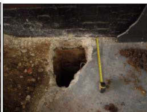
Plate 4: TP4, Looking West
