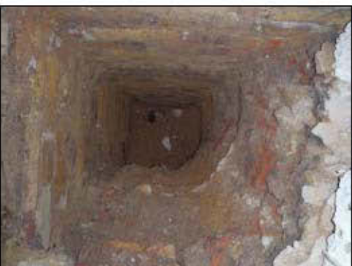
Plate 7: TP7, Looking East
