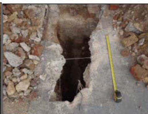
Plate 6: TP6, Looking East
