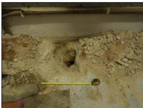
Plate 1: TP1, Looking West
