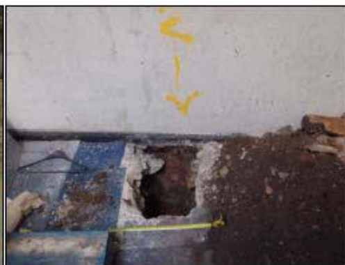
Plate 2: TP2, Looking West
