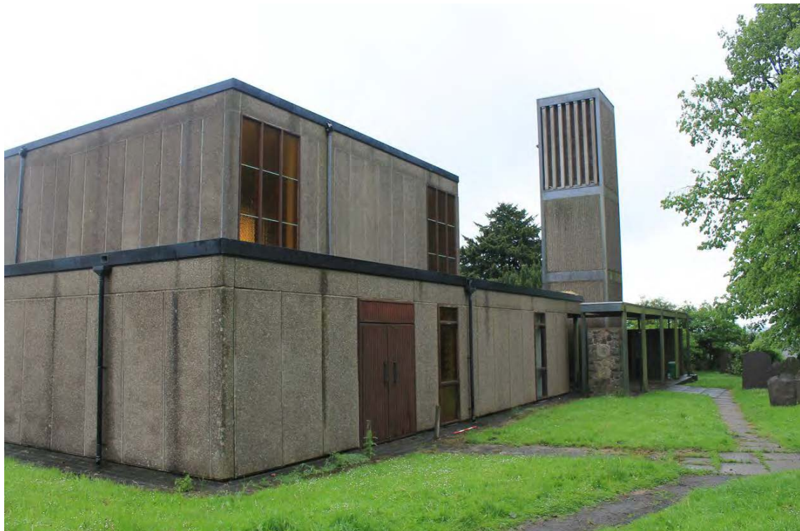
Plate 2: Holy Rood Church pre-demolition. Southern elevation looking NE
