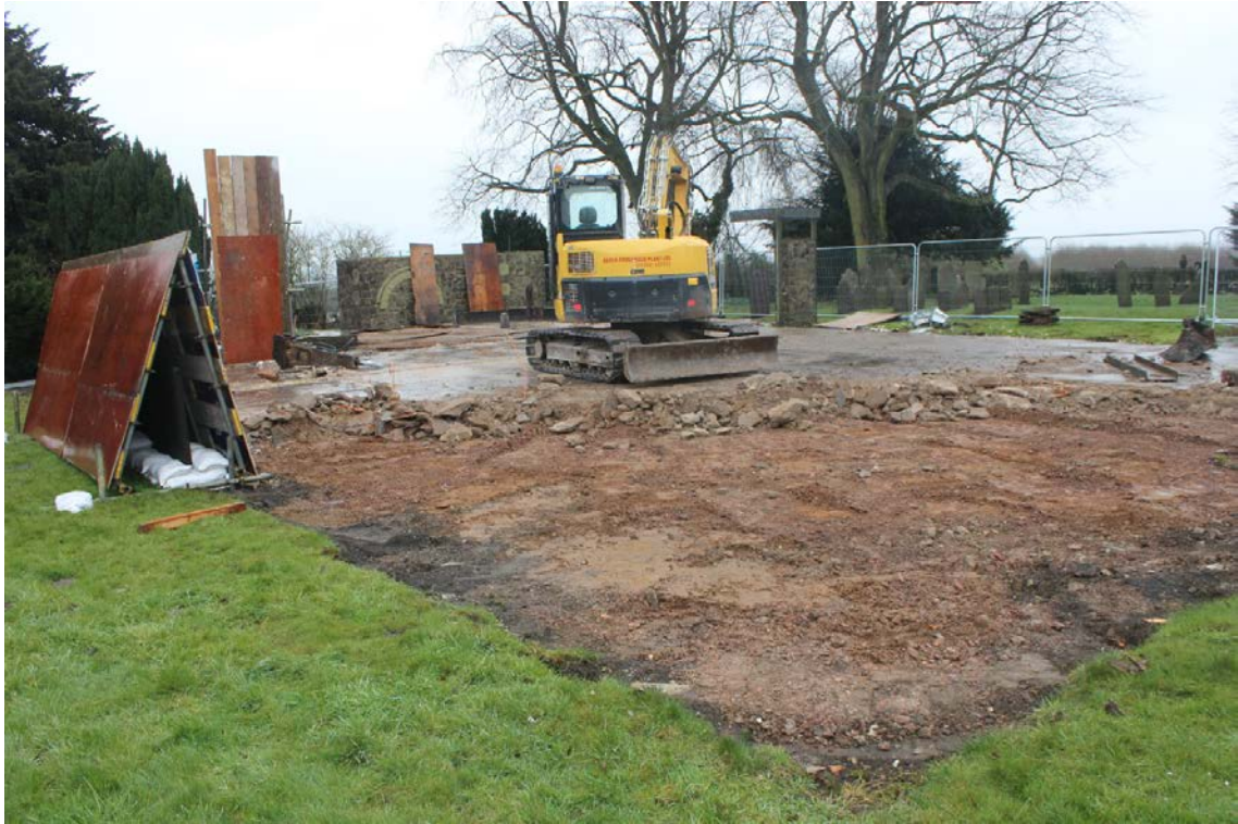
Plate 5: Study Area under demolition. From SE; context 101 exposed.
