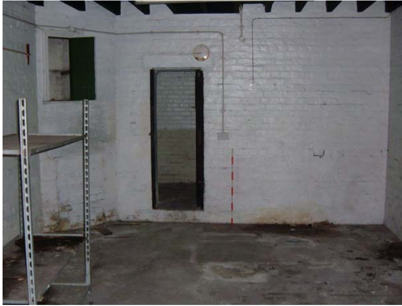
Plate 11. Former Rocket House, interior, north wall, from the south (1m scale).
