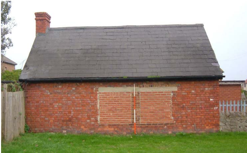
Plate 5. Former Rocket House, exterior, west elevation (2m scale).
