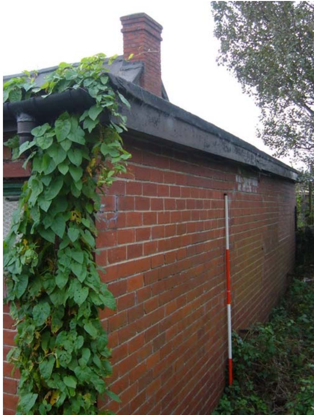
Plate 8. Modern addition to former Rocket House, from the north-east (2m scale).
