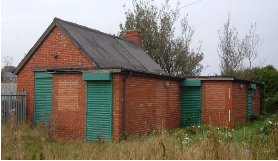
Plate 7. Former Rocket House and modern addition, exterior, from the south-east (2m scale).
