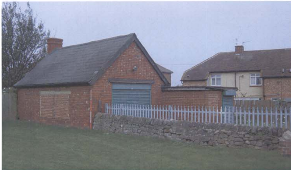
Plate 4. Former Rocket House, exterior, from the south-west ( 2m scale ).
