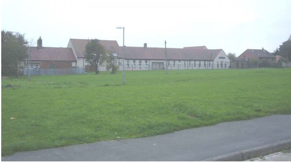
Plate 1. Whitburn C. of E. School, from the north-east.
