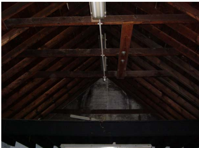
Plate 10. Former Rocket House, interior, roof space, from the south.
