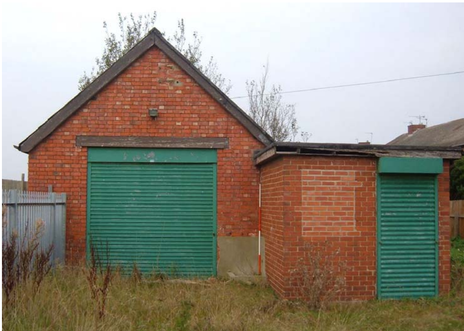
Plate 6. Former Rocket House, exterior, south elevation (2m scale).
