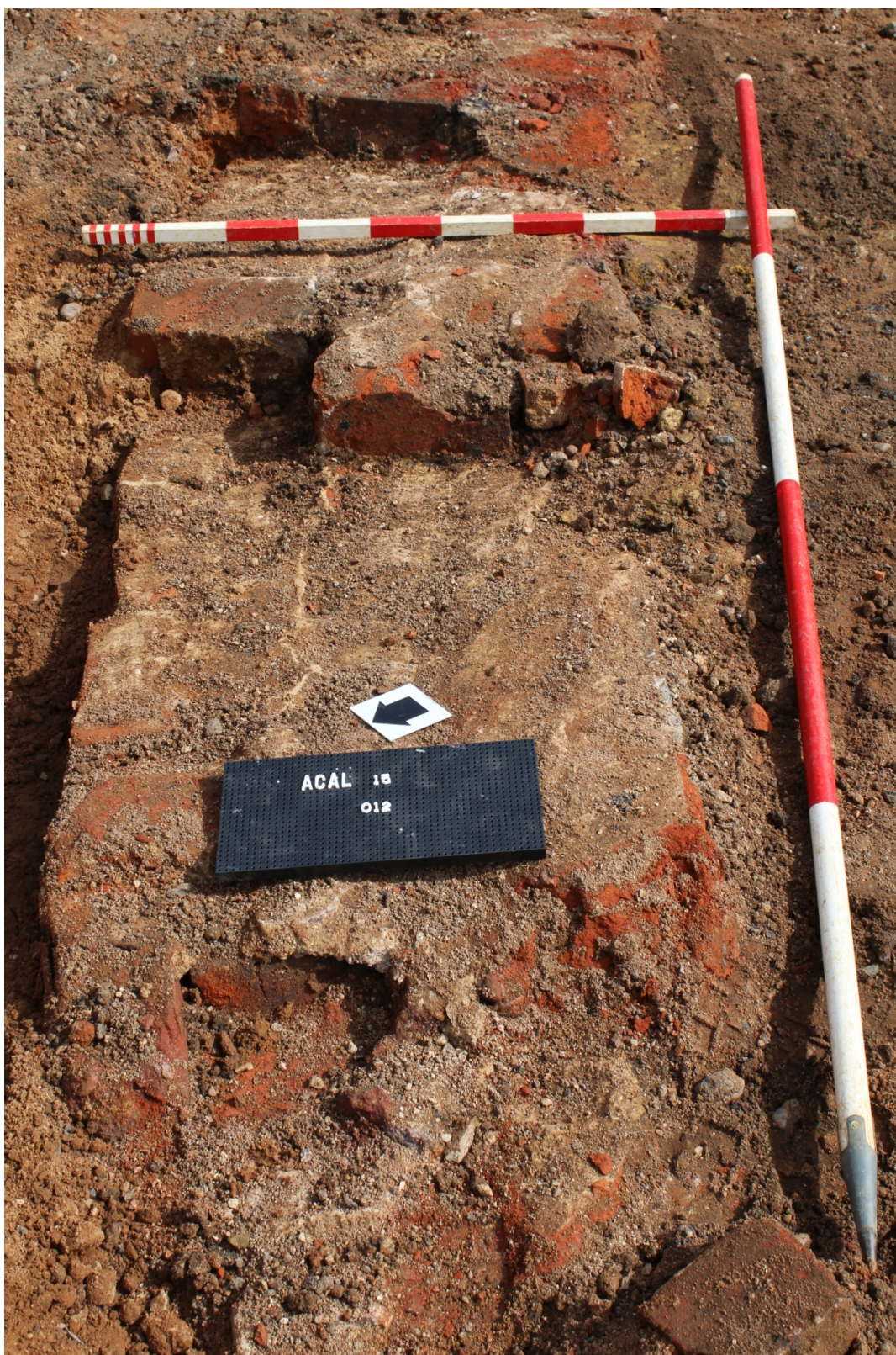
Plate 7: Surviving brick courses of the southern wall foundation (012) to Bridge 62, looking E
