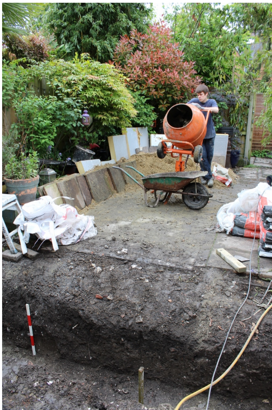
Plate 2: D9, View to South of foundation trench. Scale 0.5m
