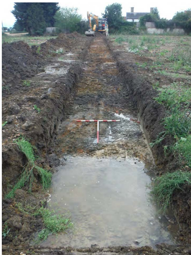
Plate 11: Trench 8, West facing view of trench
