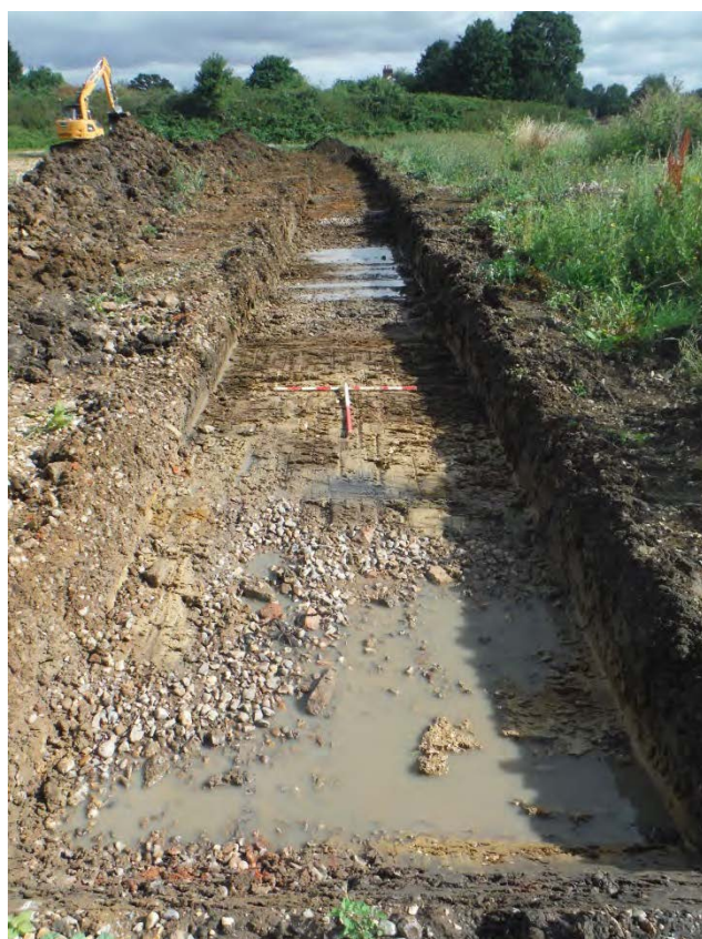
Plate 14: Trench 4, North facing view of trench
