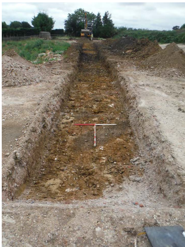
Plate 17: Trench 3, South-west facing view of trench
