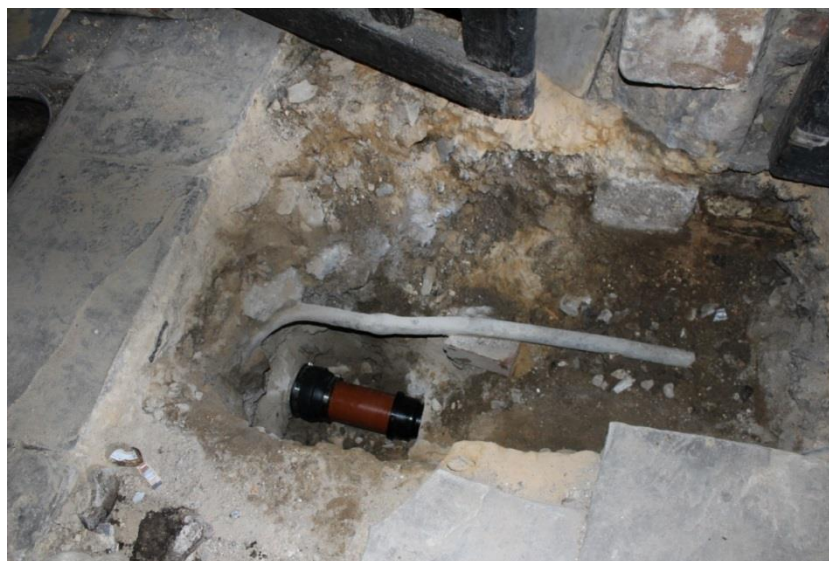
Plate 3: Pipe repair and medieval masonry [1] and [2] looking west
