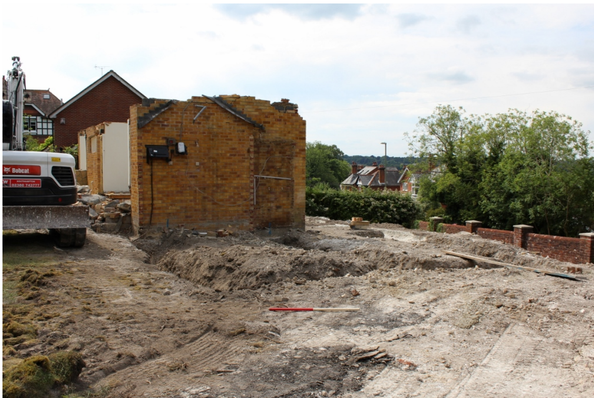
Plate 3: D6 View to west showing new foundation trenches at east end of existing house. Scale 1m
