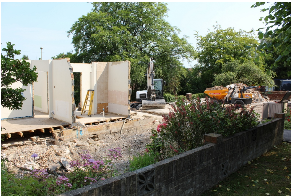
Plate 1: D12 General view of site from Baring Road looking north-east.
