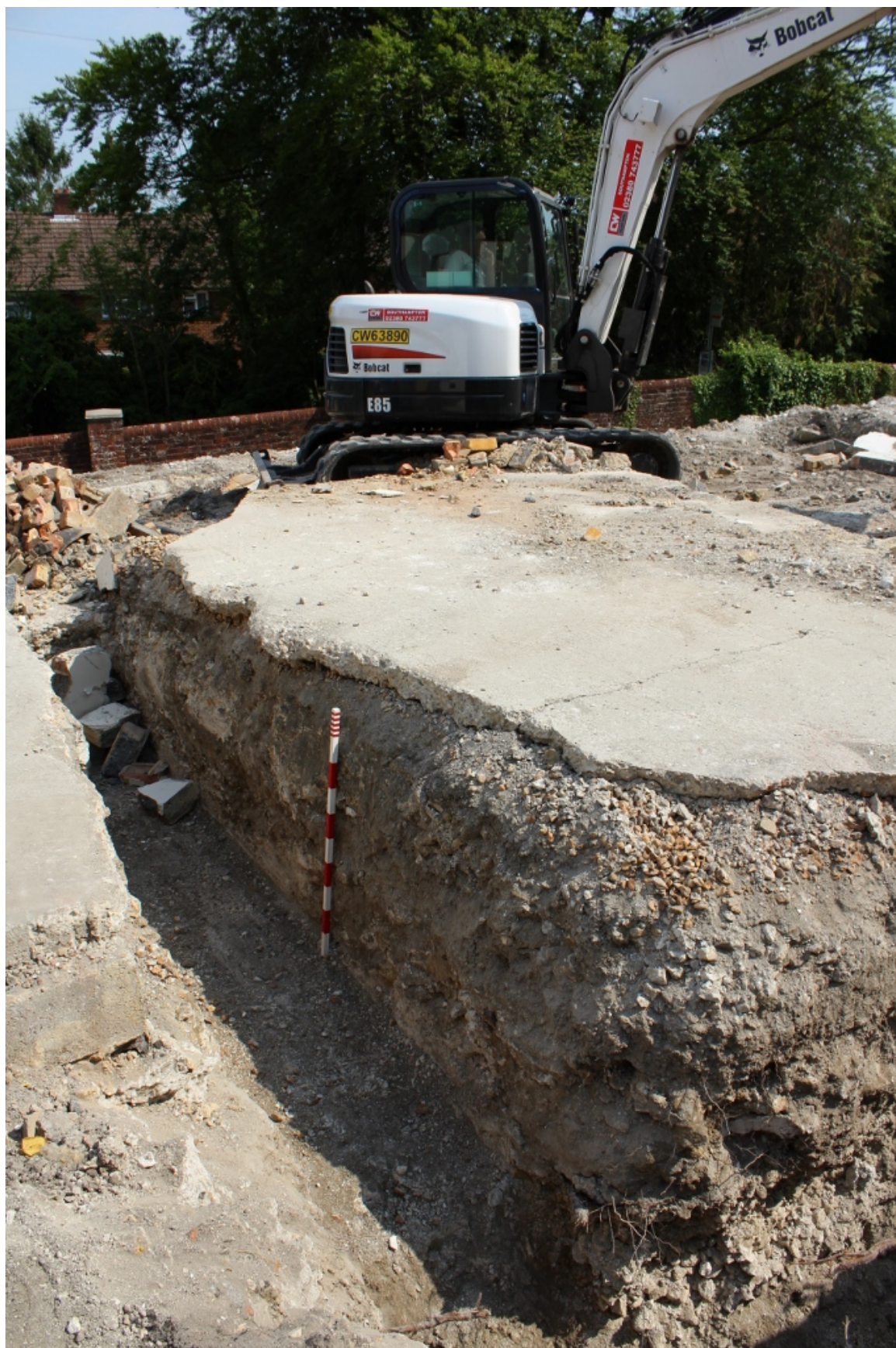
Plate 6: D9 View north-east showing new foundation trench for extension to east and soil and chalk rubble fill overlying natural chalk. Scale 1m.
