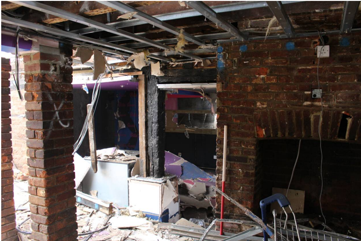
Plate 34 South-eastern storey post of original building
