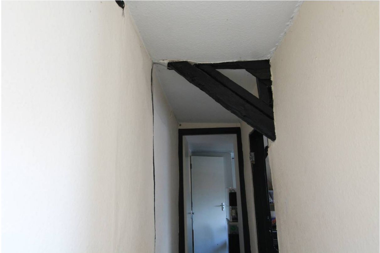
Plate 28 Common rafter of catslide seen in (FF6)
