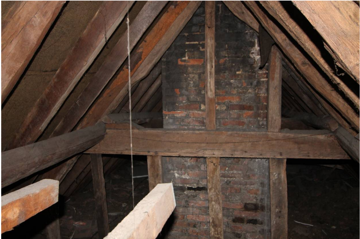
Plate 24 Framed former gable end and later overlain purlins
