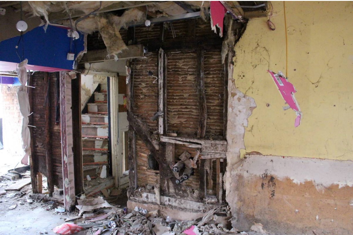
Plate 36 Wall framing and noggin to outshut
