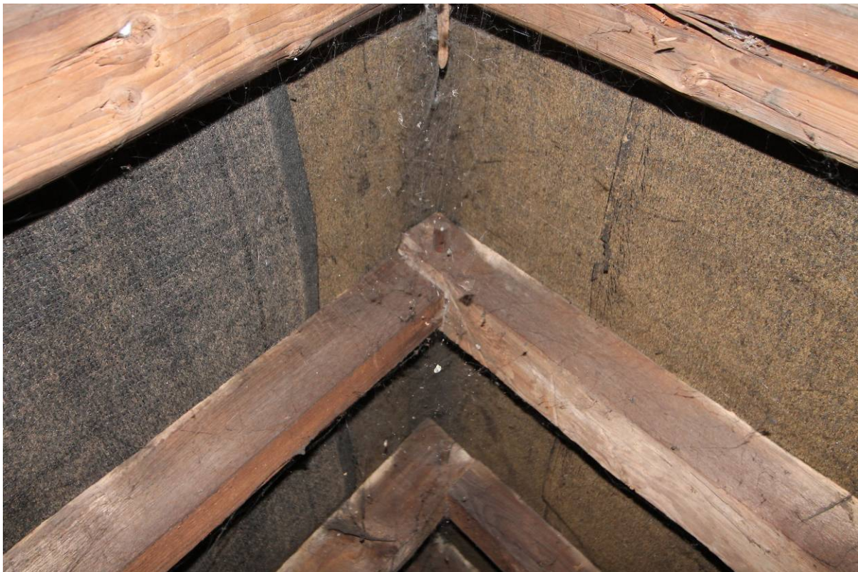
Plate 25 Halved and pegged common rafters at ridge
