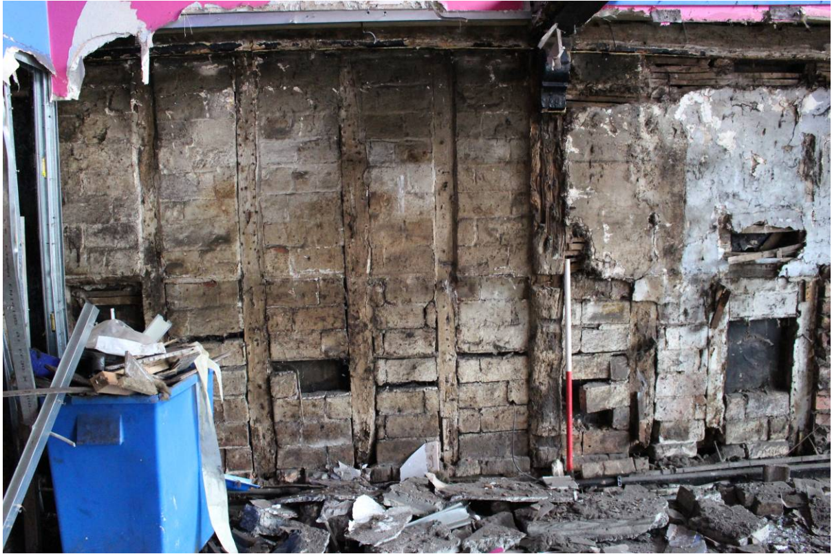
Plate 30 Timber-framing and storey post in south-western end wall of building (A)
