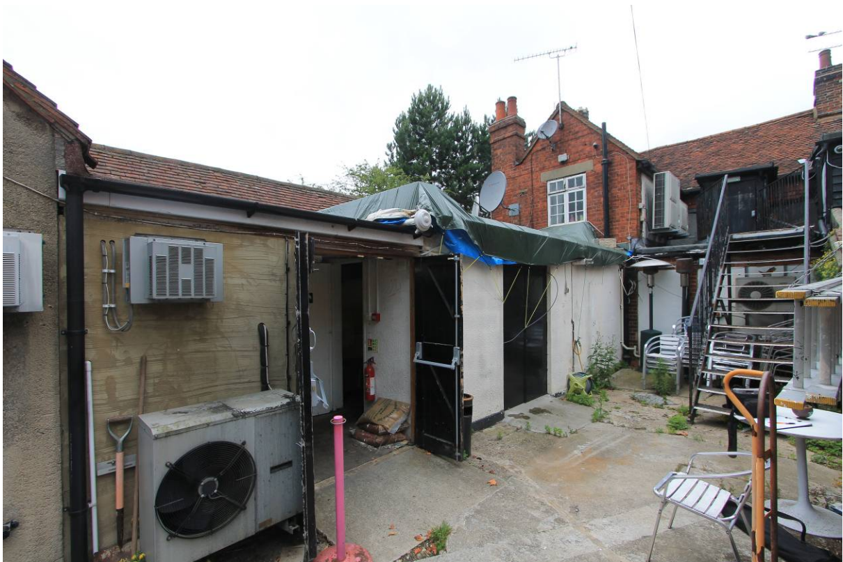
Plate 6 Rear elevations showing modern flat roofed extensions (F) and brick, 2 storey gabled addition
