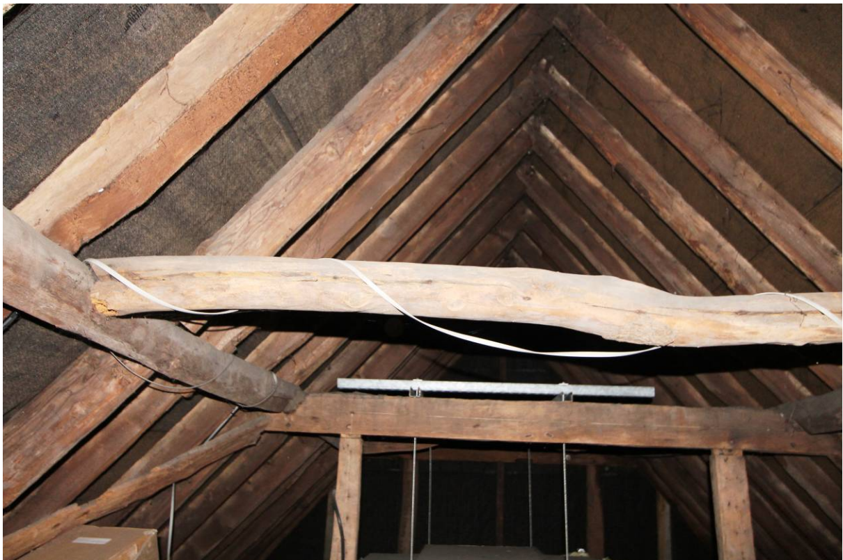
Plate 23 Clapsed side purlin roof (older roof) showing intermediate collar, looking south-west
