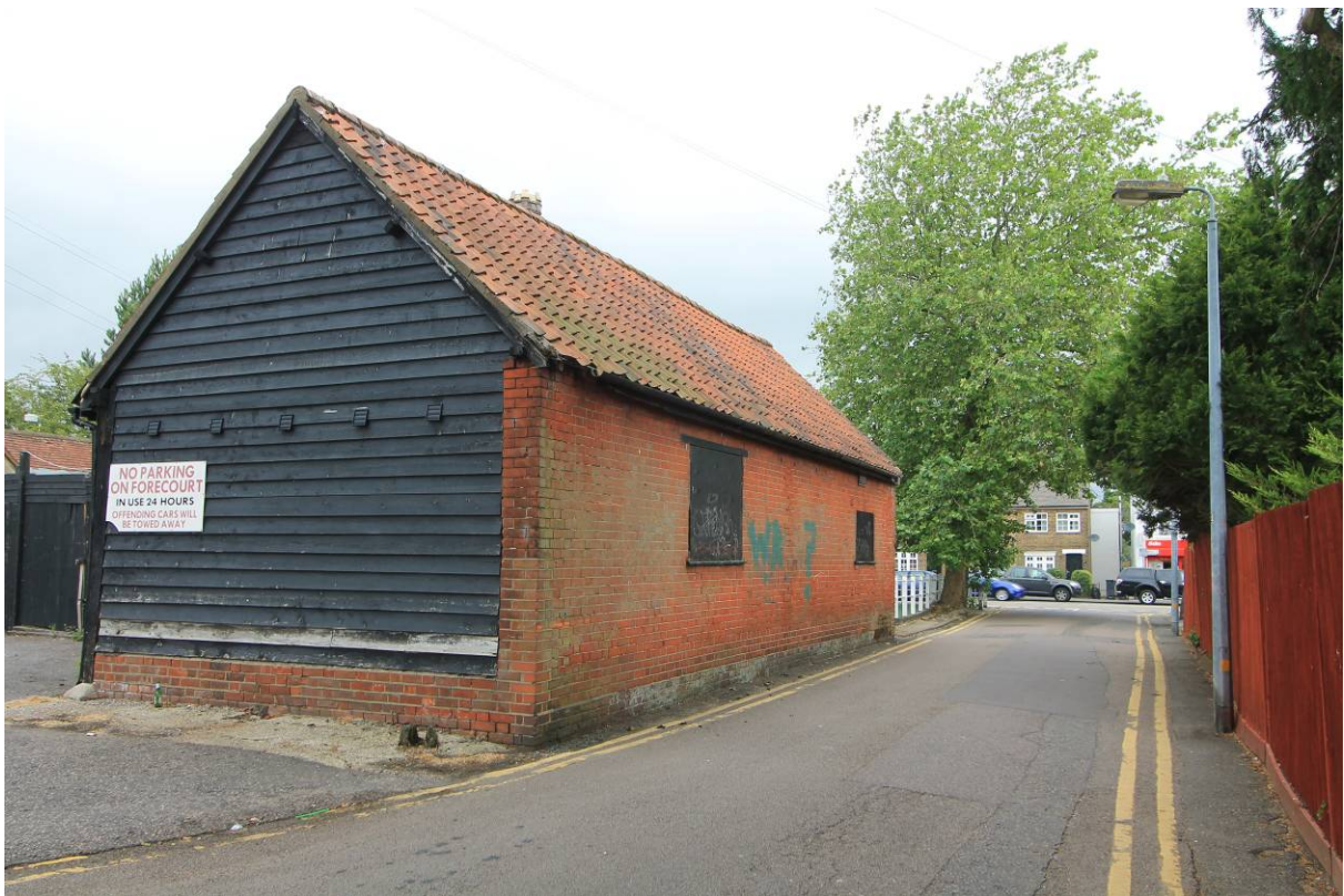
Plate 4 Former stable building (B) looking north-west
