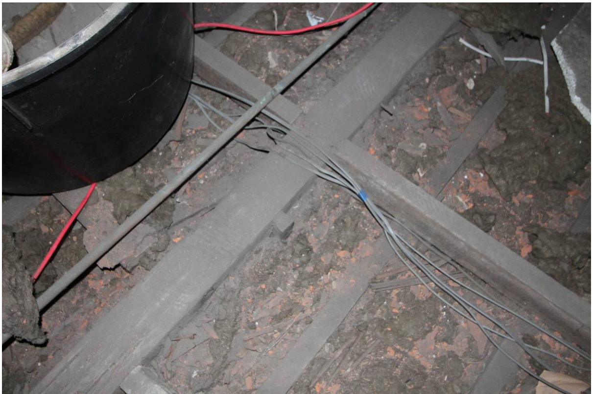
Plate 27 19 th century soft wood ceiling structure
