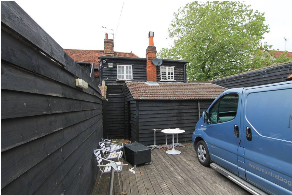
Plate 5 Rear elevations showing lean-to (D) and first floor extension, looking north-west
