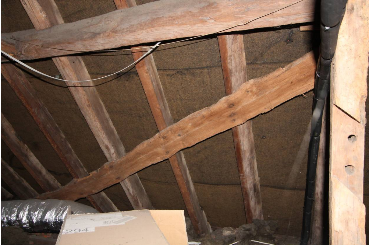
Plate 26 Plank like wind brace nailed to rafters
