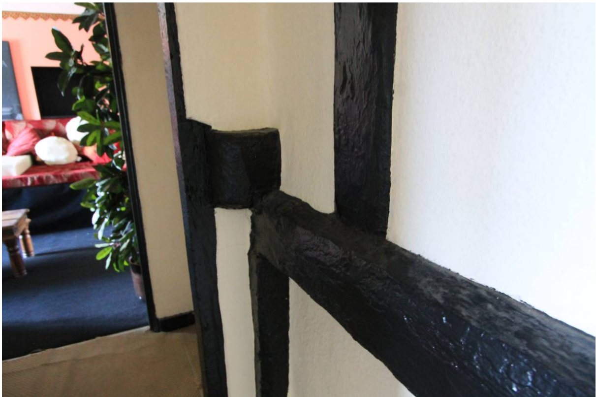
Plate 21 Wall framing to passage (FF5) and cut rail, looking north-east
