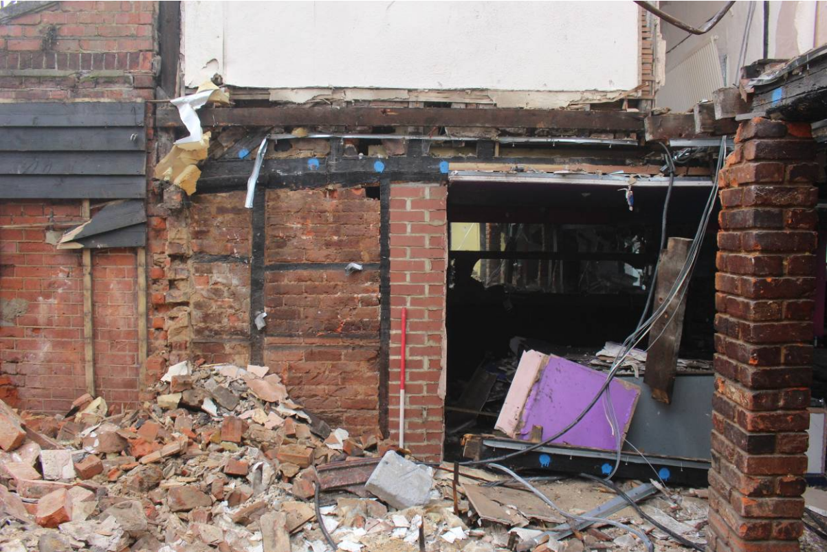
Plate 36 Wall framing and noggin to outshut
