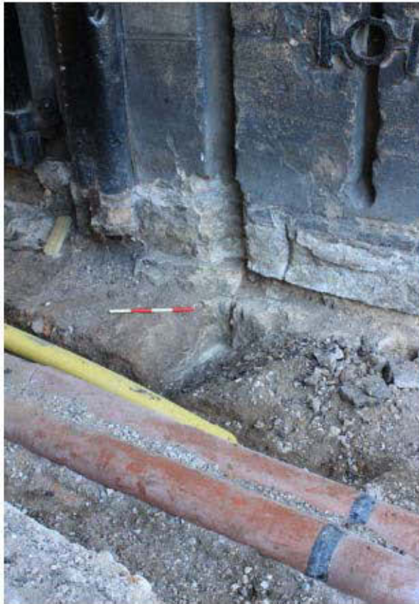
Plate 5: Eastern edge [8] of drawbridge pit [8/27/65] under outer port cullis slot, looking south east, 0.4m scale
