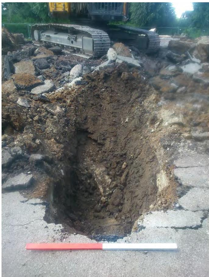
Plate 3: Made ground and alluvium revealed whilst removing concrete pads
