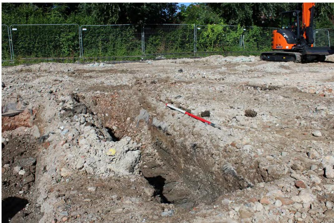
Plate 5: The narrow trench located centrally to the development plot exposing made ground overlying an organic-rich alluvium, looking northwest
