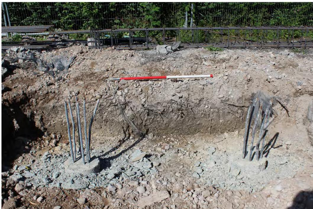
Plate 4: The new foundation pits exposing recently backfilled made ground, the concrete pads and piles, looking west.
